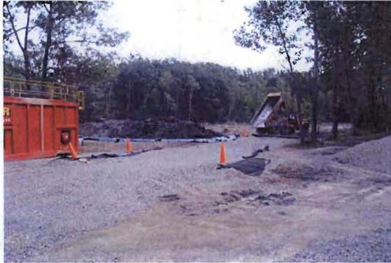
**Soil from hot spot locations are staged in lined staging area**
