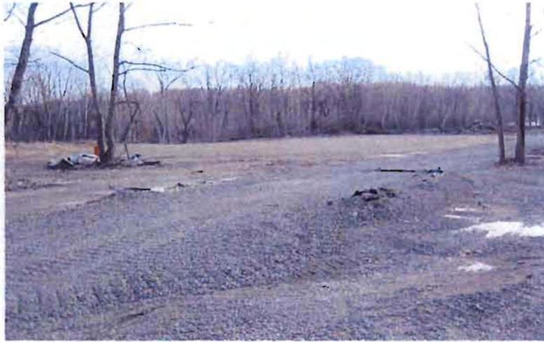
**Area 1 after backfilling and compaction**
