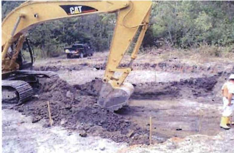
**SB-E4 being excavated, top 18 inches removed prior to removing to 4'**
