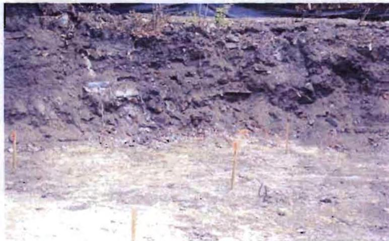
**SB-20 sidewall showing brick and debris**
