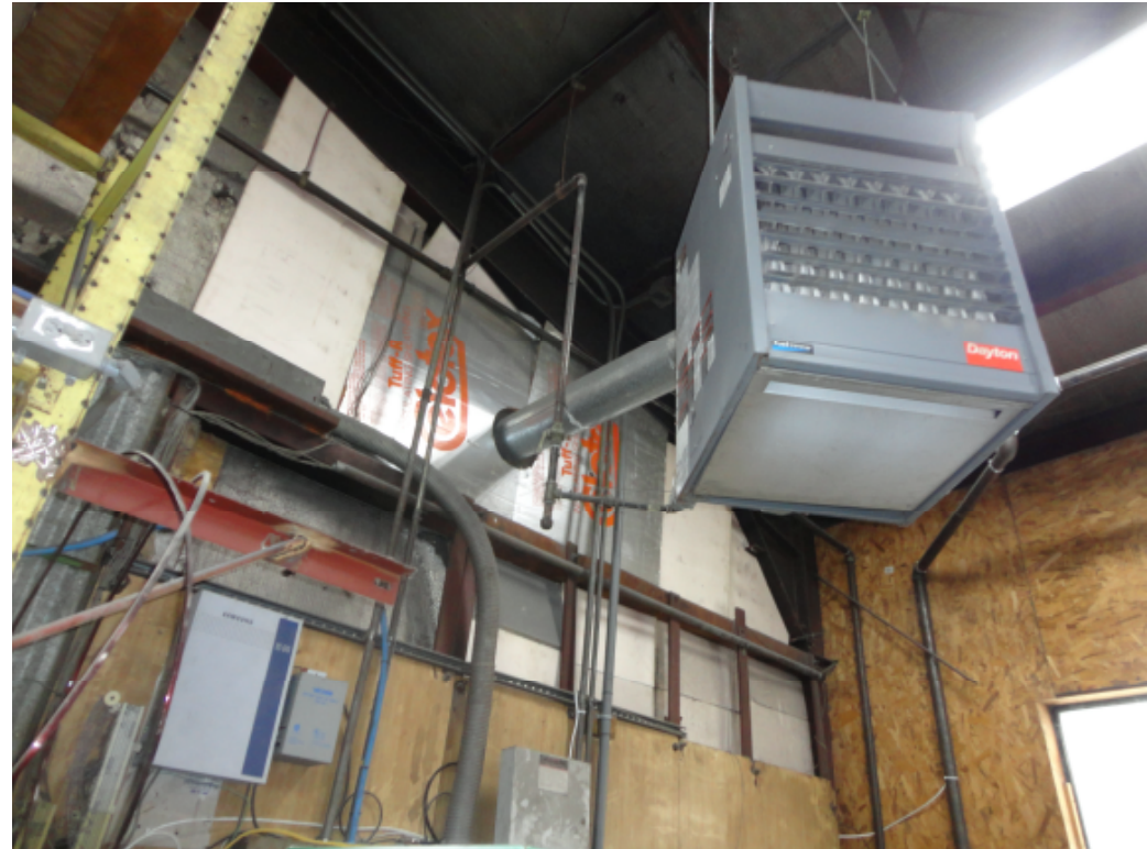
22 Ceiling mounted heater in eastern site building.JPG
