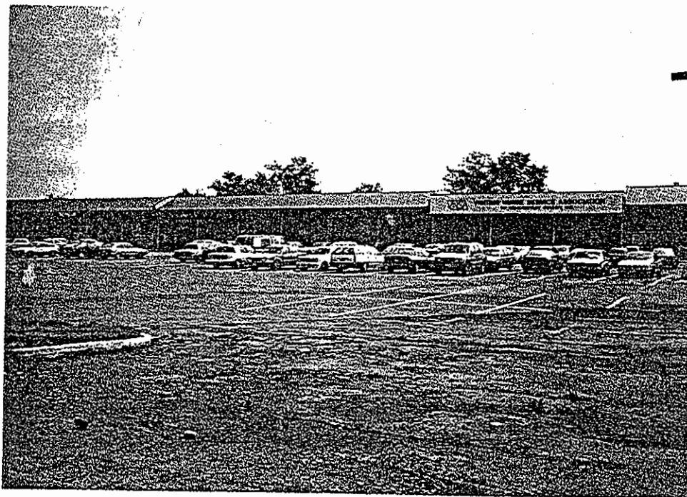
(2) Looking Northeast at Subject Site from Southwest Corner.
