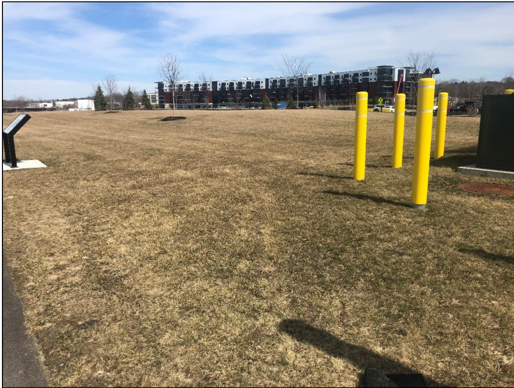
Photo 3. Parcel A – April 3, 2019 Cover Inspection
