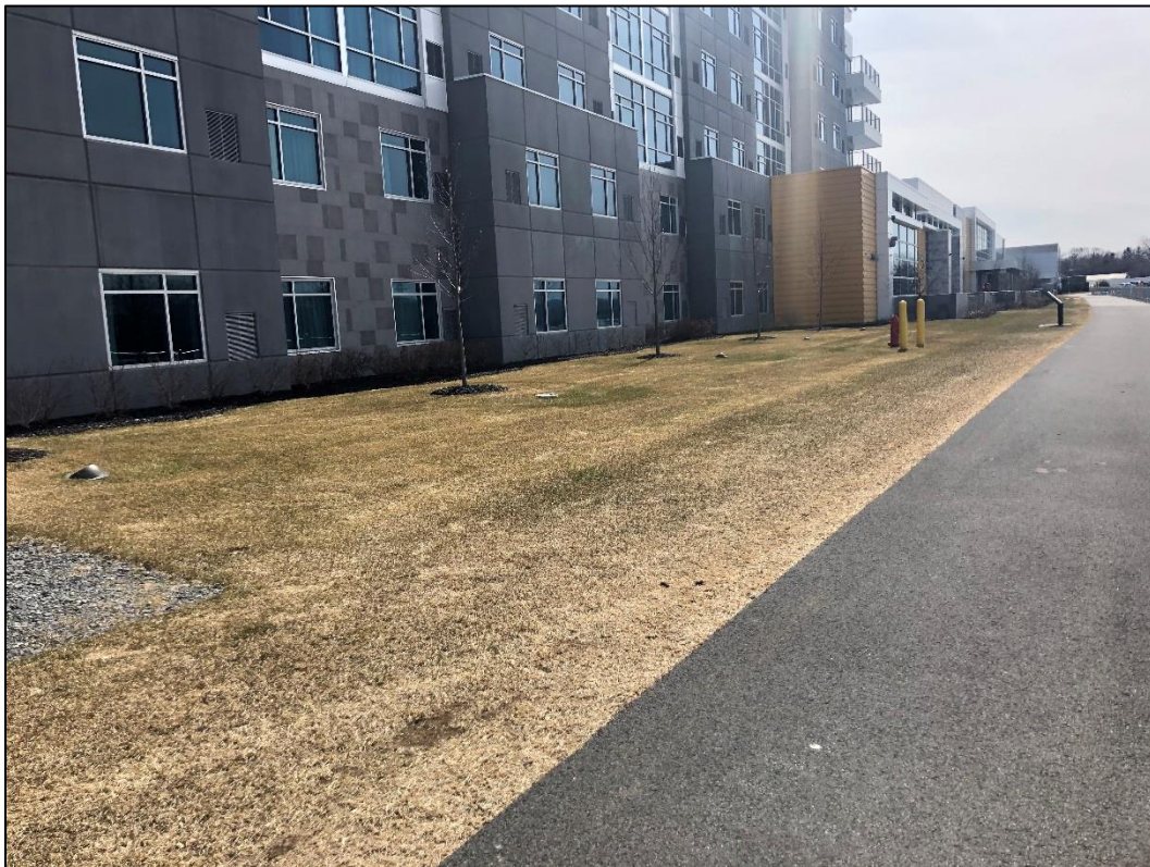
Photo 2. Parcel A – April 3, 2019 Cover Inspection
