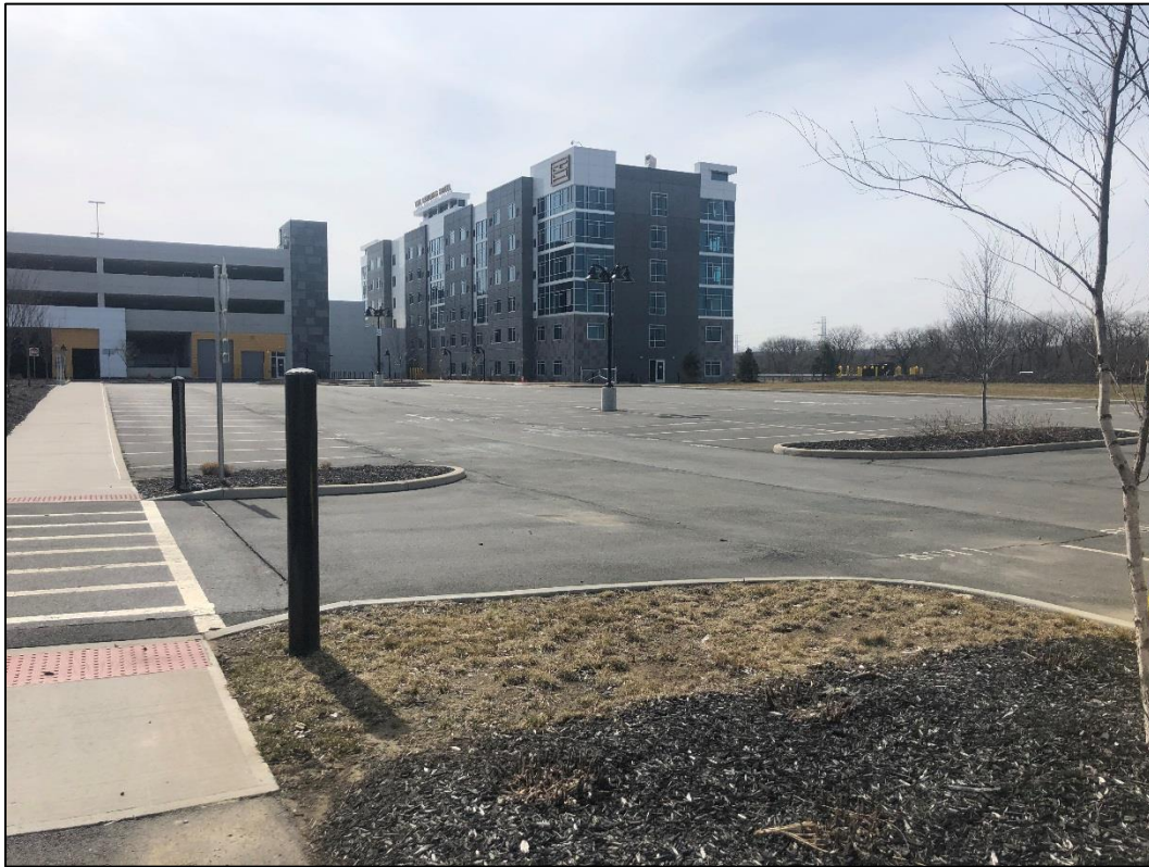
Photo 7. Parcel A – April 3, 2019 Cover Inspection
