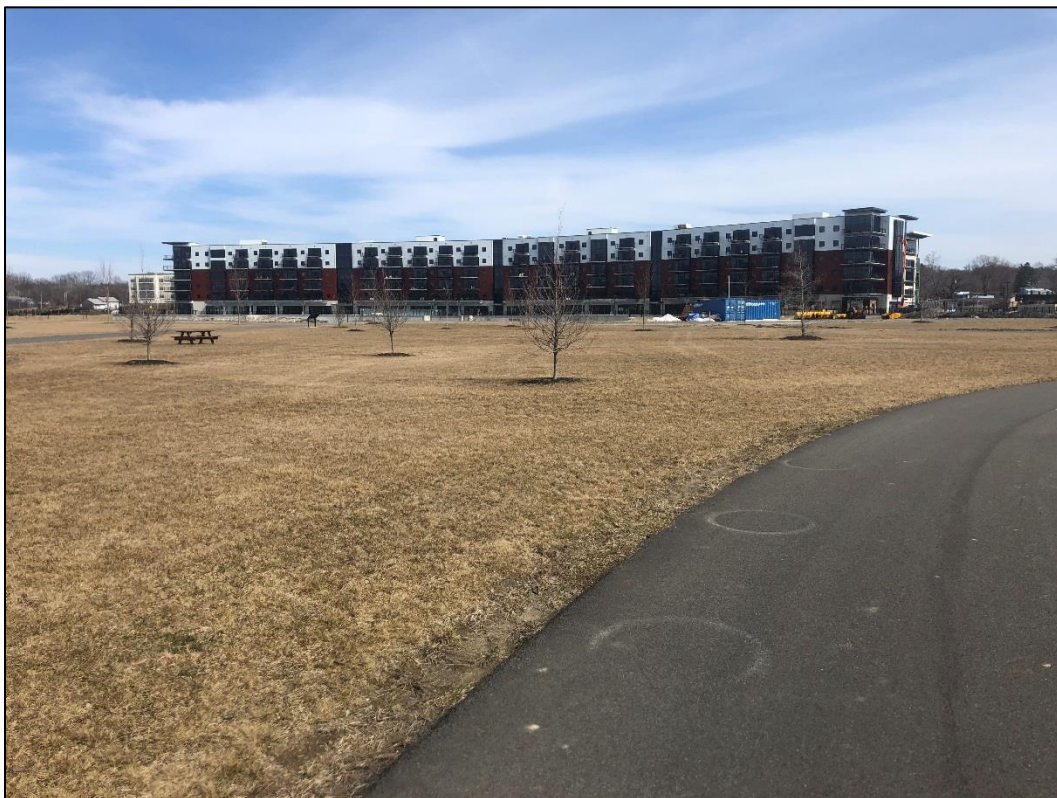
Photo 6. Parcel A – April 3, 2019 Cover Inspection
