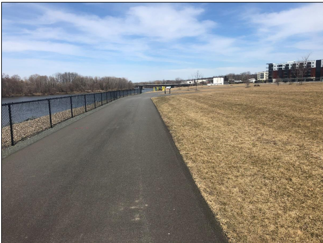
Photo 4. Parcel A – Parcel A – April 3, 2019 Cover Inspection
