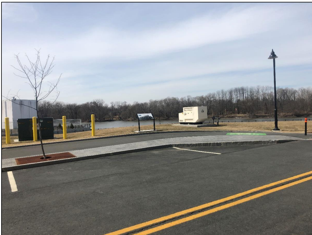
Photo 4. Parcel B – April 3, 2019 Cover Inspection.
