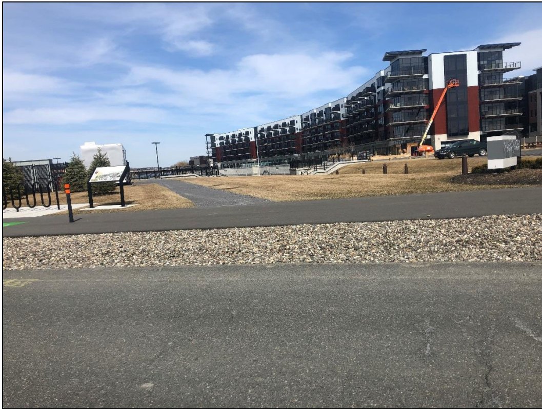
Photo 1. Parcel B – April 3, 2019 Cover Inspection.
