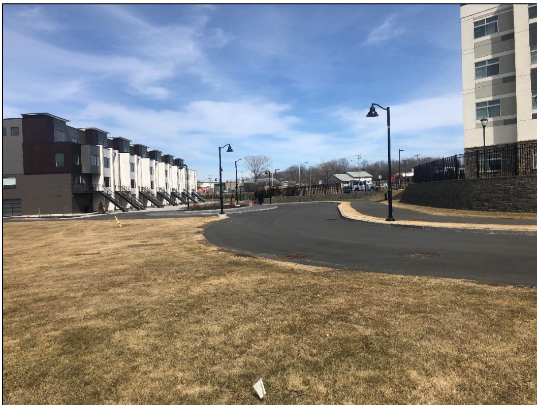
Photo 8. Parcel B – April 3, 2019 Cover Inspection.
