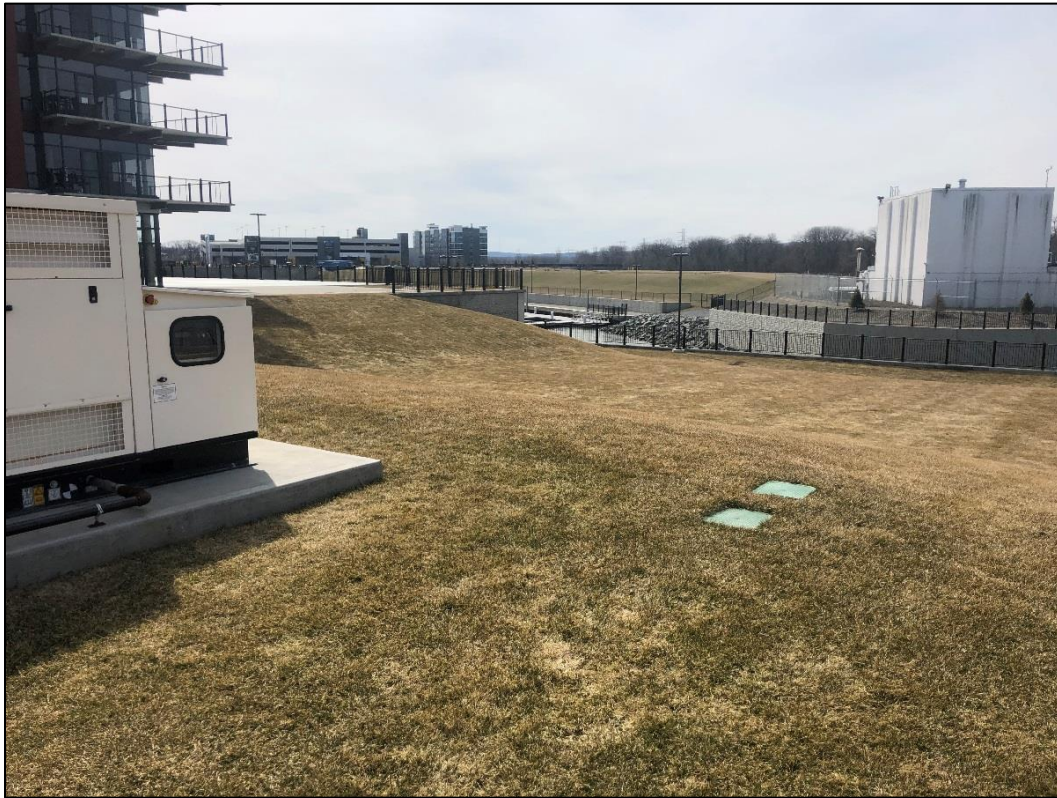
Photo 5. Parcel B – April 3, 2019 Cover Inspection.
