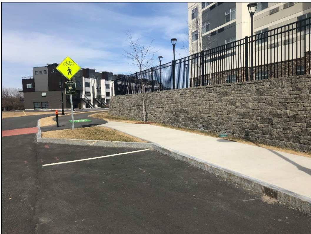
Photo 2. Parcel B – April 3, 2019 Cover Inspection.
