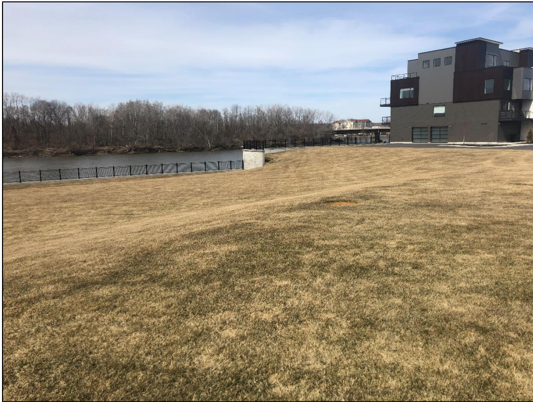
Photo 7. Parcel B – April 3, 2019 Cover Inspection.
