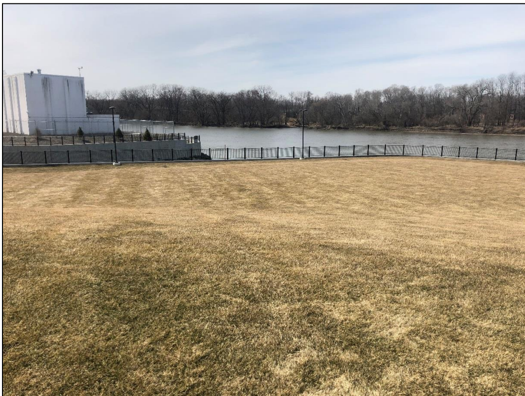
Photo 6. Parcel B – April 3, 2019 Cover Inspection.
