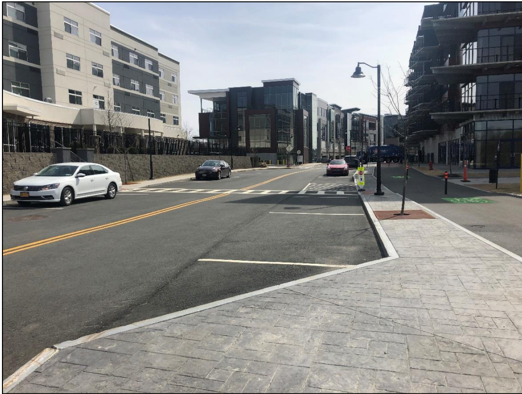
Photo 9. Parcel B – April 3, 2019 Cover Inspection.
