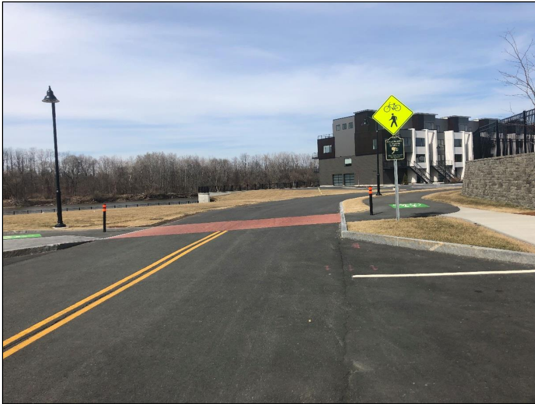
Photo 3. Parcel B – April 3, 2019 Cover Inspection.
