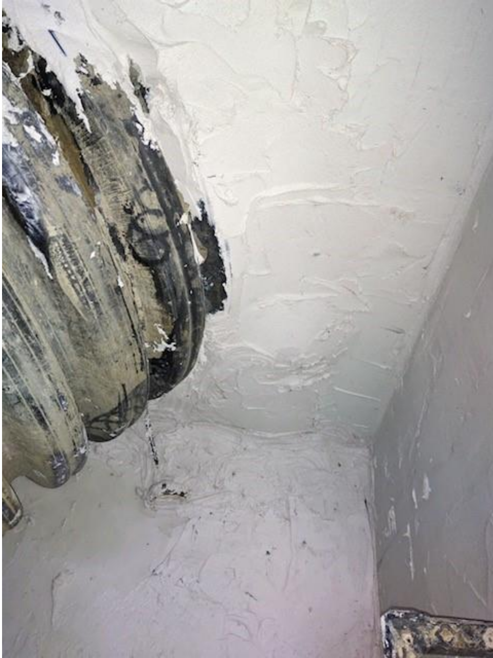
Figure 1: Epoxy seal (inlet pipe connection)
