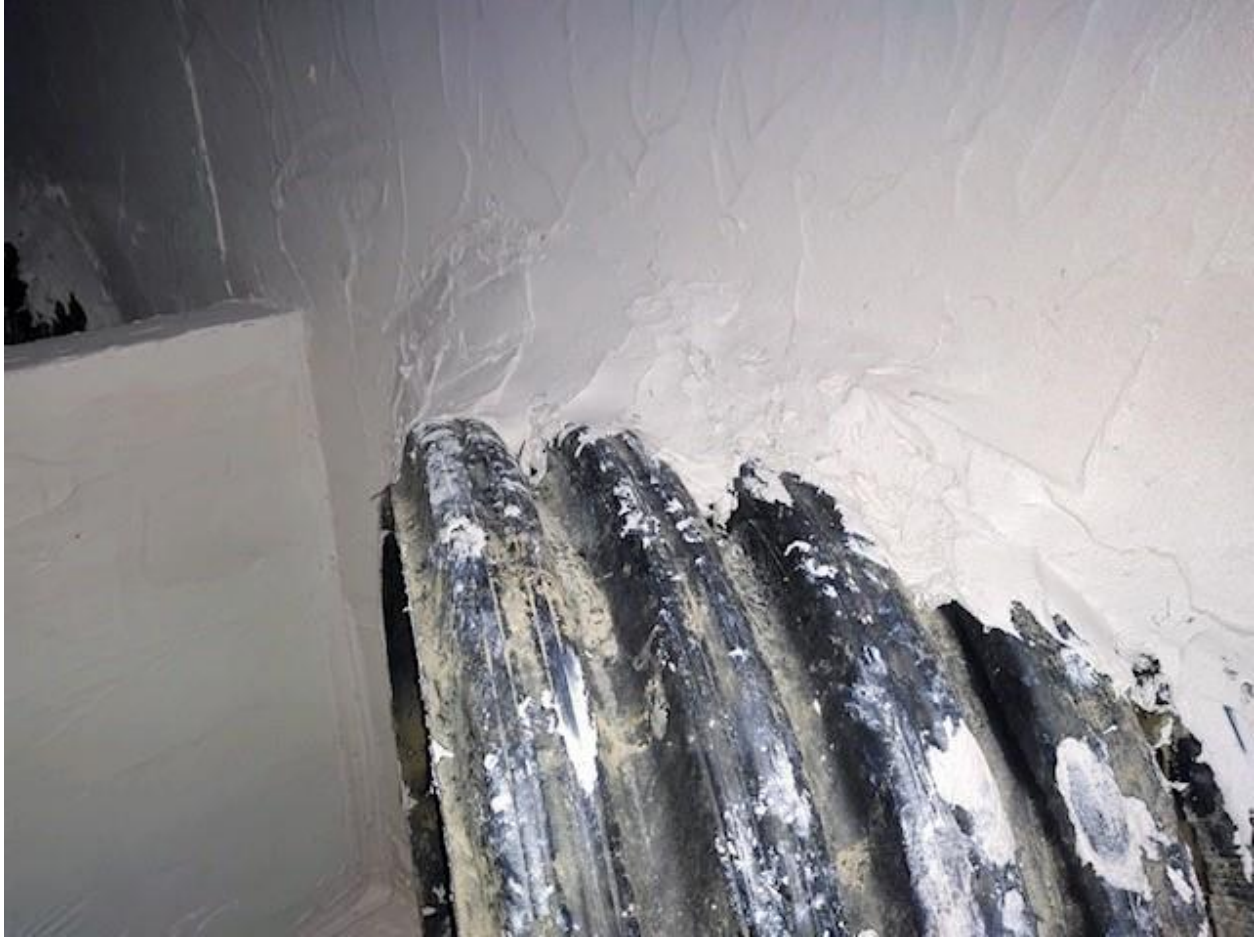
Figure 4: Epoxy Seal (outlet pipe connection)
