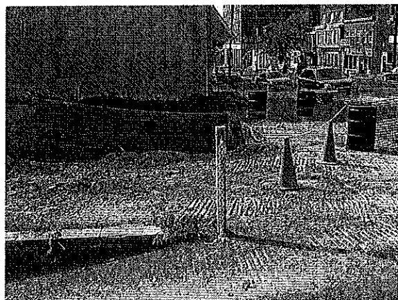
Excavation Area 3 facing west
