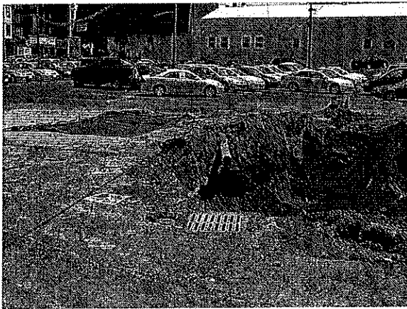
Northern edge of excavation
