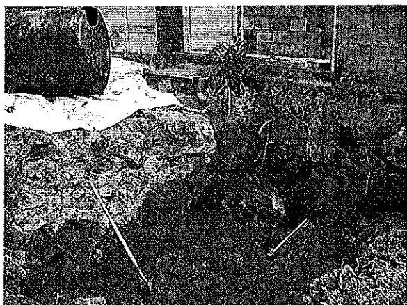
Excavation after UST-3 removal
