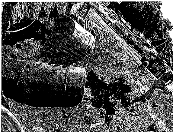
UST-4 Being removed from excavation
