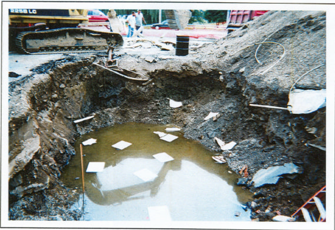
Photograph 2: View to the southwest of the kerosene UST pit
