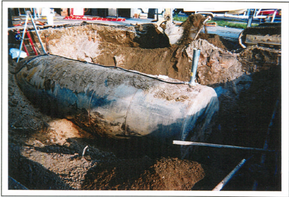
Photograph 7: View to the southeast of the central gasoline UST
