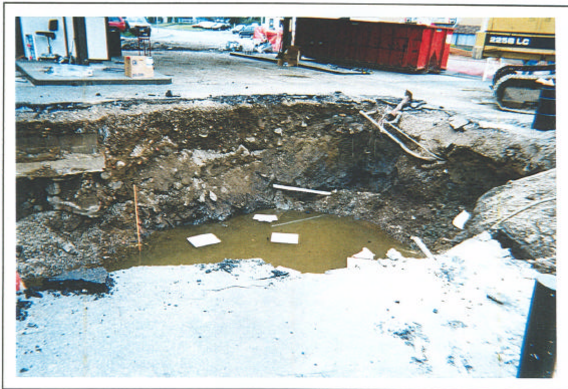
Photograph 3: View to the south of the kerosene UST pit
