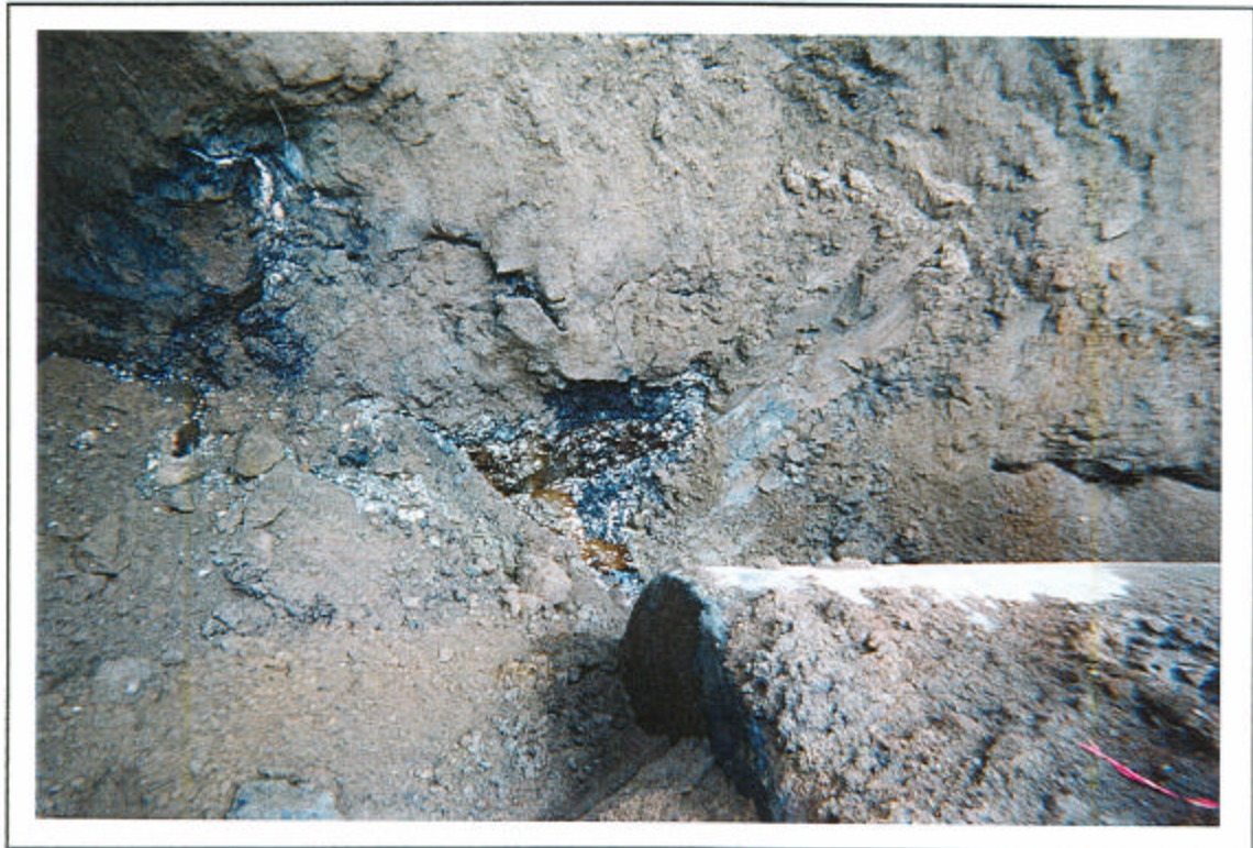
Photograph 9: View of northwest corner of southern tank pit
