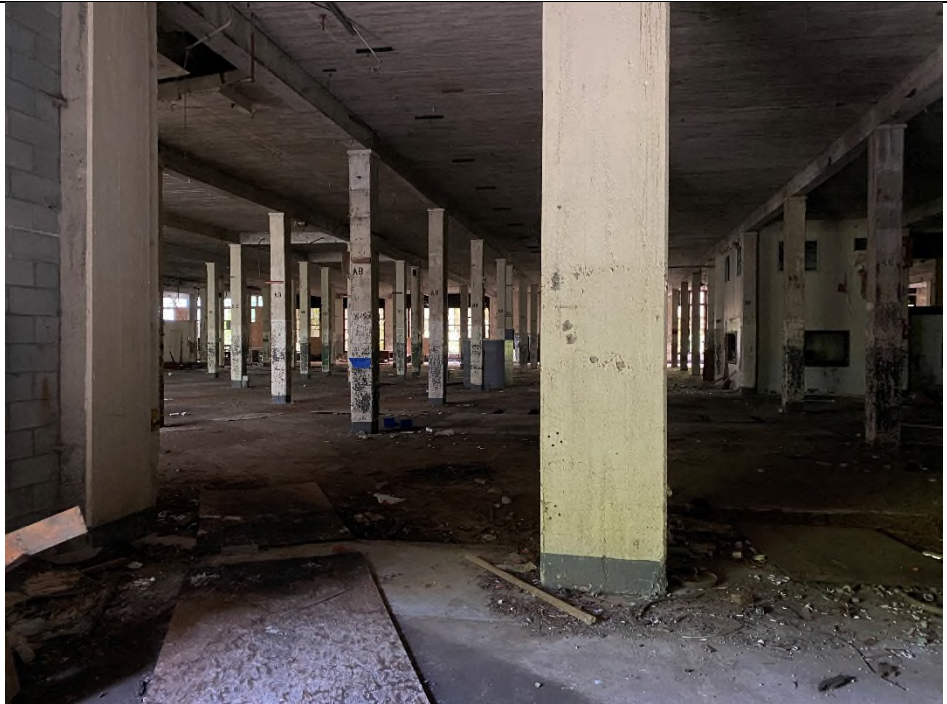
Photo 6 – Typical interior view of main structure.
