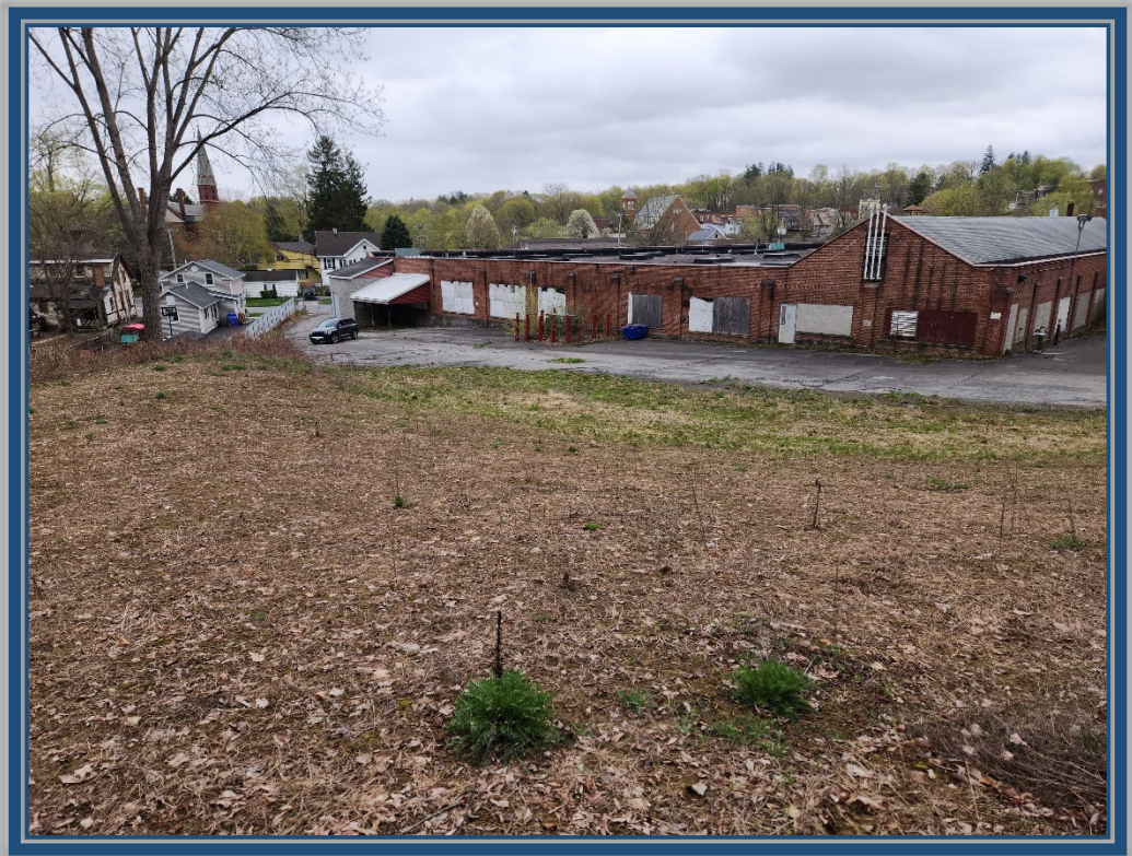
Soil cover system & asphalt/gravel surfaces; southeast view from northwest corner of Site
