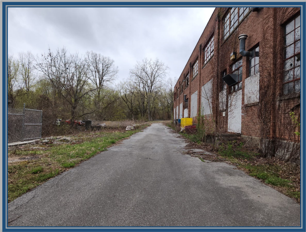
Asphalt & concrete cover system located adjacent to the building & Gordon Creek
