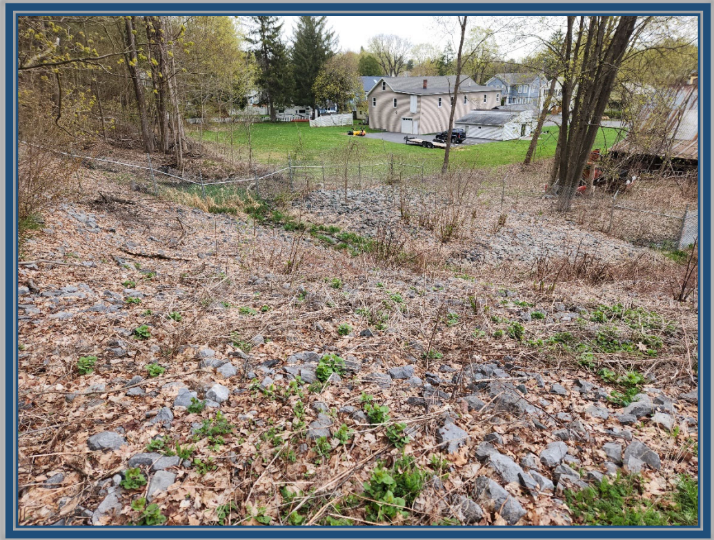
Rip/Rap cover system at northwest corner of the site; facing northeast
