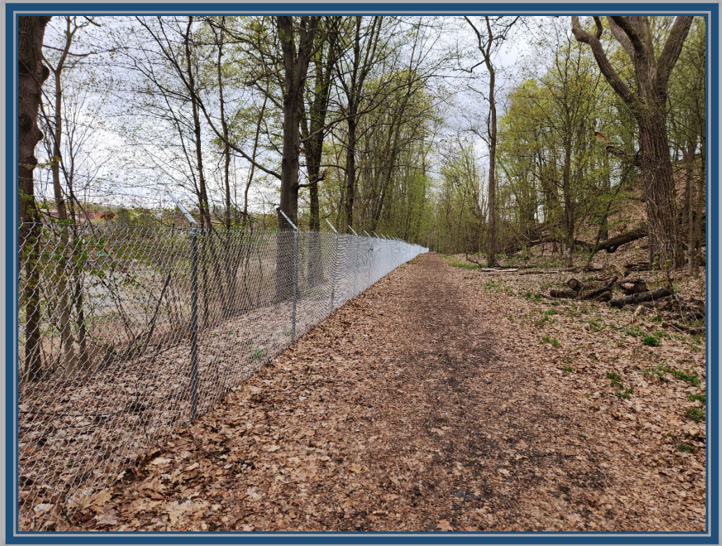
Site perimeter security fencing along western property line; facing south from Jim Tedisco Fitness Trail
