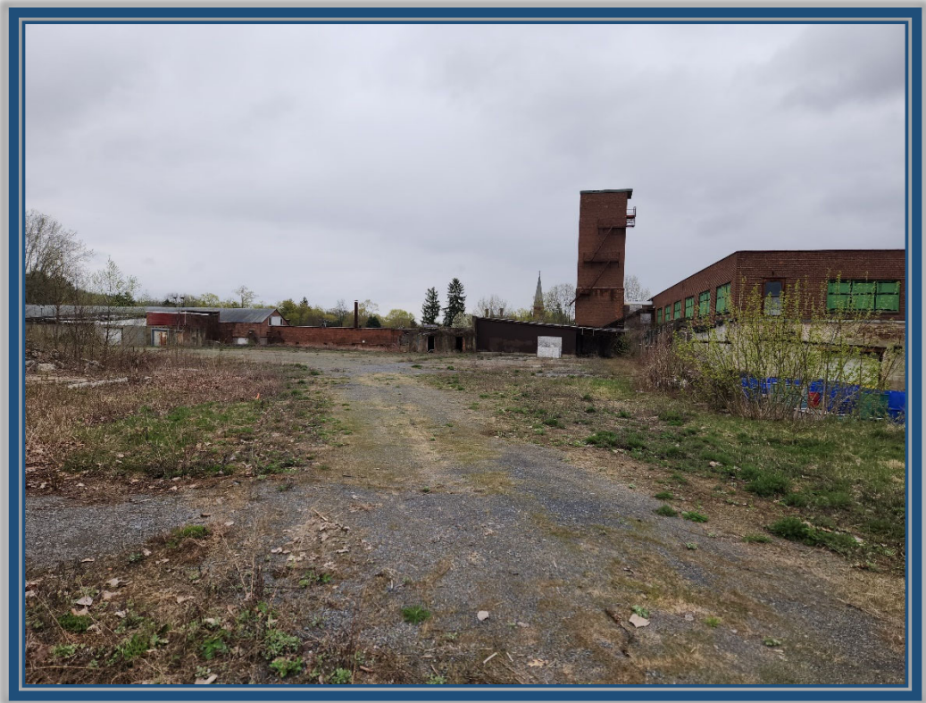
Improved gravel cover system west of building; facing east from soil / Rip Rap cover systems
