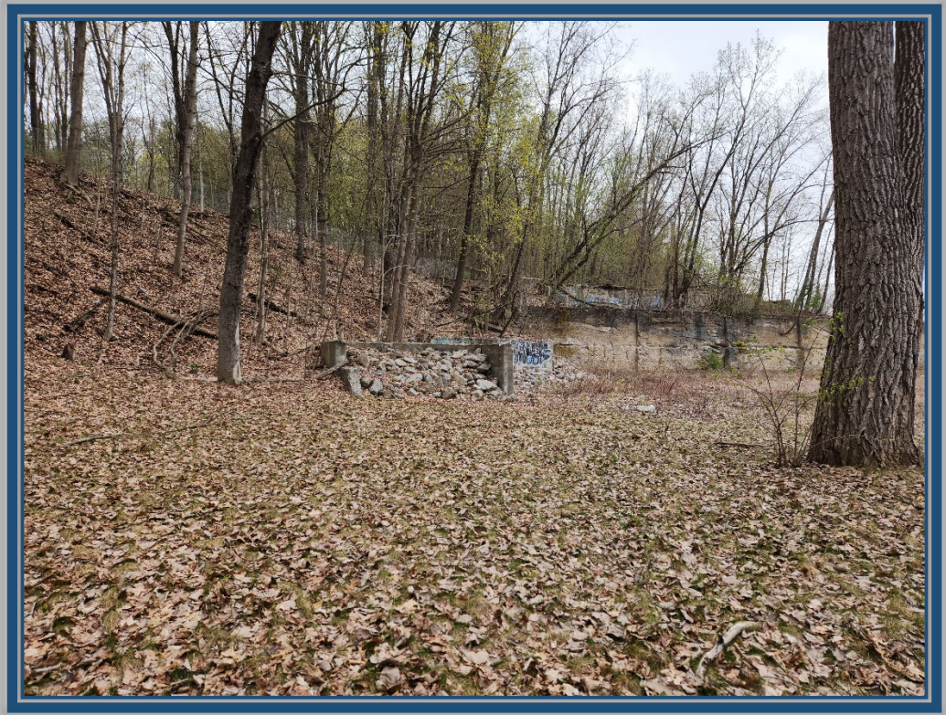
Western extent of soil / Rip Rap cover systems & building foundations north of Gordon Creek
