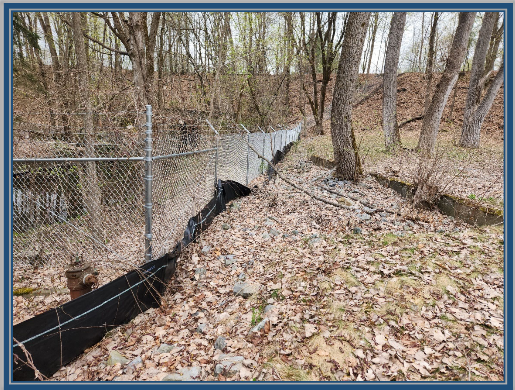
Soil cover system north of Gordon Creek; southwest corner of the Site
