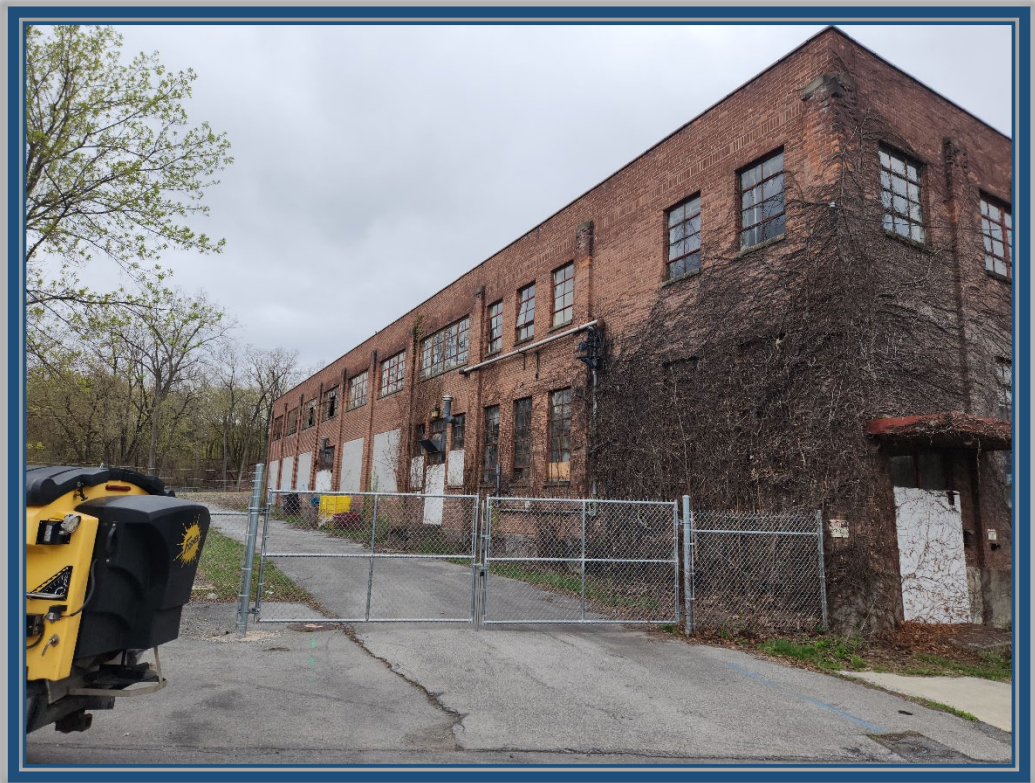
Southeast gated entrance to site facing northwest from Bath Street
