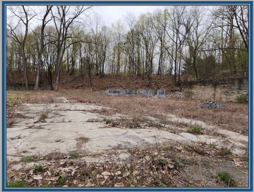
Soil cover system & concrete foundations facing northwest from Gordon Creek
