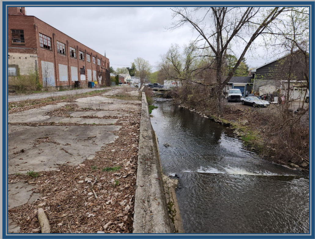
View of southern property line & concrete retaining wall along Gordon Creek
