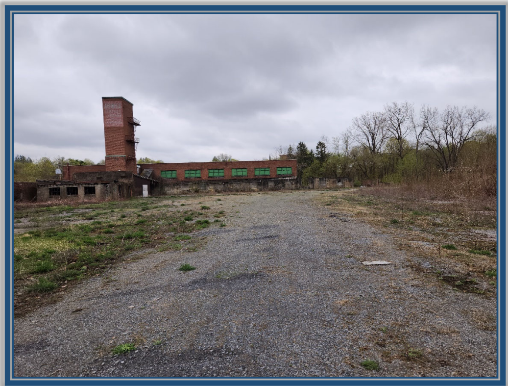
Improved gravel cover system & building foundations west of building; facing south
