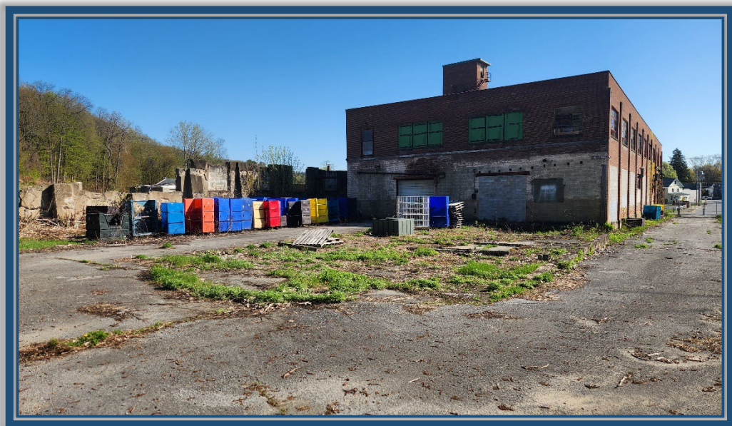
Asphalt & gravel cover systems adjacent to soil cover system southwest of building
