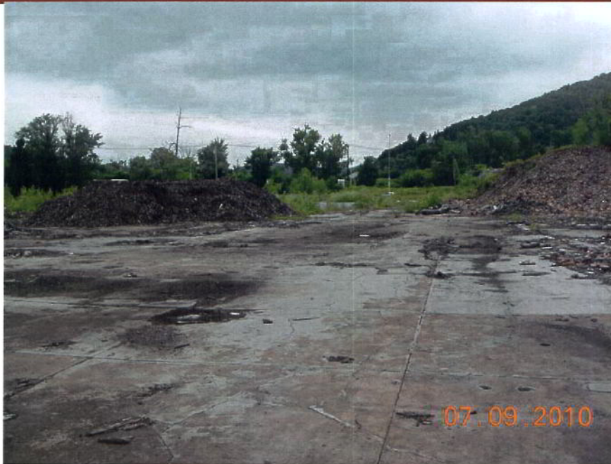
View north of remainder of building foundation observed to be stained from an oil based product.
