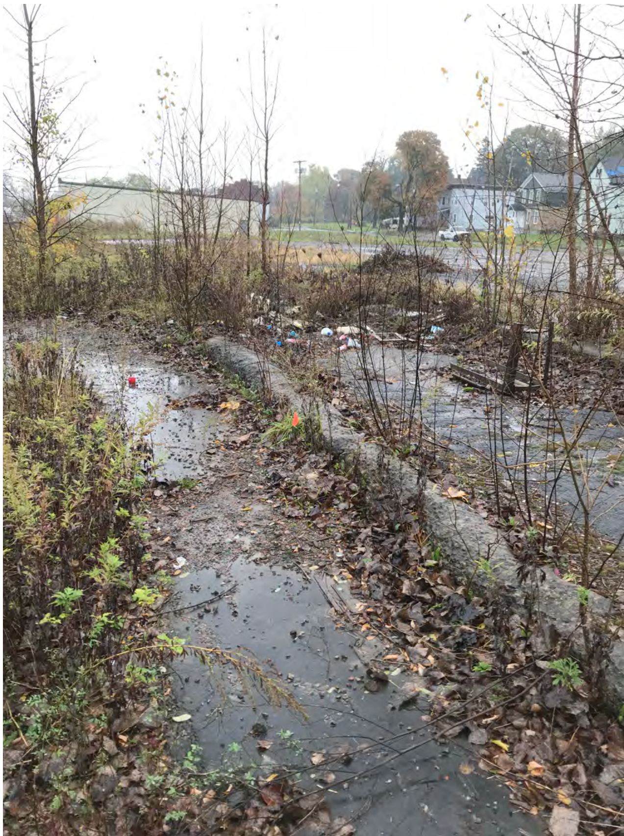
Photo 4 - Concrete slab in eastern-central (upper) portion of Site
