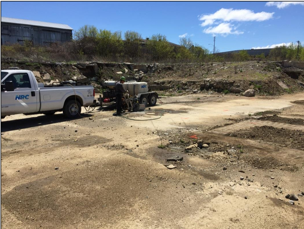
Saw cutting limits of concrete demolition
