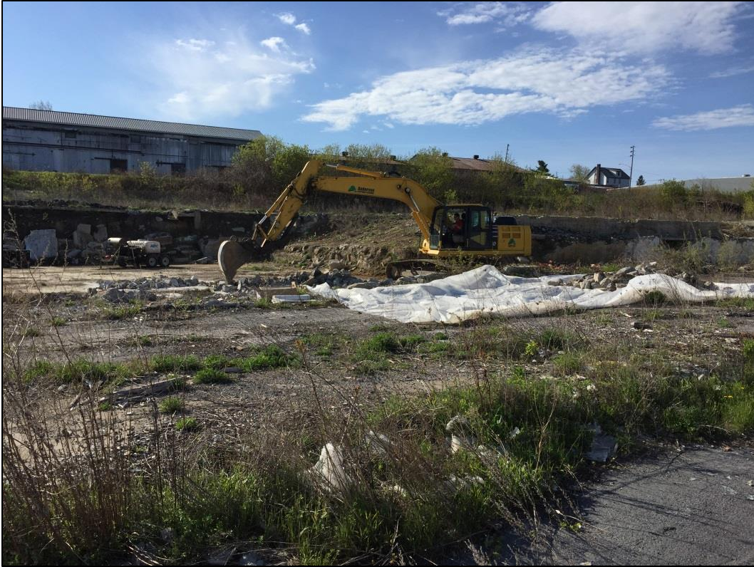
Rubblized concrete staged on 12-mil poly.
