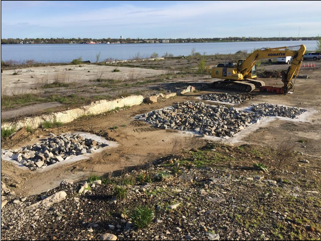
Concrete surface slab demolition.
