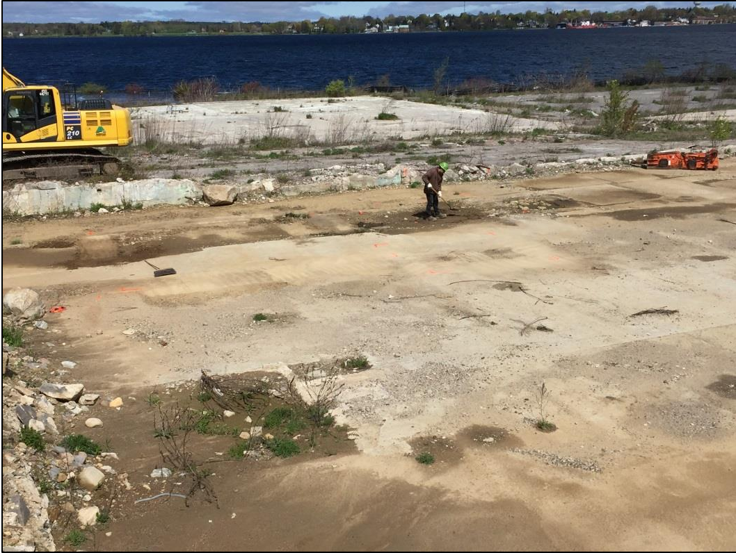
Excavation limits delineation (orange paint).
