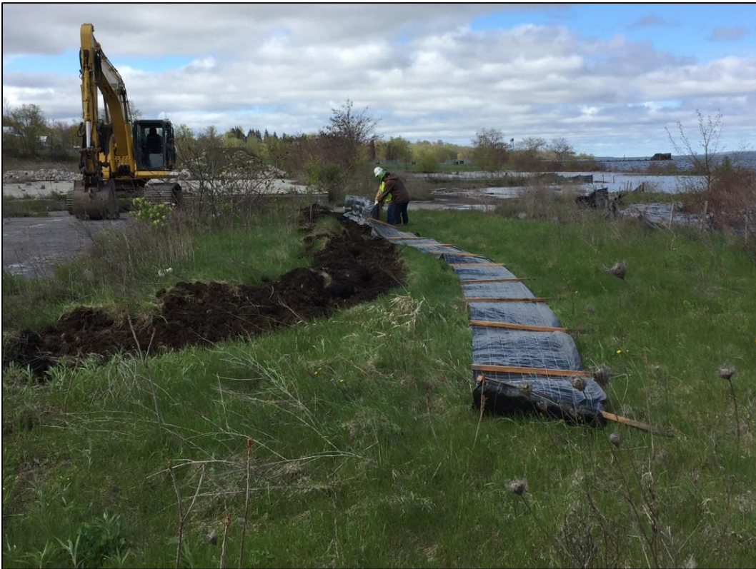
Silt fence installation
