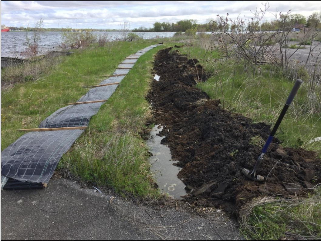
Silt fence installation
