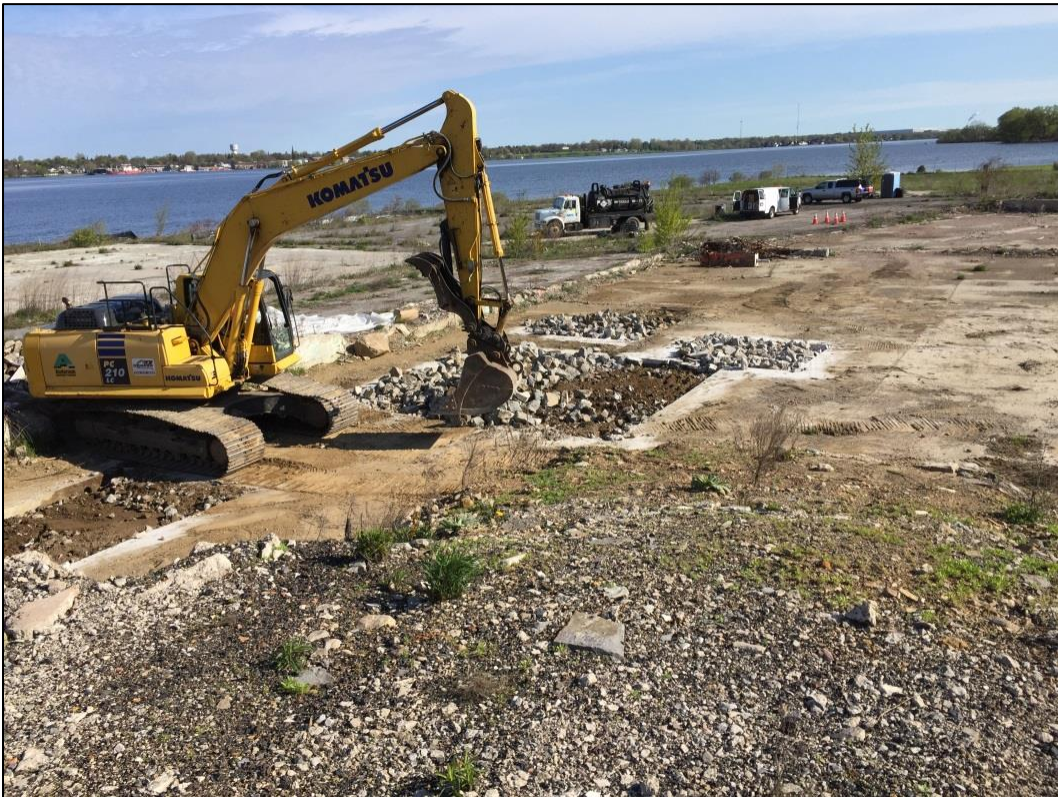
Removal of rubblized concrete from excavation areas.
