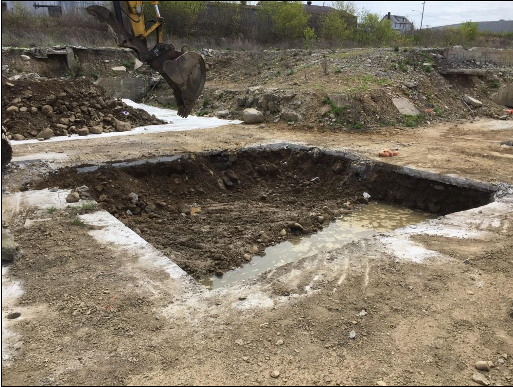
Excavation of 20'x20' pit (excavation depth ranged from 4' to 8').
