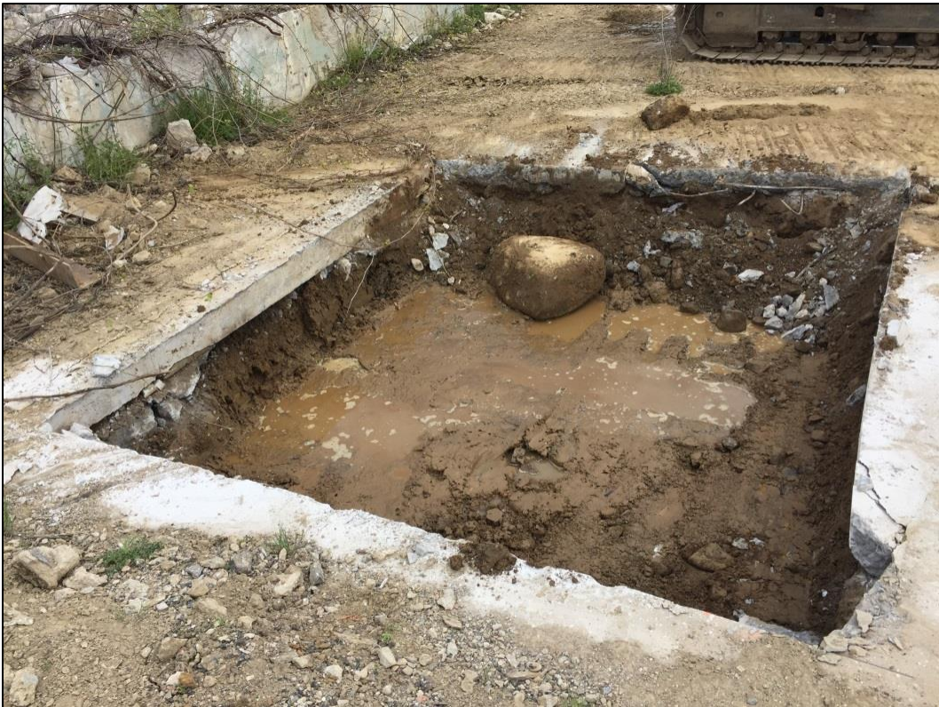
Completed excavation of western most pit (10'x10'x2'deep).
