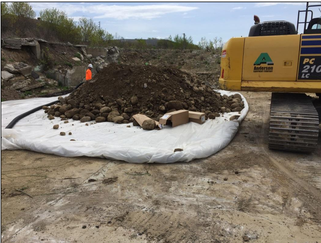
Soil stockpile area over 12-mil poly with bermed perimeter.
