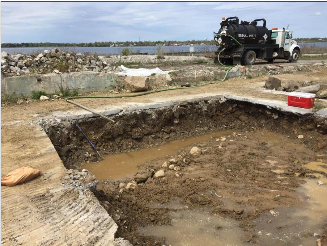
Excavation dewatering operations.
