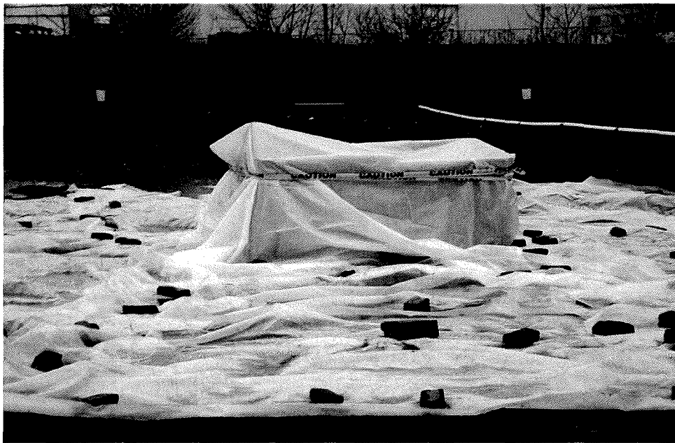
Photograph 2. Metal bins situated on and covered with poly sheeting.
