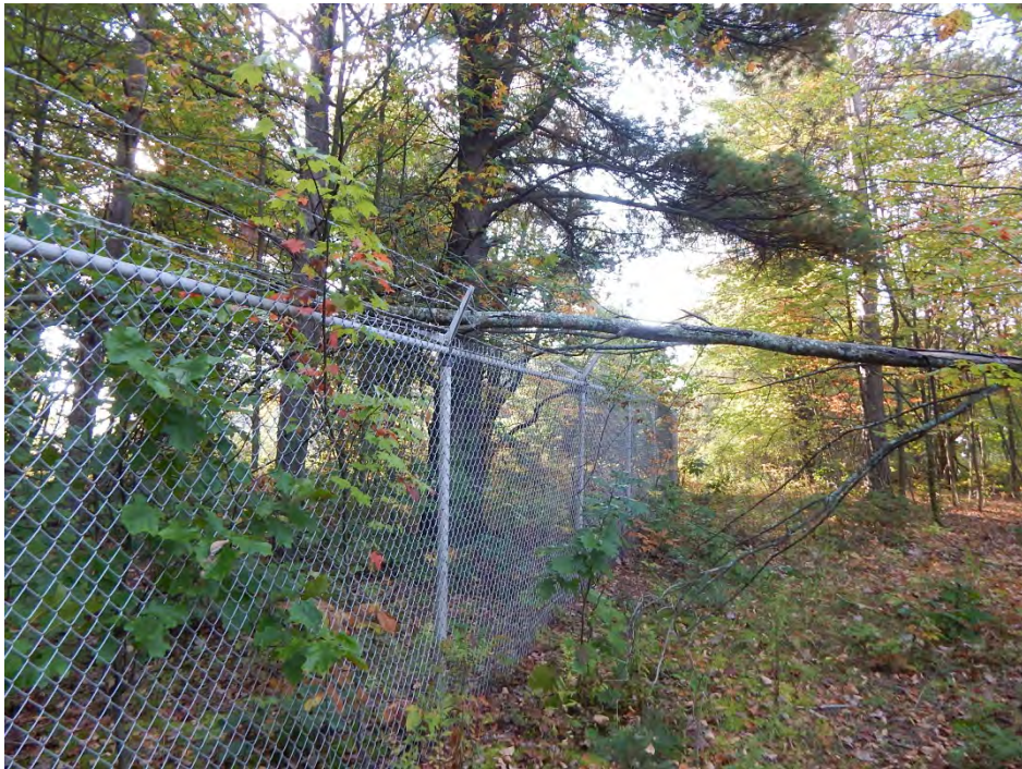
Photo 14: Small tree resting on fence in the northwest corner of the perimeter fence.
