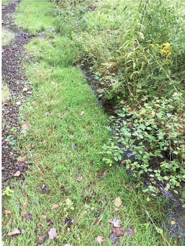
Photo 5: Looking west along the southern access road. The toe of the seep area with water breaking out along the length is to the right in the photo. Black fabric of the partially covered silt fence is faintly visible in the lower right.
