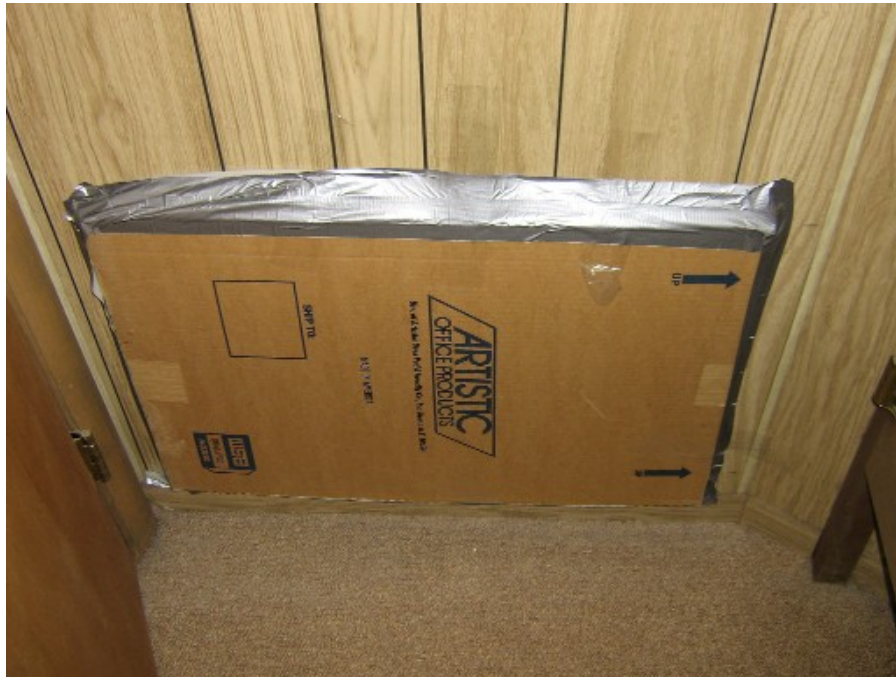
Photo 18 Sealed Vent in Washroom Near Executive Office – First Floor, Northside Looking South
