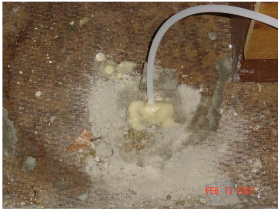
Photo 1 Sampling Location SS-1 Slab Penetration Sealed with Beeswax
