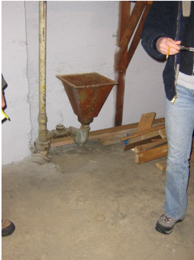
Photo 2 Drain Funnel – Basement Northeast Portion of Basement – Looking Southeast
