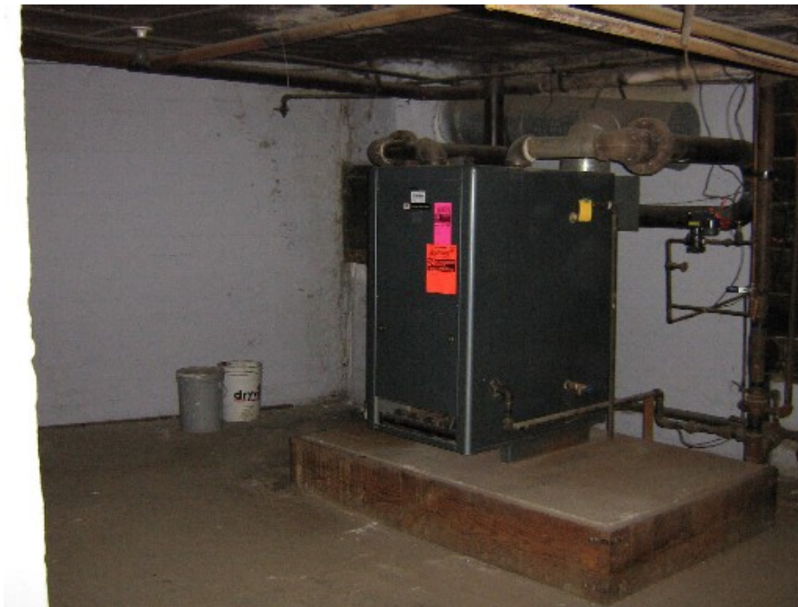
Photo 3 Natural Gas Fired Boiler – Basement Southeast Corner of Basement – Looking Southeast
