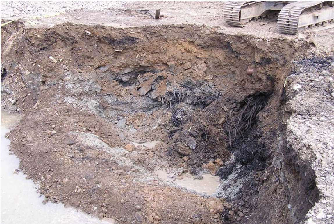
Photograph 2: View of rubber scraps within the fill at the Area H Gannett Parcel Excavation.
