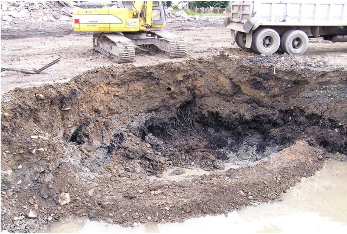
Photograph 1: View of rubber scraps within the fill at the Area H Gannett Parcel Excavation.
