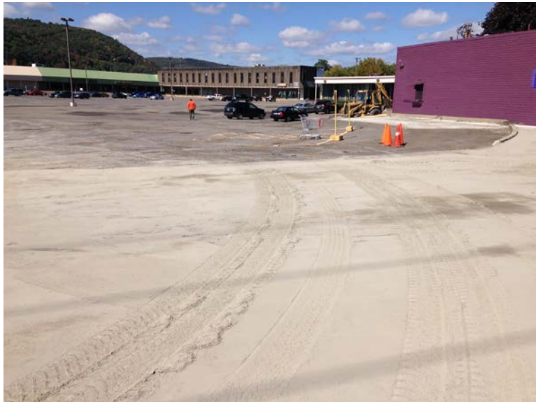
September 22, 2014, base material placement (Areas 2-7)
