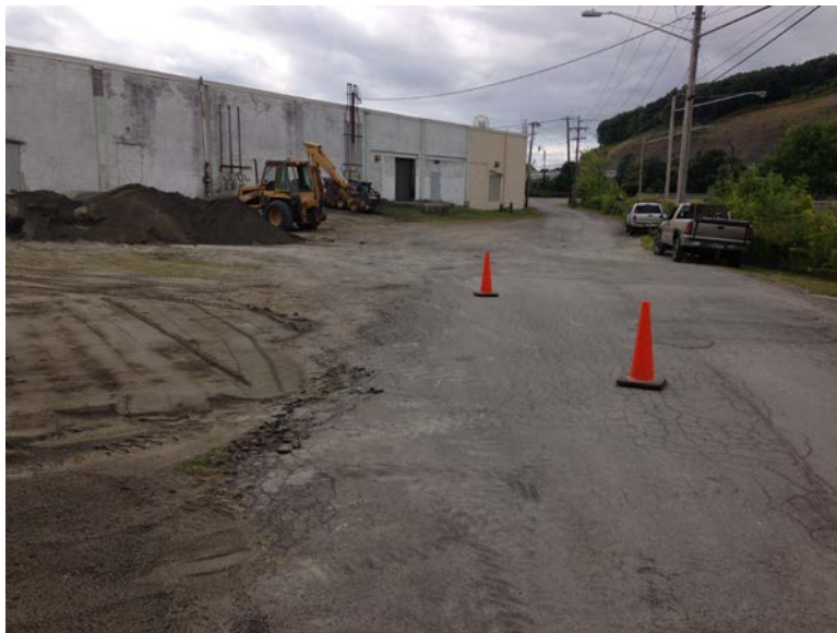
September 9, 2014, Area 1, placing and grading base material
