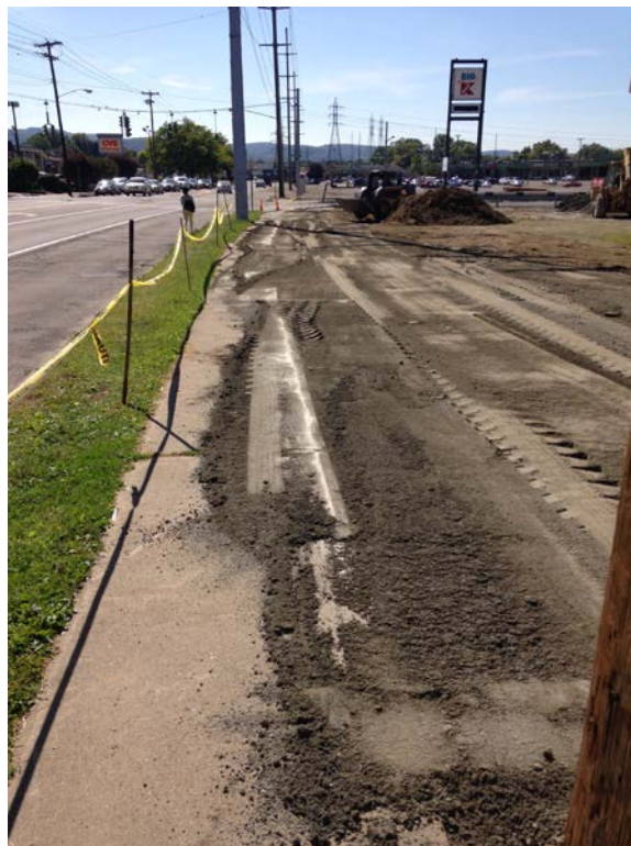
September 22, 2014, grading and base material placement (Area 16)
