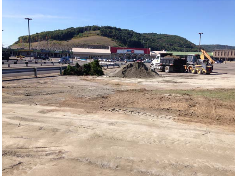
September 22, 2014, grading and base material placement (Area 16)
