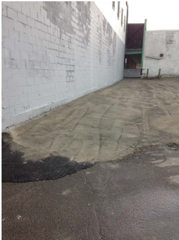
September 11, 2014, Area 1, partially completed base layer
