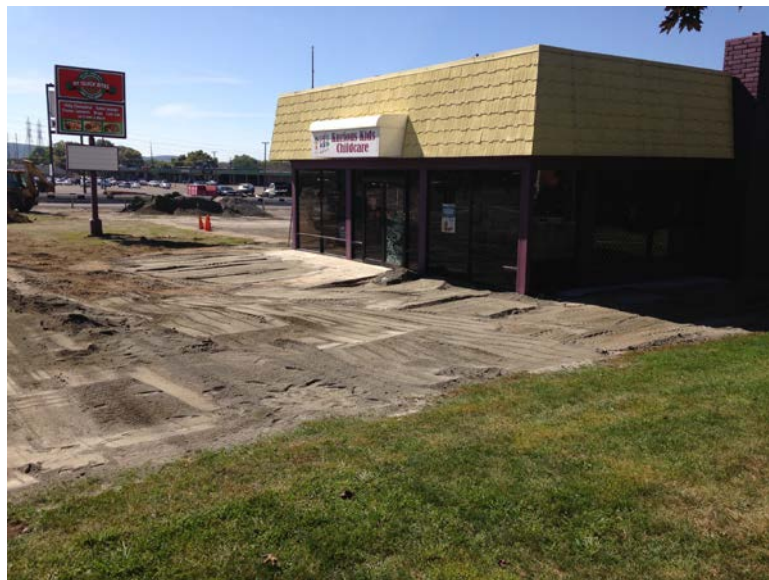
September 22, 2014, grading and base material placement (Area 16)
