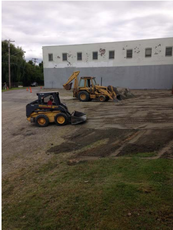
September 9, 2014, Area 1, placing and grading base material
