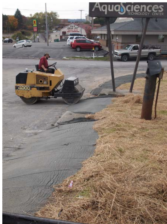
October 20, 2014 Placing base material for transition to existing grade (Area 9).
