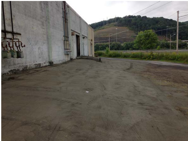
September 11, 2014, Area 1, partially completed base layer
