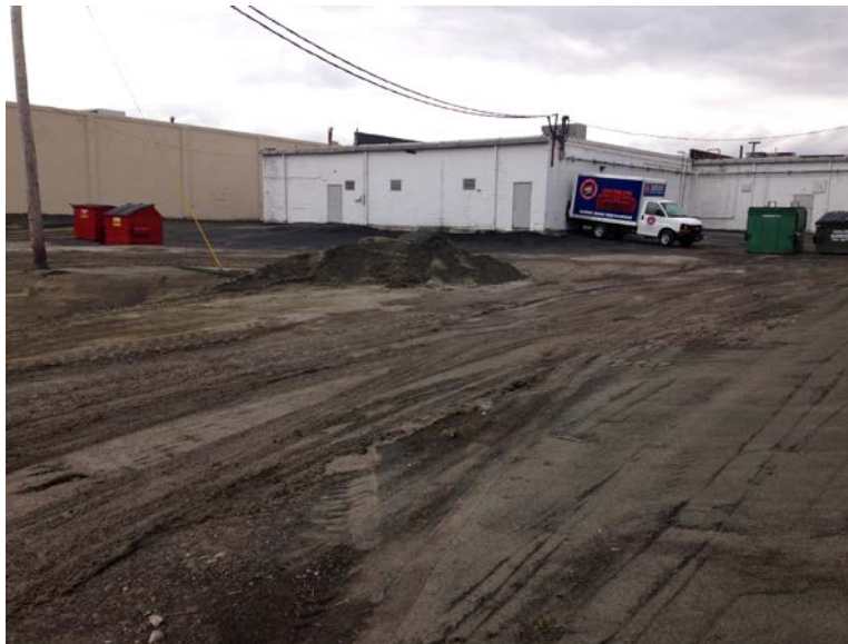
September 16, 2014, partially placed base material in Areas 2-6. At the time of photo, work suspended in this area due to rain and pool drainage
