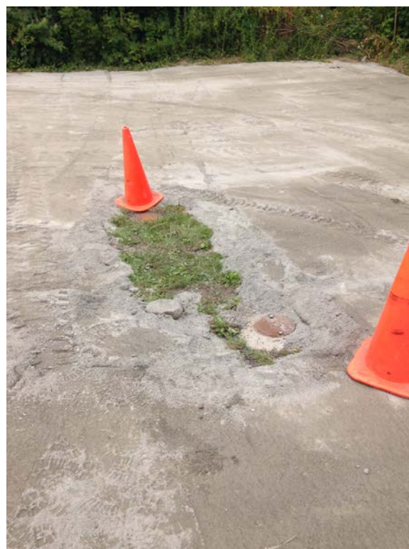
September 9, 2014, Area 13, flush-mount wells prior to raising
