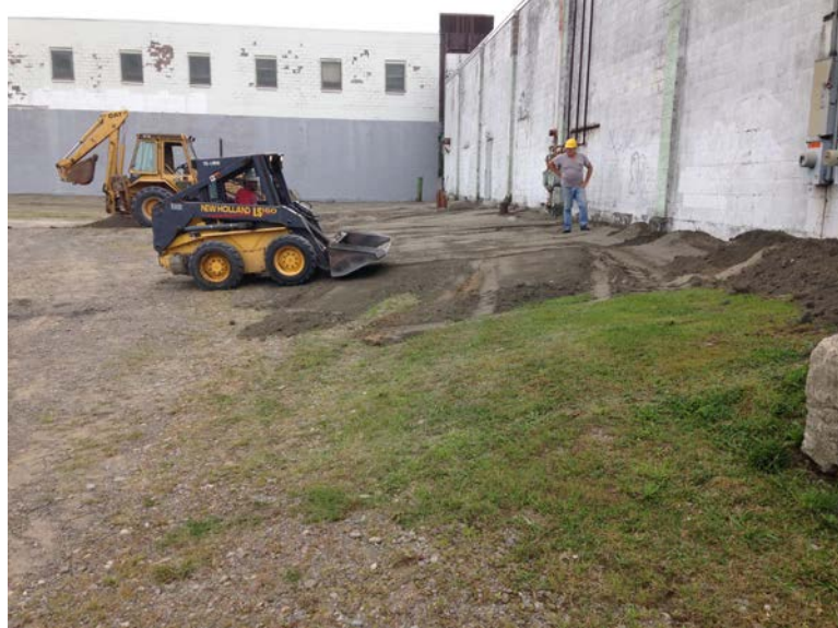
September 9, 2014, Area 1, placing and grading base material
