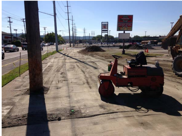
September 22, 2014, grading and base material placement (Area 16)
