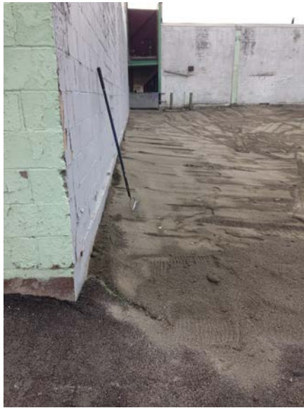
September 9, 2014, Area 1, placing and grading base material
