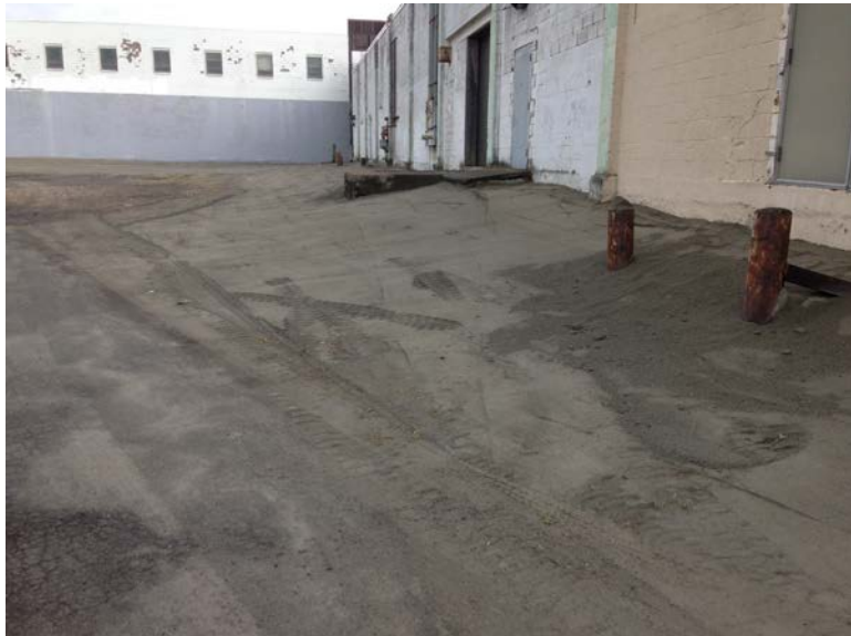
September 11, 2014, Area 1, partially completed base layer
