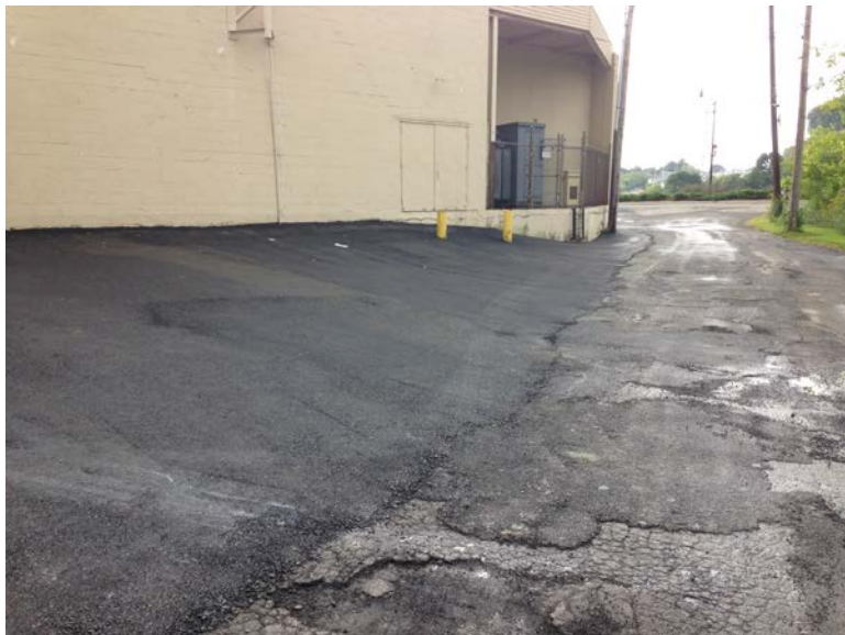
September 11, 2014, fresh paving placed in northwest portion of Area 1 to stabilize downspout area prior to expected rain.
