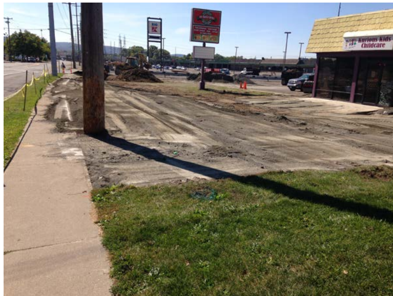
September 22, 2014, grading and base material placement (Area 16)
