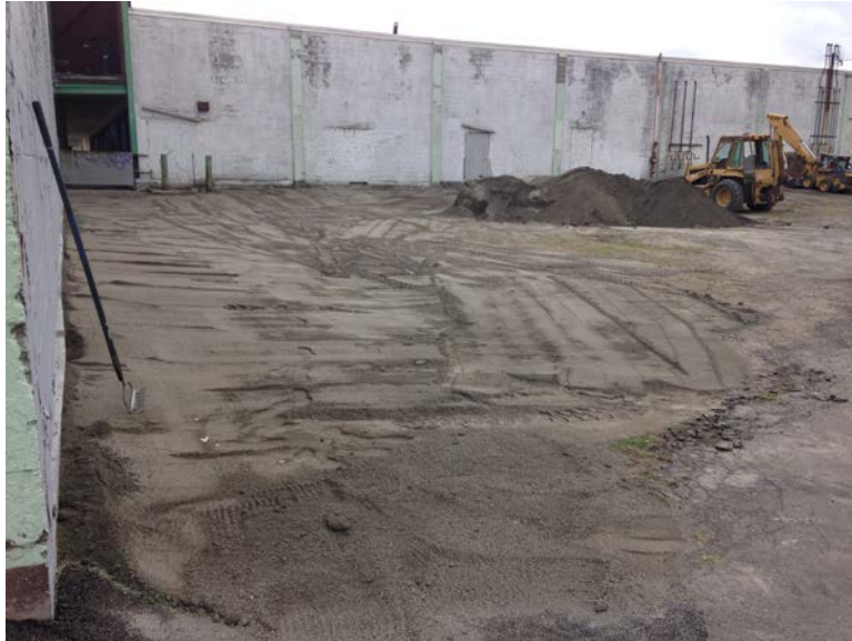
September 9, 2014, Area 1, placing and grading base material
