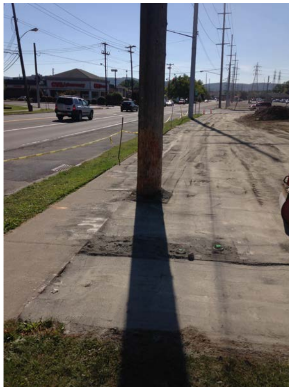
September 22, 2014, grading and base material placement (Area 16)
