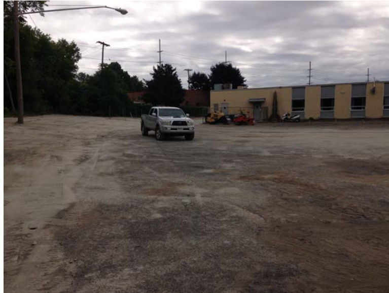
September 9, 2014, Area 13 base material placed prior to paving
