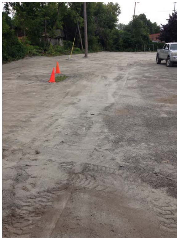
September 9, 2014, Area 13 base material placed prior to paving
