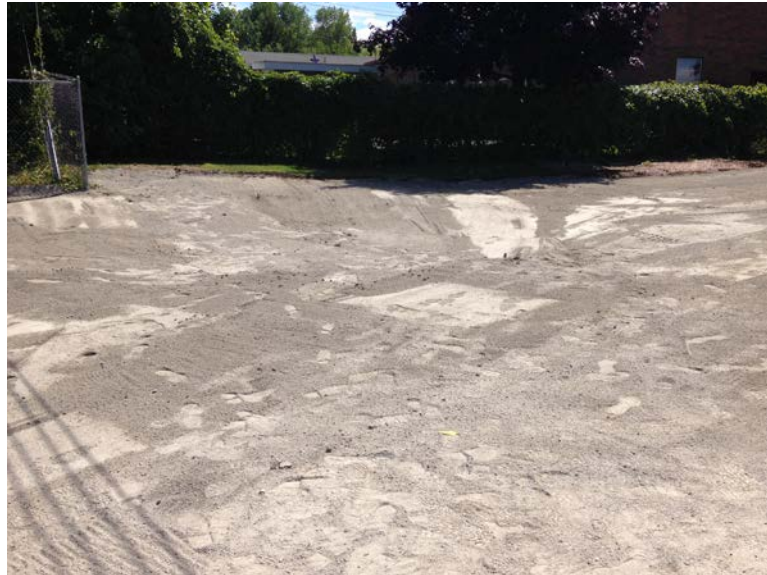
September 8, 2014, Area 13, placing base material
