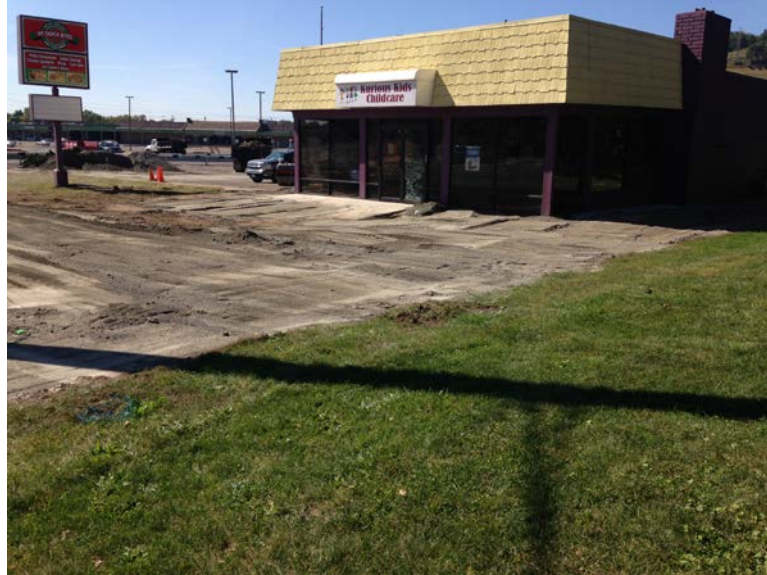
September 22, 2014, grading and base material placement (Area 16)
