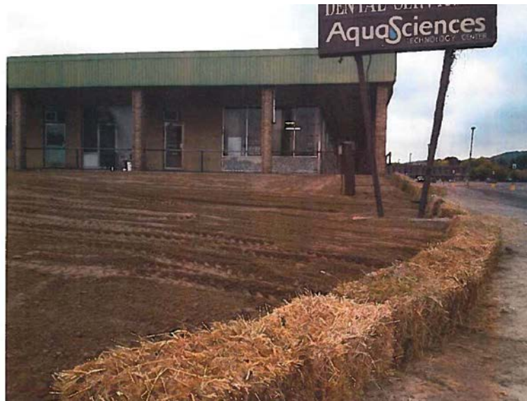
October 7, 2014, Clean soil cover in Area 9 and hay bale barrier for erosion control
