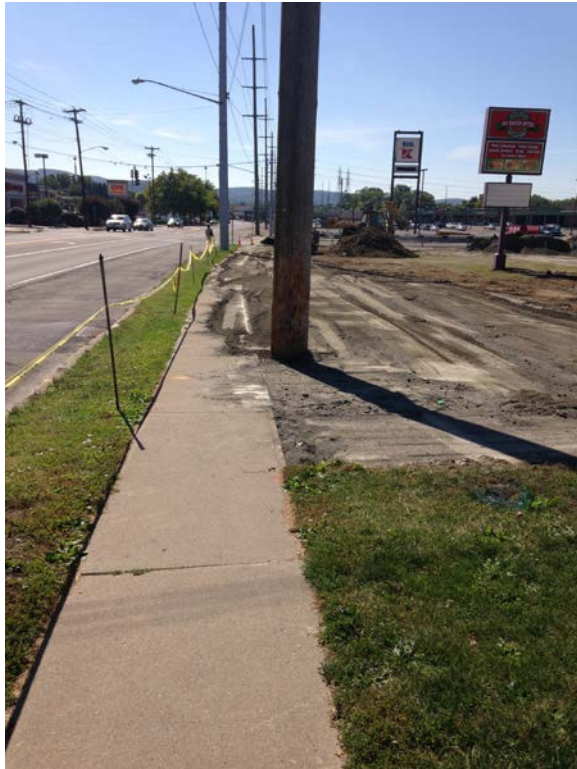
September 22, 2014, grading and base material placement (Area 16)
