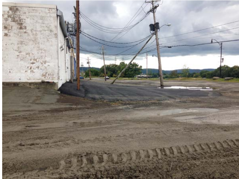
September 16, 2014, partially placed base material in Areas 2-6. At the time of photo, work suspended in this area due to rain and pool drainage
