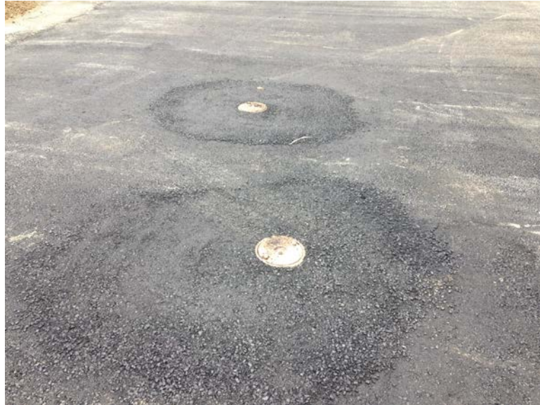
September 16, 2014, Area 13 well flush-mount after paving
