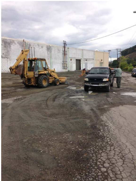
September 16, 2014, continued place mark of base material in Area 1.
