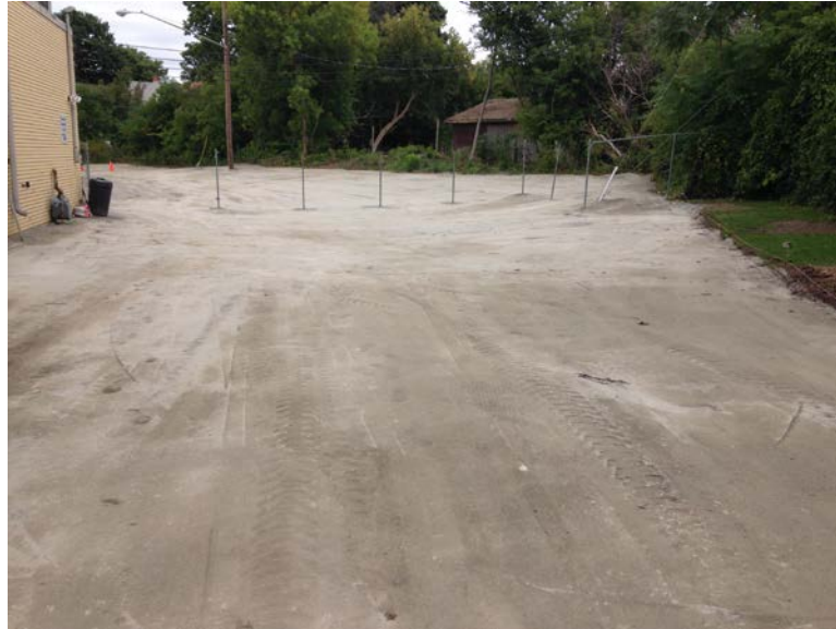
September 9, 2014, Area 13, flush-mount wells prior to raising
