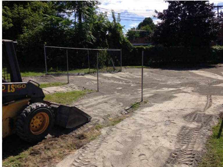
September 8, 2014, Area 13, placing base material
