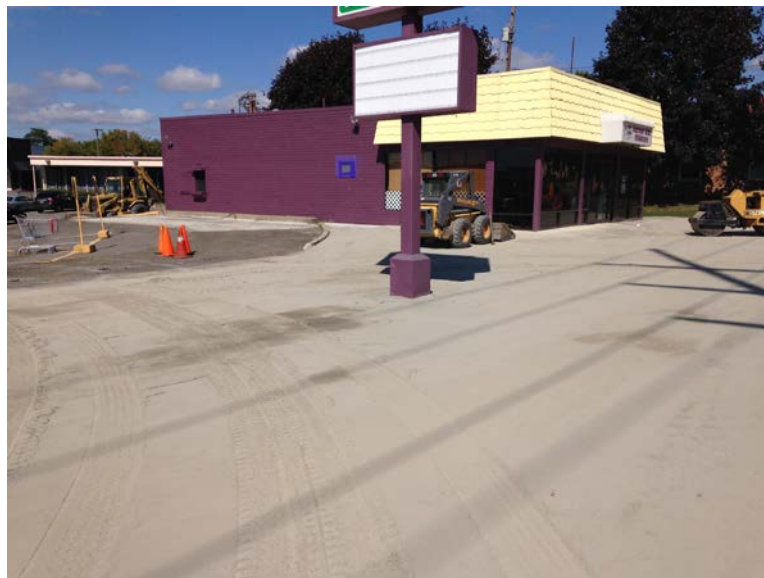
September 22, 2014, base material placement (Areas 2-7)
