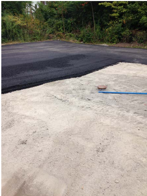
September 12, 2014, Area 13 well flush-mount raised and awaiting paving
