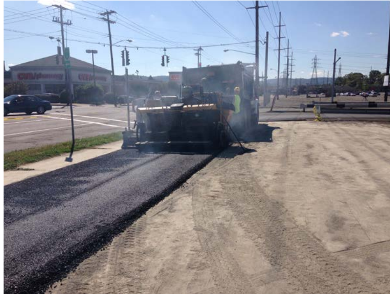
September 22, 2014, base material placement (Areas 2-7)
