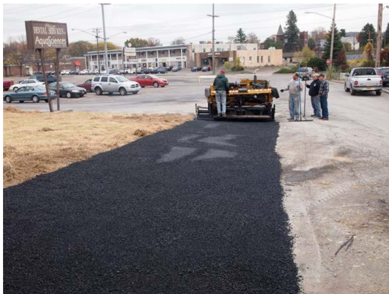
October 20, 2014, Area 9. Paving grade transition.
