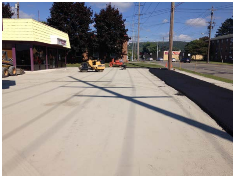
September 22, 2014, base material placement (Areas 2-7)
