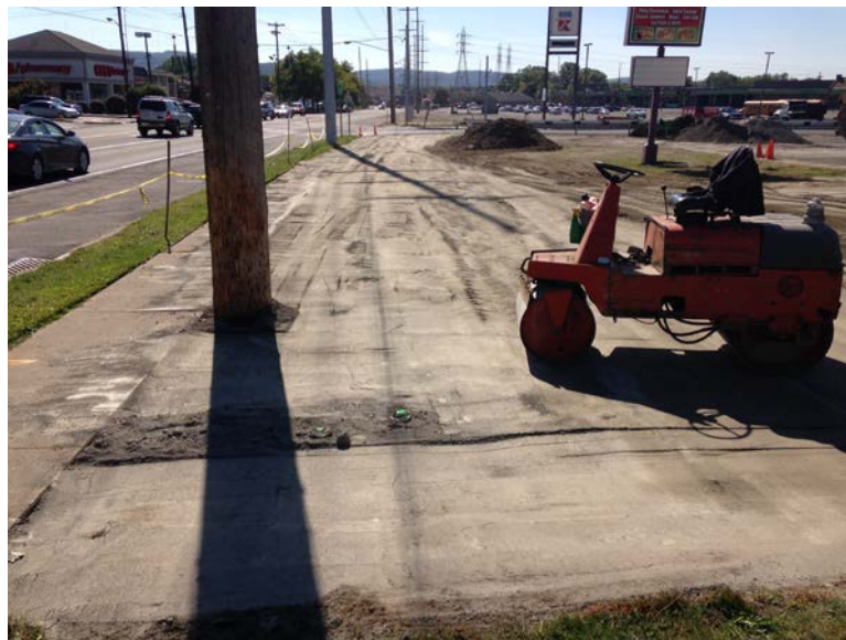
September 22, 2014, grading and base material placement (Area 16)
