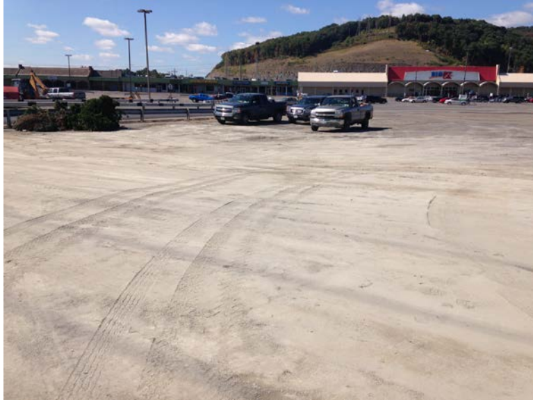
September 22, 2014, base material placement (Areas 2-7)
