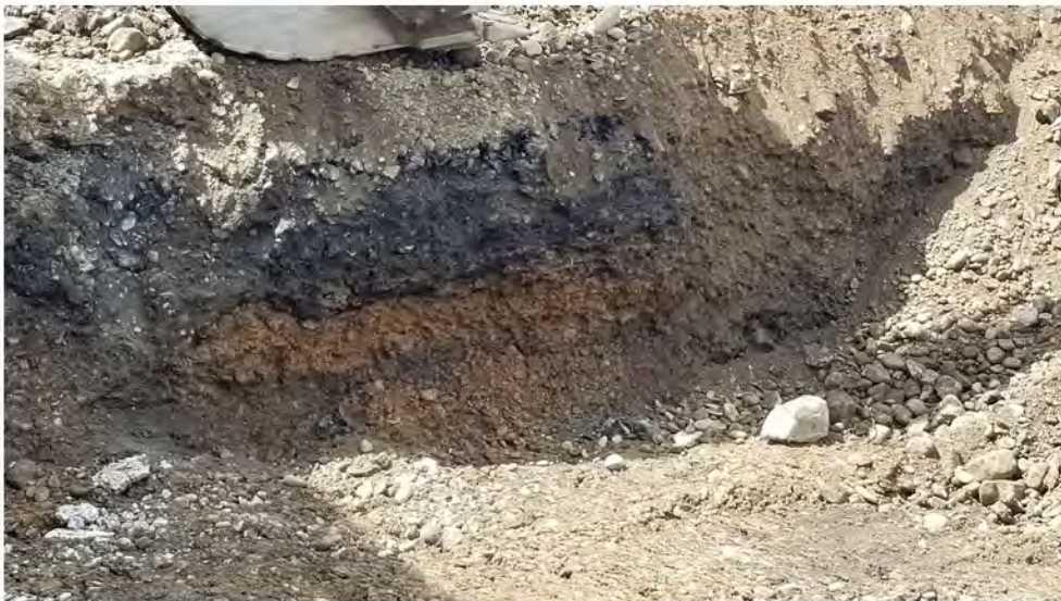
Rail bed visible in western wall of loading dock excavation 2022-05-18 14:53
