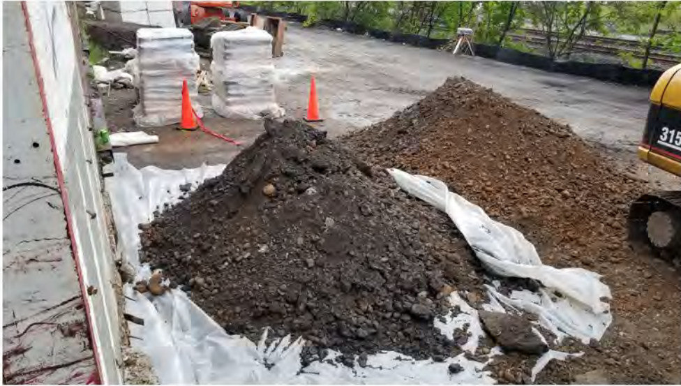
Staged rail bed materials 2022-05-19 09:40
