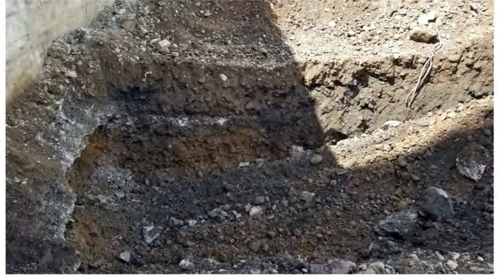
Loading dock excavation 2022-05-18 13:25
