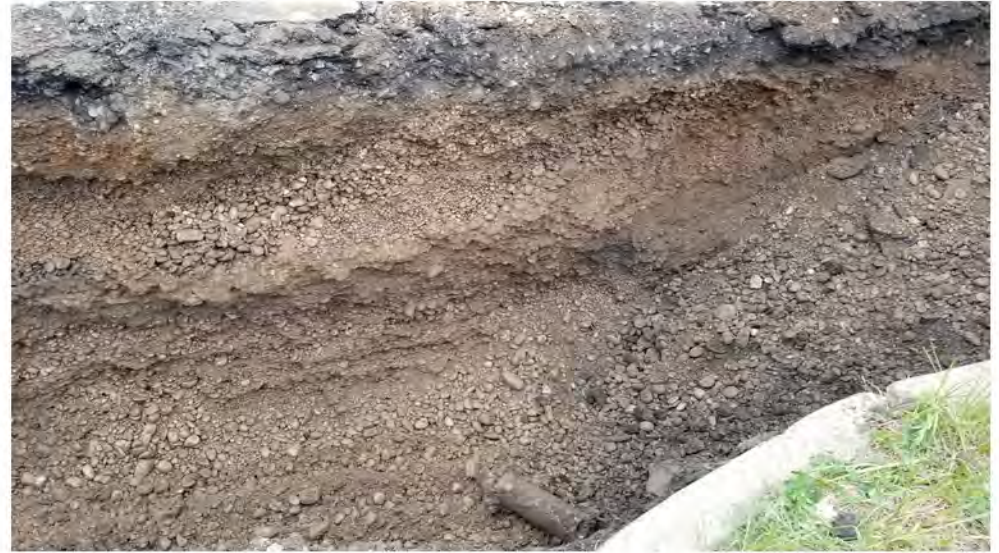
Helen Drive near Avenue B 2022-05-16 13:08
