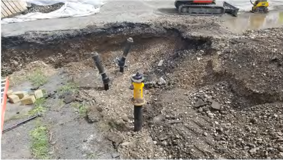
Trench from Helen Drive to corner hydrant. 2022-05-17 11:58
