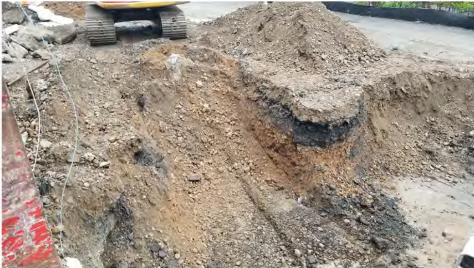
Western extension of loading dock excavation 2022-05-19 09:27
