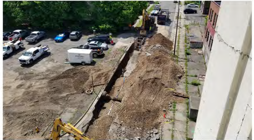
Aerial view of Avenue B 2022-05-18 11:59
