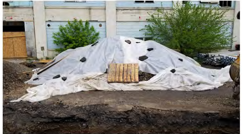
Main pile of gasoline-contaminated soil 2022-05-16 13:21
