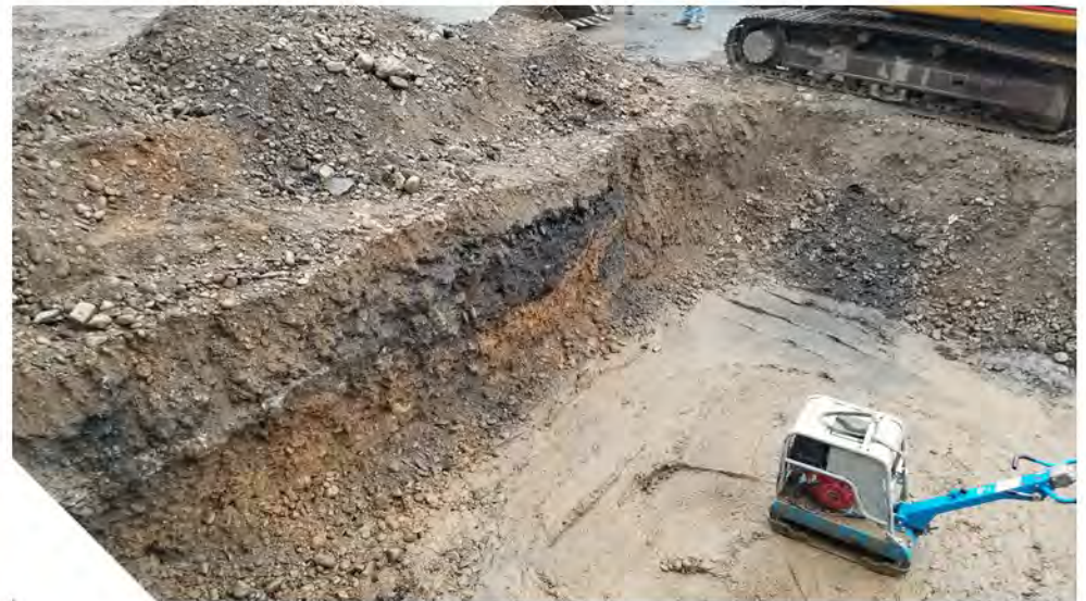
Western wall of loading dock excavation 2022-05-19 07:42
