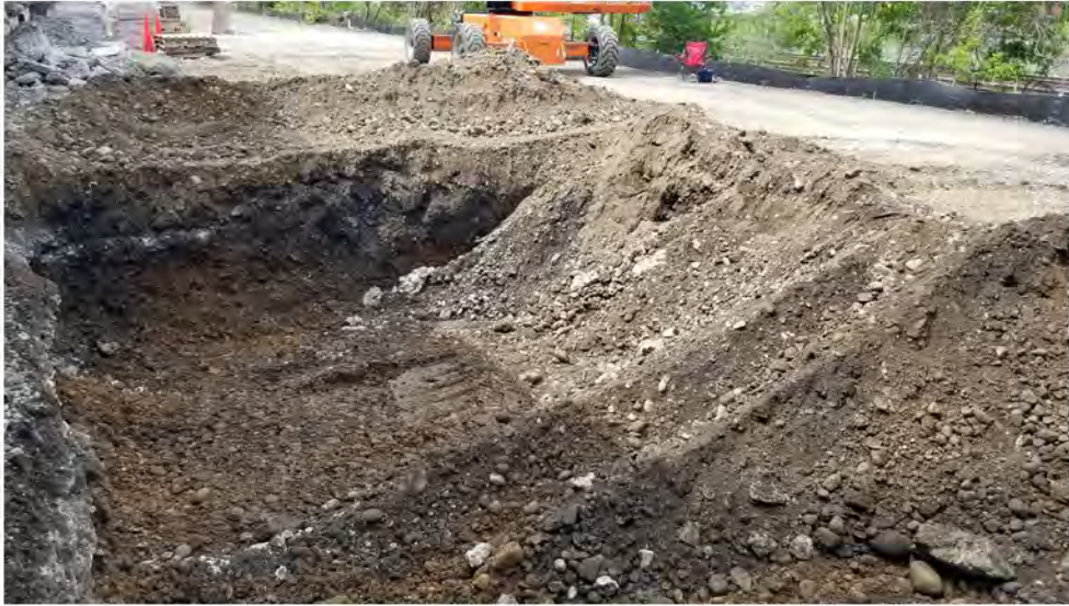
Loading dock excavation 2022-05-18 14:19
