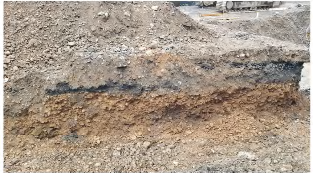
Rail bed visible along northern wall of loading dock extension 2022-05-19 11:15
