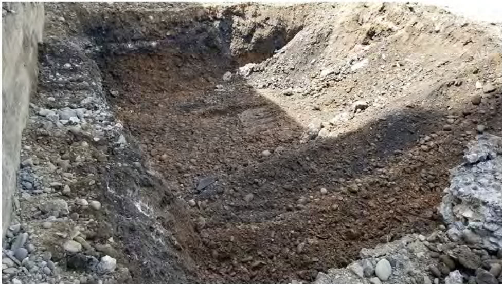
Loading dock excavation 2022-05-18 14:08
