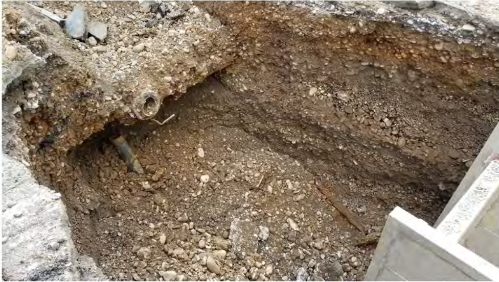
Avenue B trench 2022-05-17 15:31
