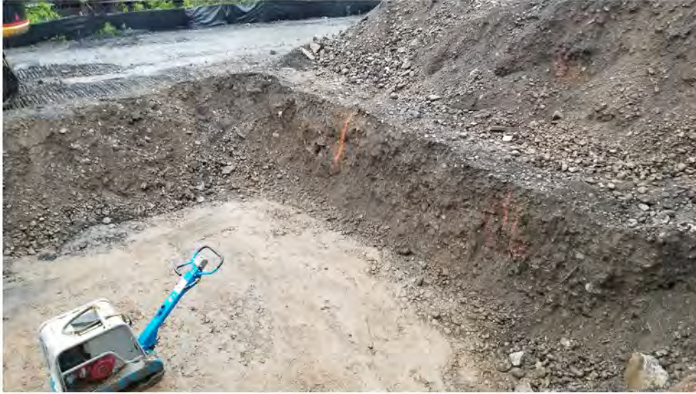
Eastern wall of loading dock excavation 2022-05-19 07:42
