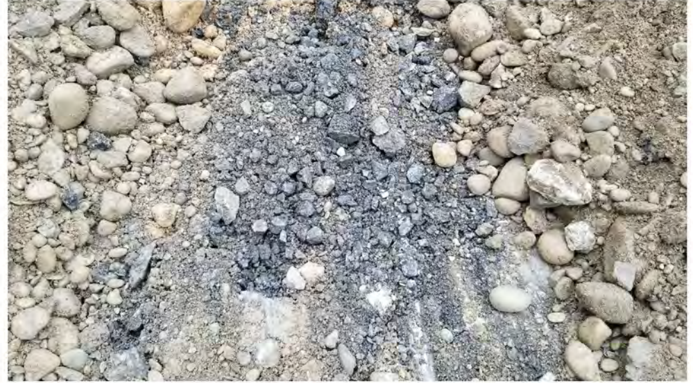
Typical rail bed material 2022-05-19 08:19
