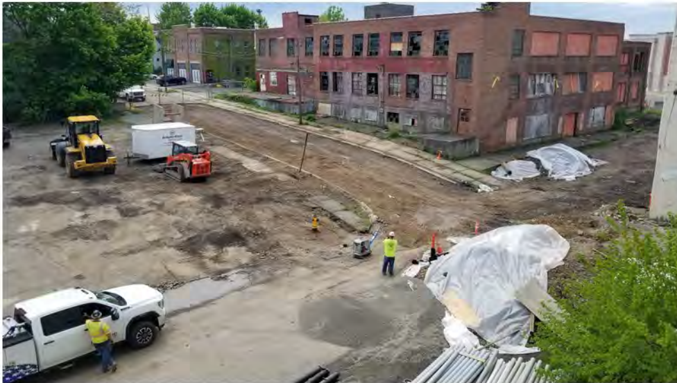
Aerial view of Avenue B (background) and Helen Drive (foreground) 2022-05-20 14:27
