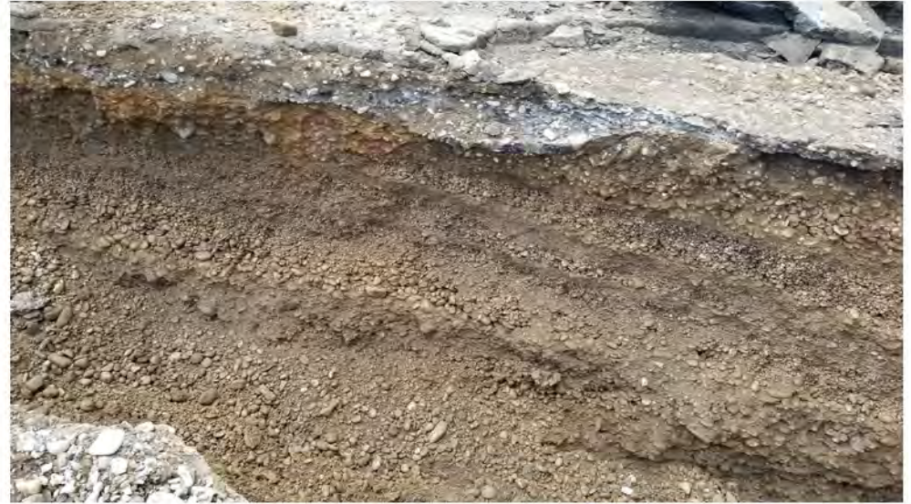
Avenue B trench 2022-05-17 14:06
