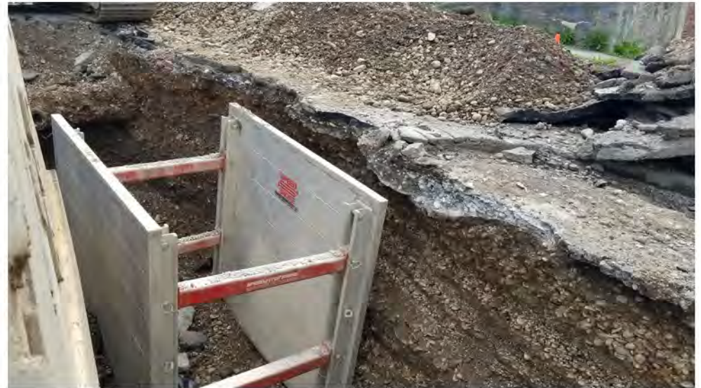
Avenue B trench 2022-05-17 15:30
