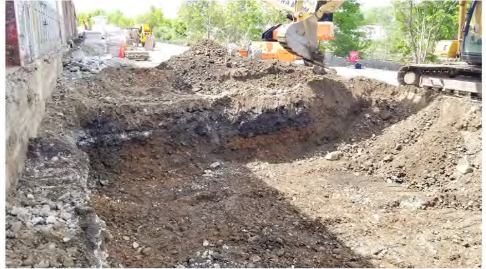
Loading dock excavation 2022-05-18 14:53
