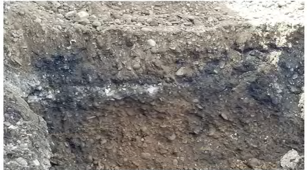
Stained soil at western wall of loading dock excavation 2022-05-18 14:09
