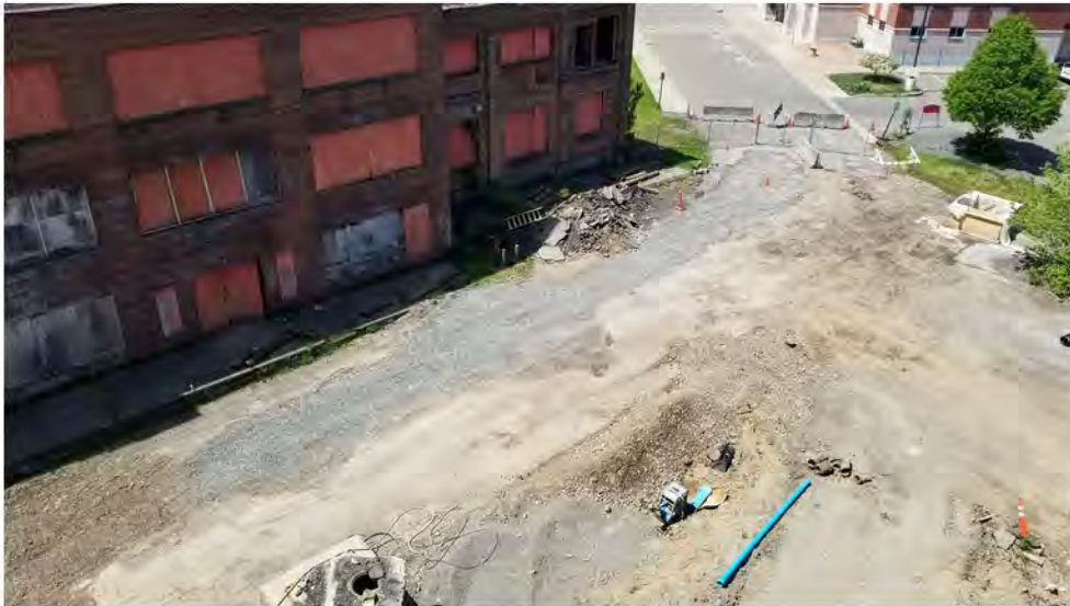
Aerial view of western portion of Helen Drive 2022-05-18 11:58
