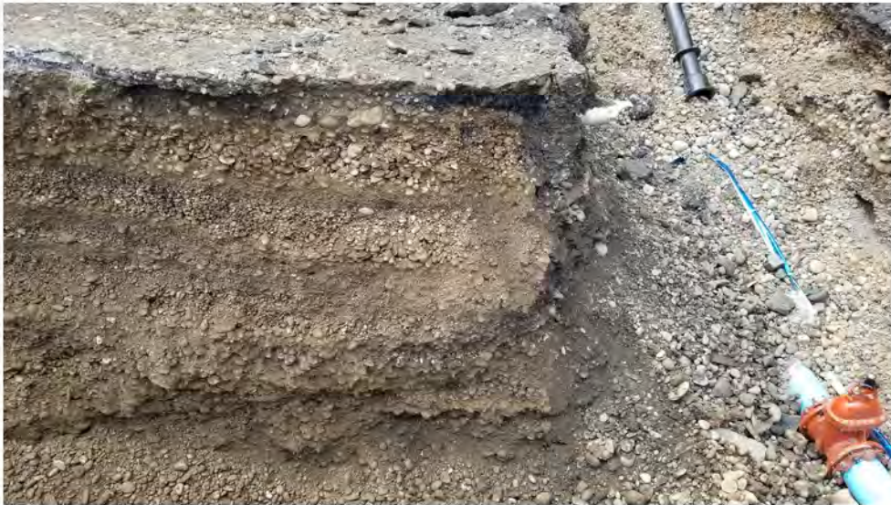
Corner of Helen Drive and Avenue B trenches 2022-05-17 14:07
