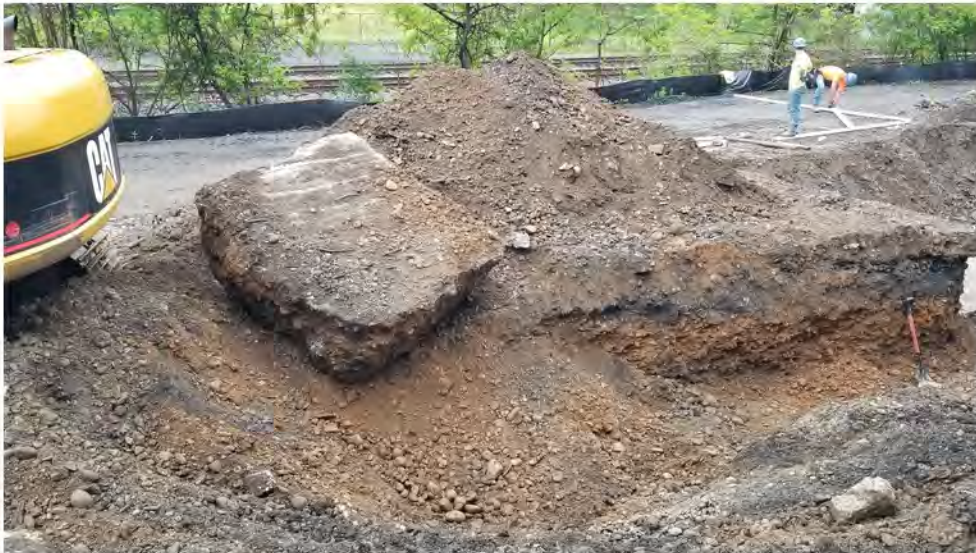
Foundation within loading dock extension 2022-05-19 10:31
