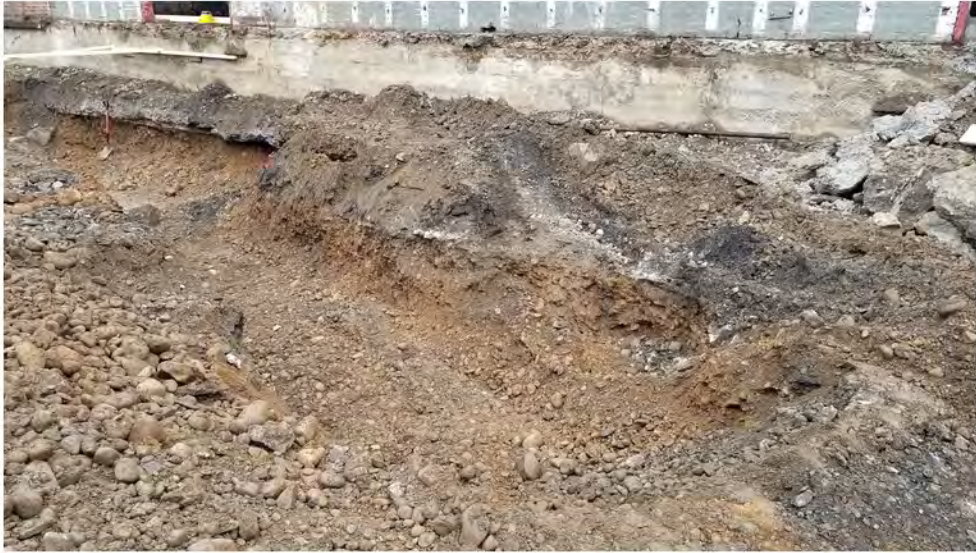
Southern wall of loading dock extension 2022-05-19 11:16
