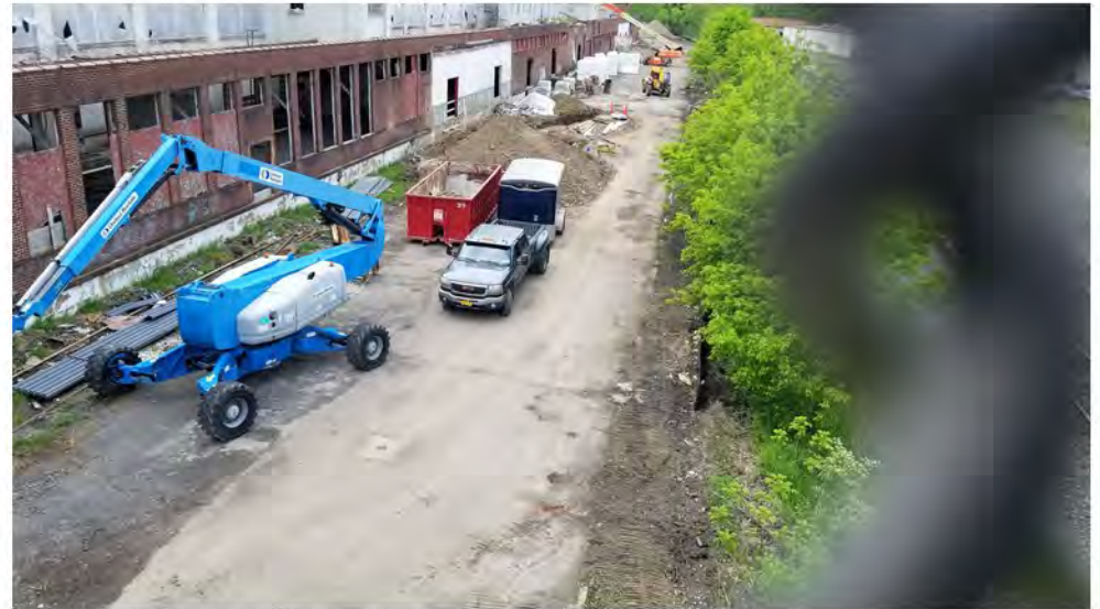
Aerial view of loading dock excavation 2022-05-20 14:33
