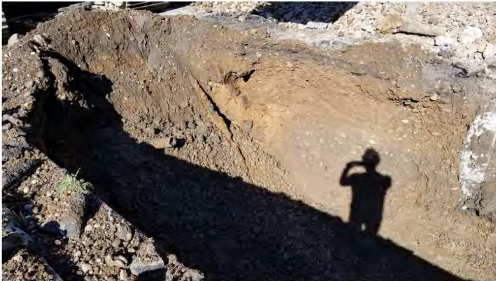
Avenue B trench 2022-05-18 08:27
