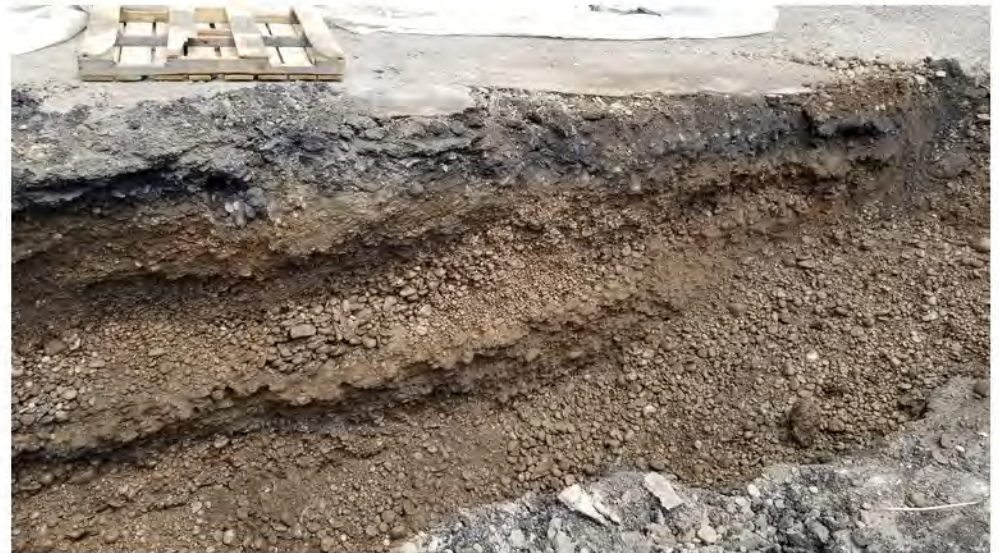
Helen Drive near Avenue B 2022-05-16 12:57
