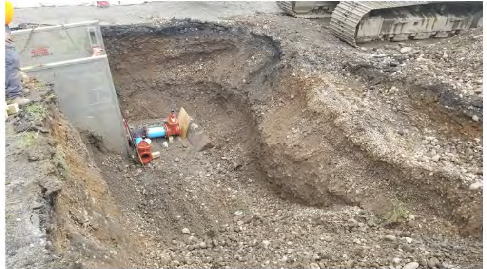
Trench from Helen Drive to corner hydrant. 2022-05-17 09:51
