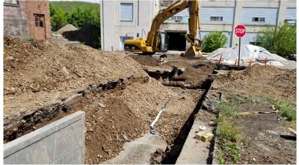
Avenue B trench 2022-05-18 11:33
