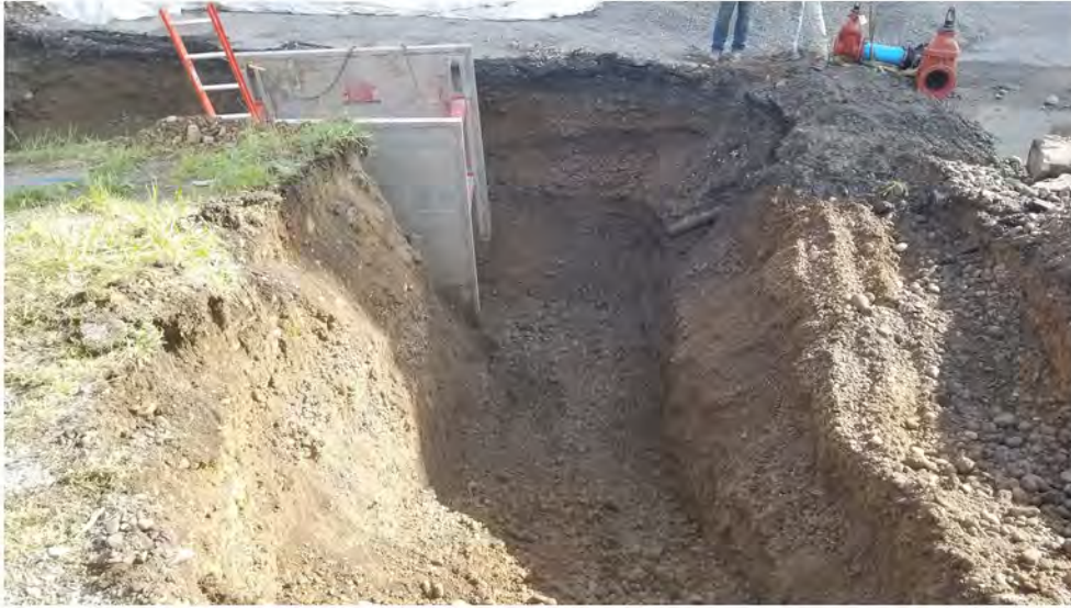
Trench from Helen Drive to corner hydrant. 2022-05-17 08:50
