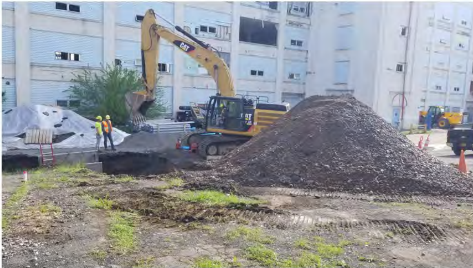
Clean soils excavated from hydrant trench 2022-05-17 08:51
