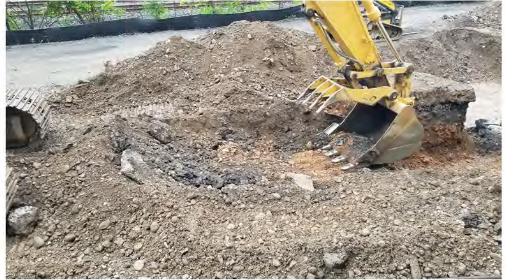
Western extension of loading dock excavation 2022-05-19 09:40
