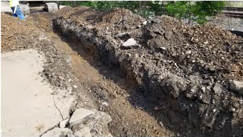
2022-06-01 08:54 42.1157322 N , 75.9510126 W Typical trench along Avenue C
