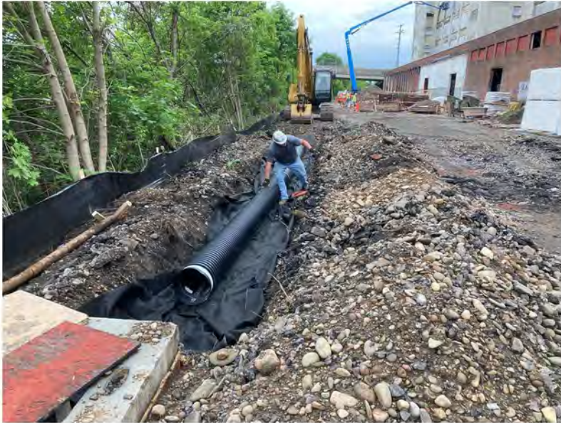
2022-06-02 08:15 42.1159361 N , 75.9516444 W Typical pipe installation along Avenue C
