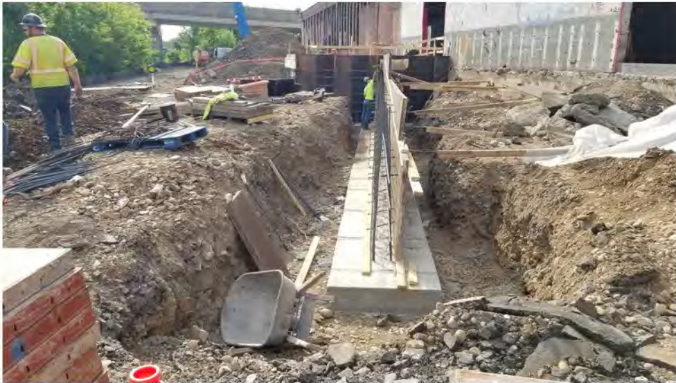
2022-06-01 08:58 42.1157041 N , 75.9512283 W Loading dock foundation progress along Avenue C
