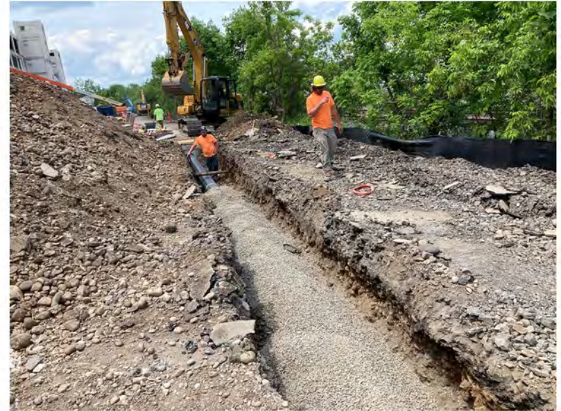
2022-05-31 13:24 42.1156667 N , 75.9507222 W Typical section of trench along Avenue C
