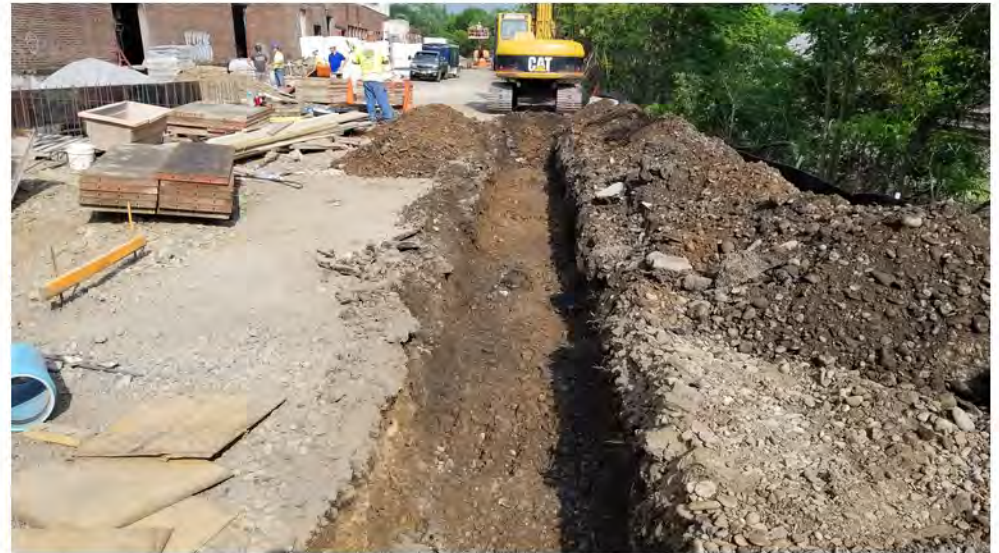
2022-06-01 08:55 42.1112048 N , 75.9577543 W Typical trench along Avenue C
