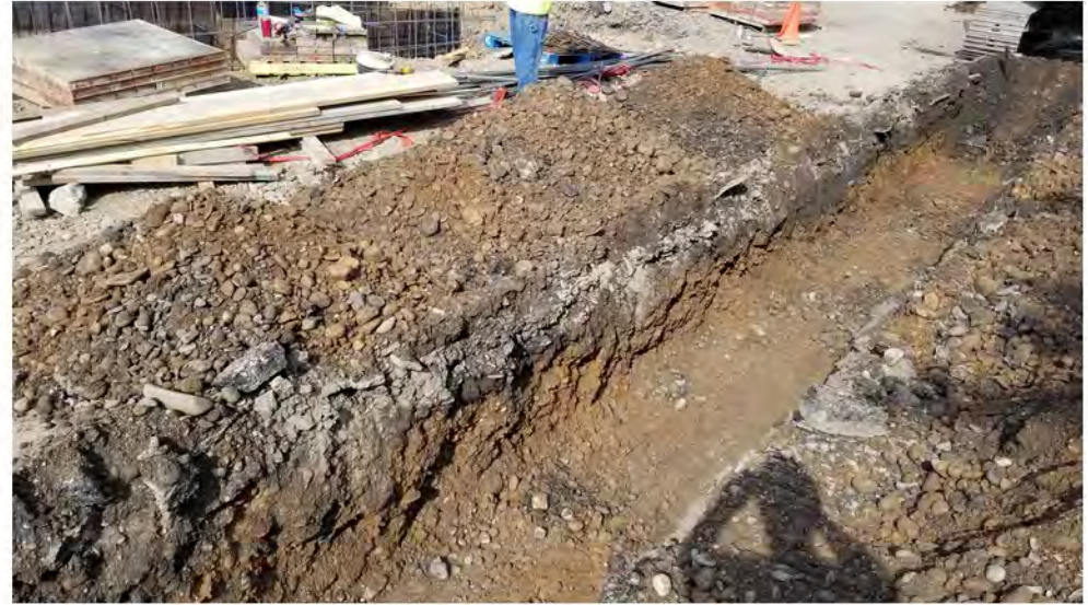
2022-06-01 08:57 42.1165448 N , 75.9526167 W Typical trench along Avenue C
