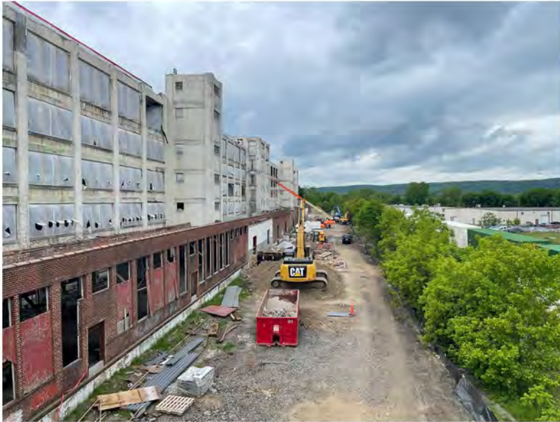
2022-05-27 13:14 42.1156194 N , 75.9503250 W Aerial view of Avenue C, looking west
