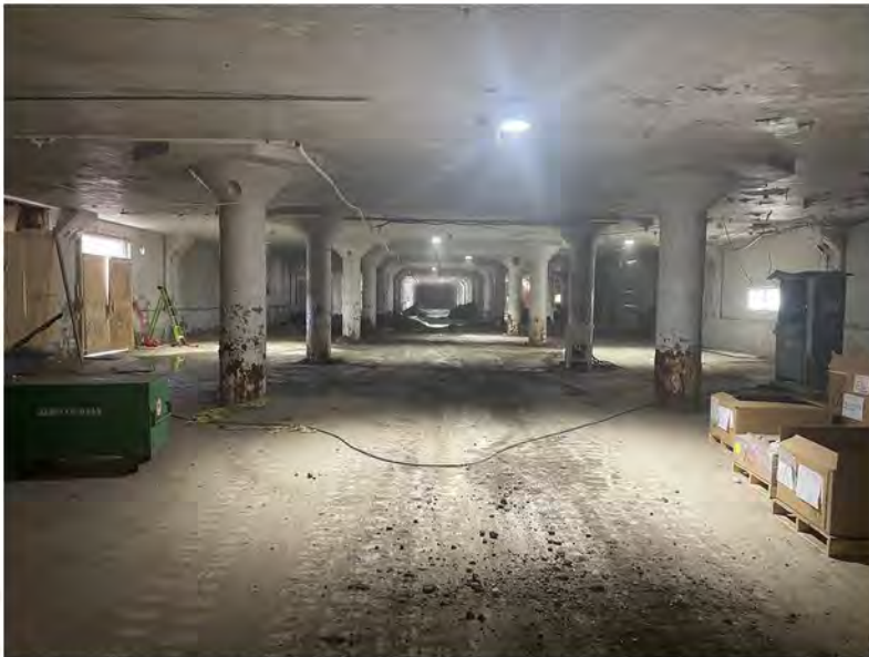
2022-05-25 11:31 42.1149528 N , 75.9518139 W Interior trench soils removed from ground floor of building
