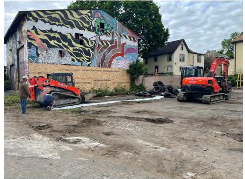
2022-05-25 09:17 42.1152917 N , 75.9511111 W Temporary exterior staging area for interior trench soils
