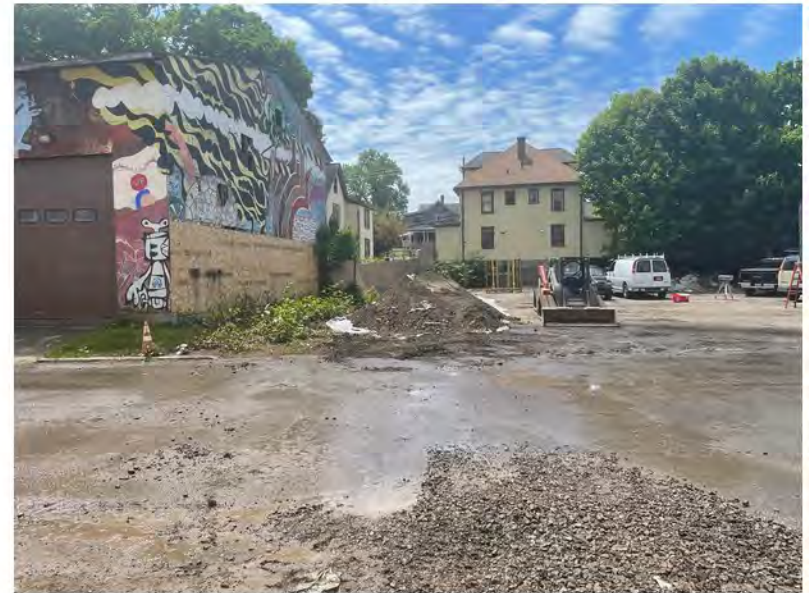
2022-05-25 12:48 42.1153333 N , 75.9509722 W Temporary exterior staging area for interior trench soils
