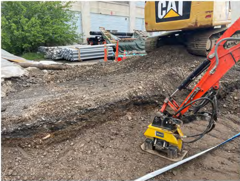
2022-05-24 12:43 42.1156278 N , 75.9527194 W Helen Drive waterline installation, tamping backfill
