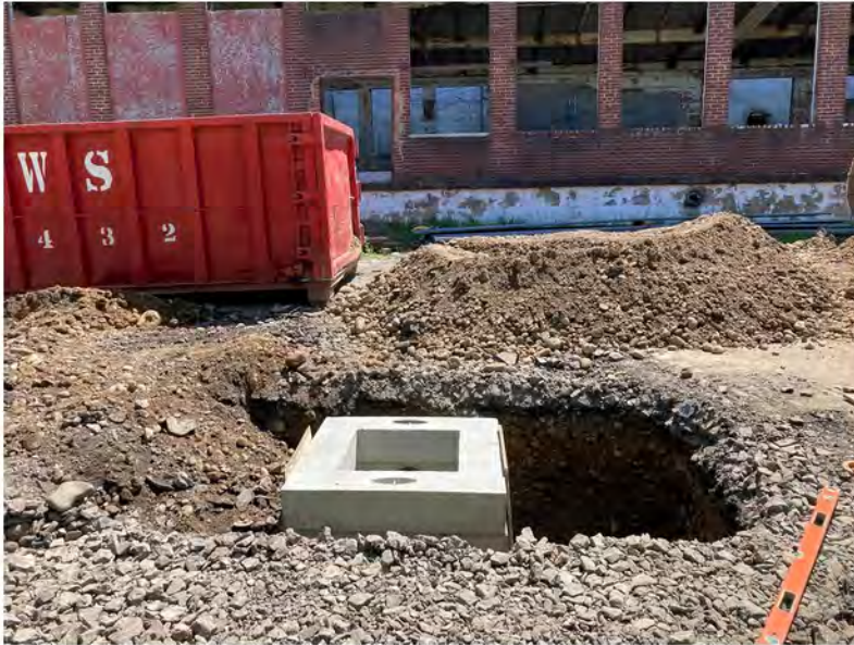
2022-05-25 14:28 42.1156778 N , 75.9507056 W Stormwater catch basin installation along Avenue C
