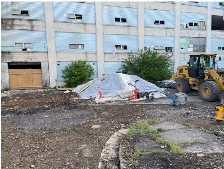
2022-05-23 07:23 42.1155750 N , 75.9528722 W Helen Drive at Avenue B, looking north
