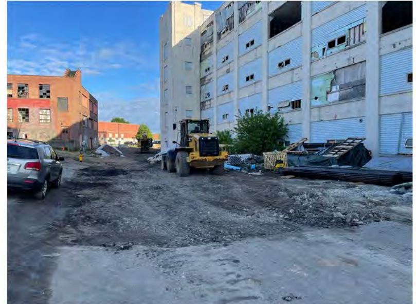
2022-05-24 07:36 42.1155611 N , 75.9524000 W Helen Drive, between Avenues A and B, looking west
