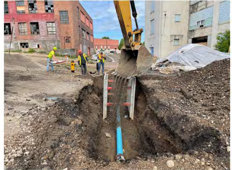
2022-05-24 09:31 42.1156056 N , 75.9526278 W Helen Drive waterline installation, placing clean bedding, looking west
