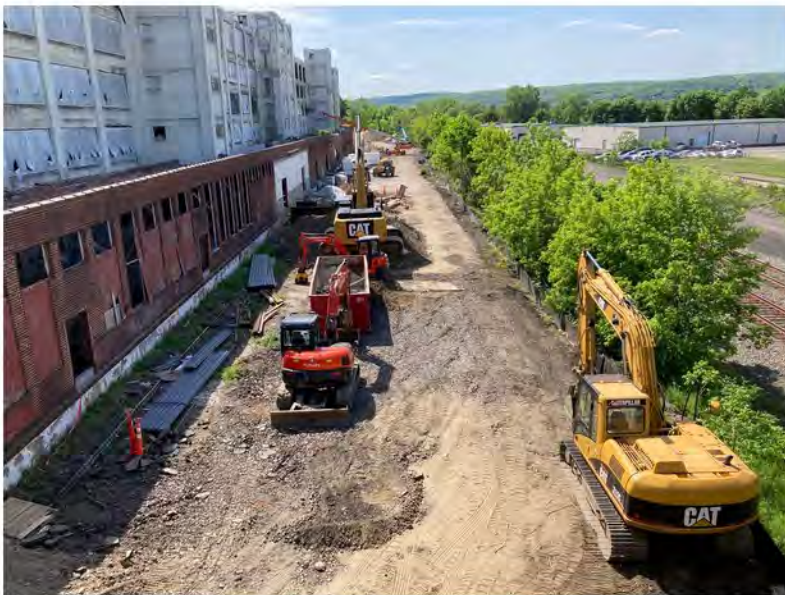
2022-05-25 15:39 42.1155667 N , 75.9502806 W Aerial view of Avenue C, looking west
