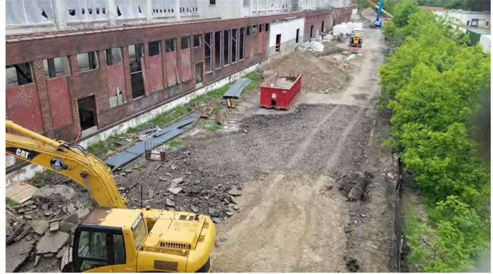
2022-05-23 15:12 0.000000 N , 0.000000 E Aerial view of Avenue C, looking west
