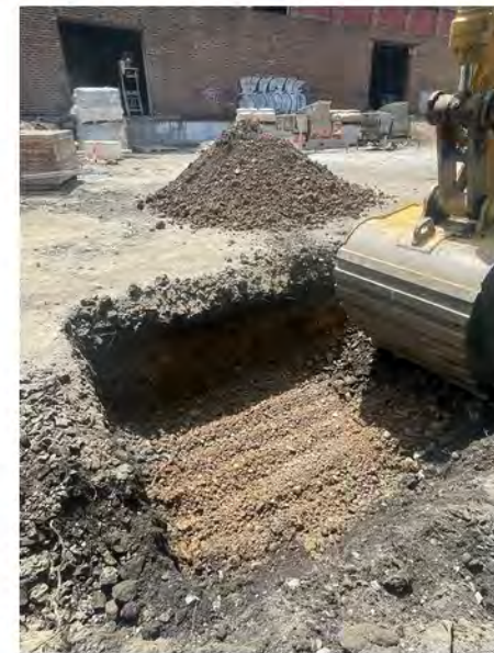
2022-05-26 13:24 42.1158056 N , 75.9512028 W Stormwater catch basin excavation along Avenue C
