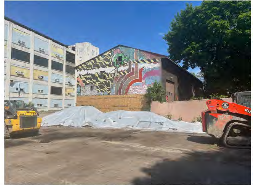
2022-05-25 15:27 42.1151111 N , 75.9513250 W Temporary exterior staging area for interior trench soils
