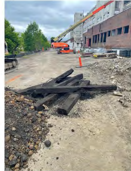
2022-05-27 11:42 42.1209139 N , 75.9531111 W Railroad ties unearthed during storm sewer excavation
