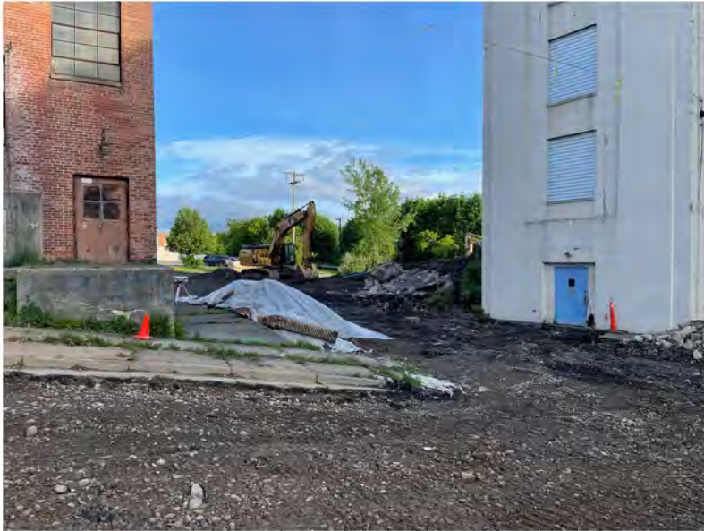
2022-05-23 07:23 42.1155750 N , 75.9528667 W Helen Drive (Work Zone #1) at Avenue B, looking west
