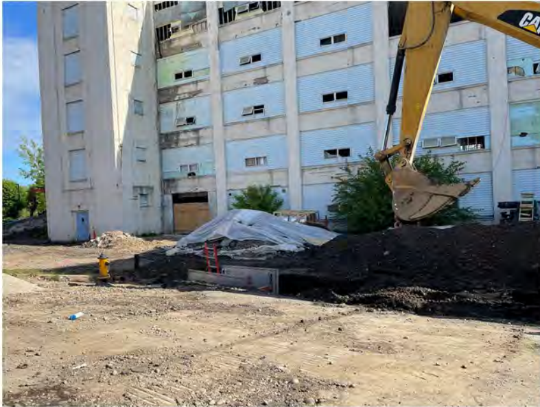
2022-05-24 09:03 42.1150361 N , 75.9528889 W Helen Drive waterline installation, looking northwest
