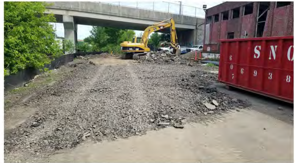
2022-05-23 15:02 0.0000000 N , 0.0000000 E Northeast corner of Avenue C (Work Zone #2)
