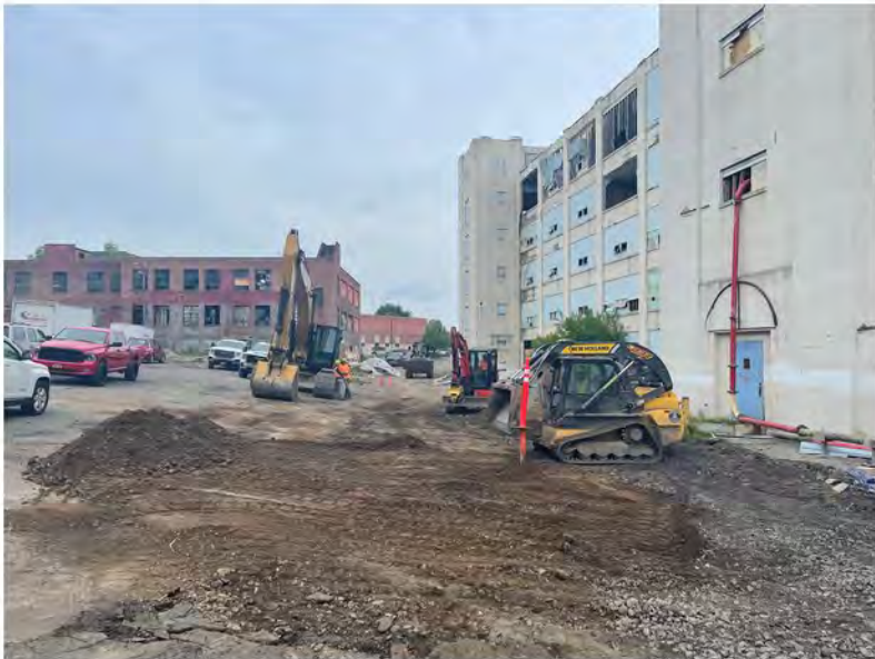
2022-06-07 13:42 42.1155667 N , 75.9522472 W Work Zone #1 (Helen Drive), looking west
