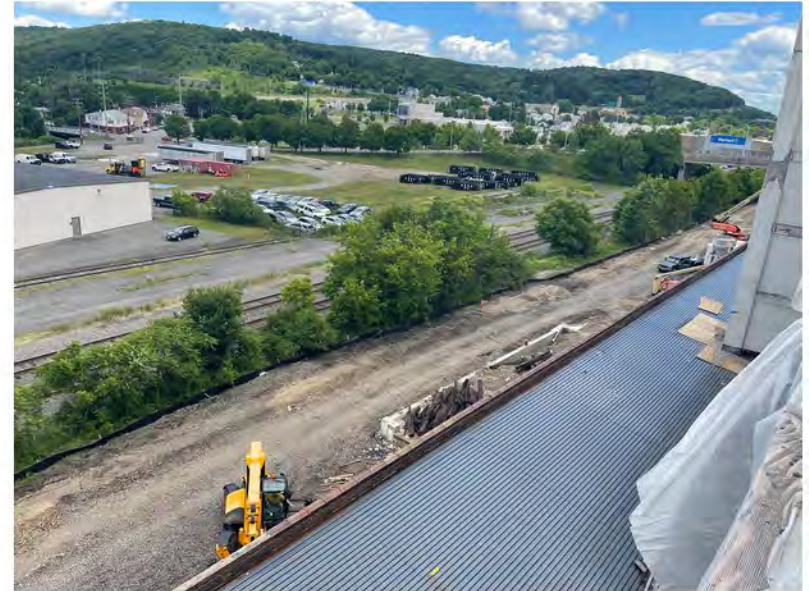
2022-06-10 13:51 42.1159639 N , 75.9527139 W Aerial view of work along Avenue C, looking northeast.
