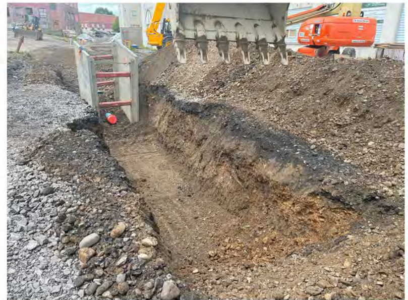
2022-06-09 13:39 42.1155139 N , 75.9519972 W Installation of water line along Helen Drive
