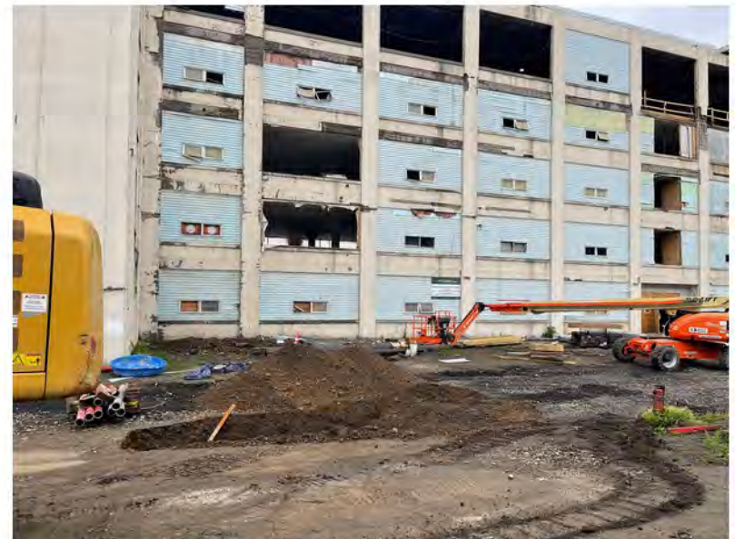
2022-06-09 08:35 42.1154222 N , 75.9523861 W Status of storm sewer work along Helen Drive
