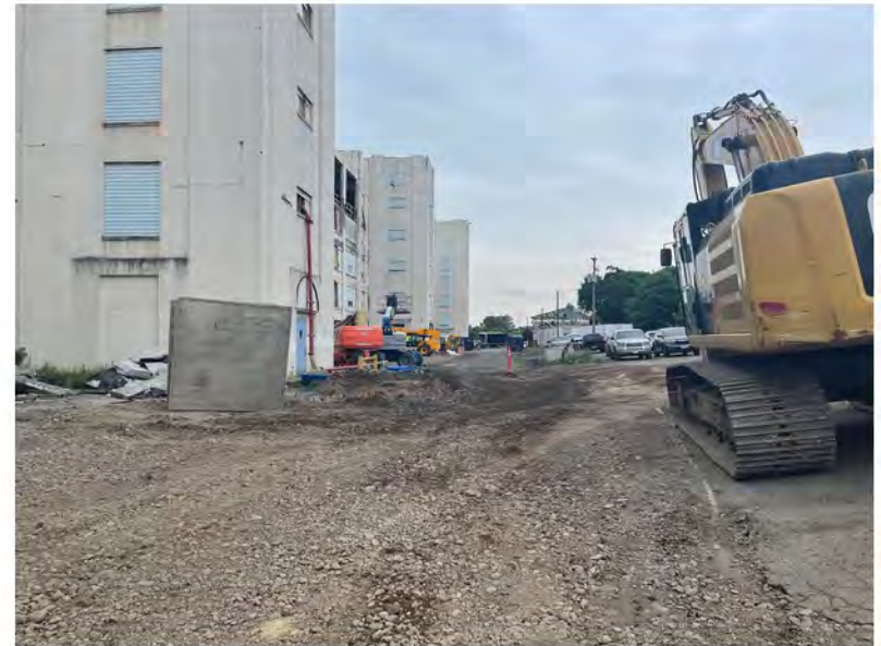
2022-06-07 13:57 42.1154278 N , 75.9527056 W Work Zone #1, looking east
