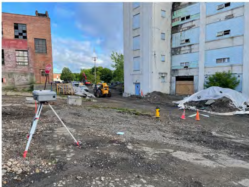
2022-06-08 07:54 42.1156194 N , 75.9526889 W Work Zone #1, looking northwest
