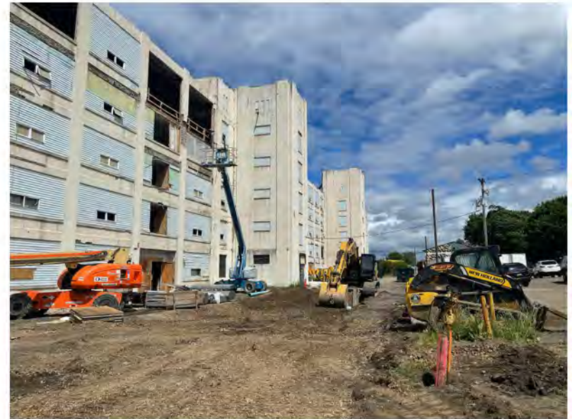
2022-06-09 15:10 42.1155250 N , 75.9522694 W Work progress along Helen Drive, looking east
