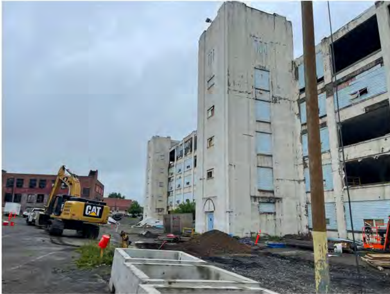
2022-06-09 08:35 42.1153833 N , 75.9520722 W Work Zone #1 (Helen Drive), looking west
