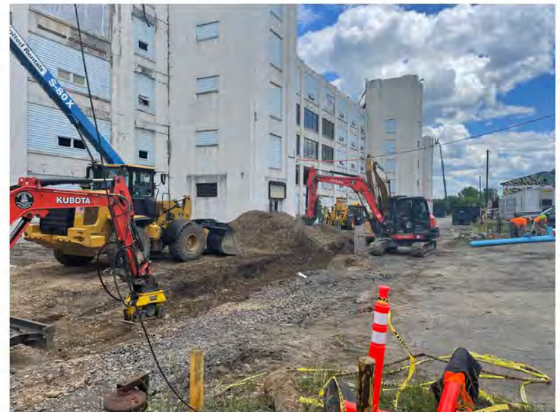
2022-06-10 12:59 42.1154417 N , 75.9521028 W Installation of water line along Helen Drive, looking east
