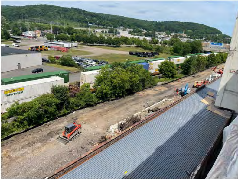
2022-06-06 14:47 42.1159333 N , 75.9527278 W Aerial view of work along Avenue C, looking northeast
