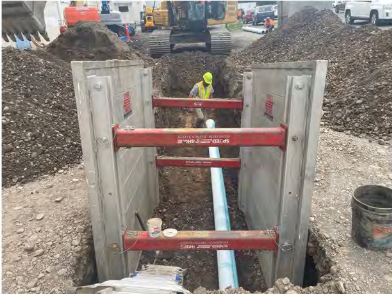
2022-06-07 11:29 42.1155667 N , 75.9525222 W Installation of water line along Helen Drive
