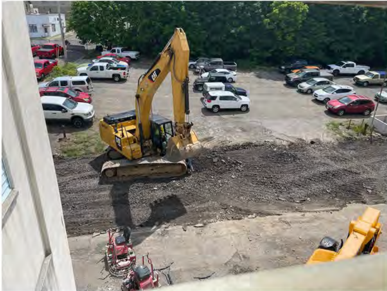
2022-06-06 14:43 42.1151083 N , 75.9525444 W Aerial view of work along Helen Drive, looking south
