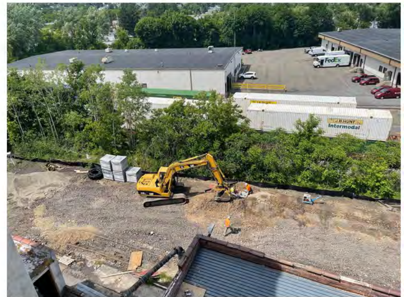
2022-06-06 14:47 42.1159056 N , 75.9527139 W Aerial view of work along Avenue C, looking northwest
