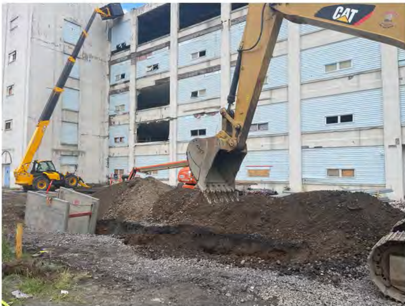
2022-06-09 13:39 42.1147528 N , 75.9518889 W Installation of water line along Helen Drive, looking east
