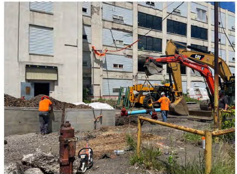
2022-06-10 14:11 42.1154056 N , 75.9520194 W Installation of water line along Helen Drive
