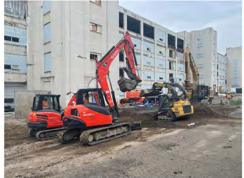
2022-06-07 13:21 42.1155194 N , 75.9526139 W Installation of water line along Helen Drive
