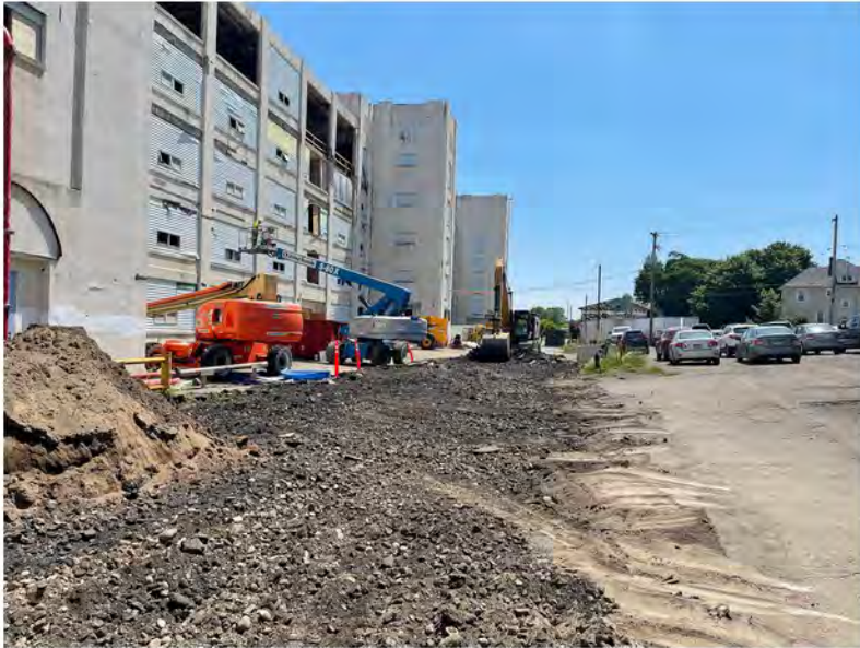
2022-06-06 11:43 42.1156194 N , 75.9524778 W Work Zone #1 (Helen Drive), looking east
