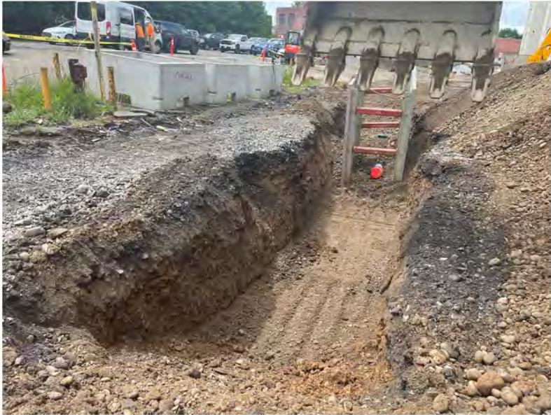
2022-06-09 13:40 42.1155083 N , 75.9520028 W Installation of water line along Helen Drive
