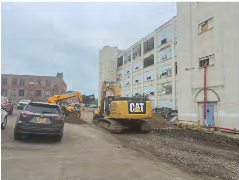
2022-06-07 10:43 42.1154417 N , 75.9522639 W Removal of asphalt along Helen Drive, looking west
