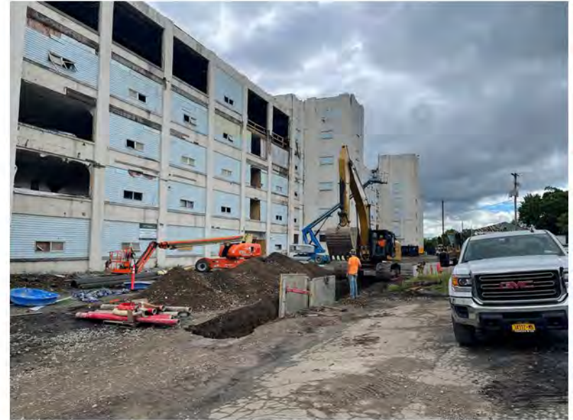
2022-06-09 10:43 42.1154750 N , 75.9525222 W Installation of water line along Helen Drive, looking east
