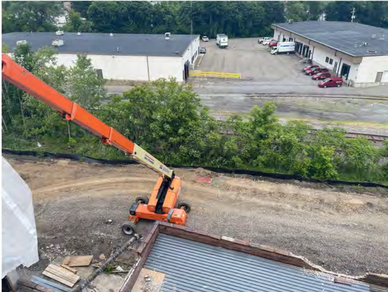
2022-06-10 13:51 42.1159528 N , 75.9527194 W Aerial view of work along Avenue C, looking north.
