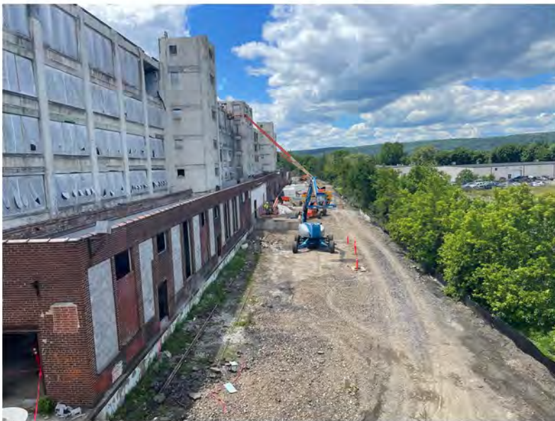
2022-06-10 13:57 42.1155556 N , 75.9503333 W Aerial view of work along Avenue C, looking west.
