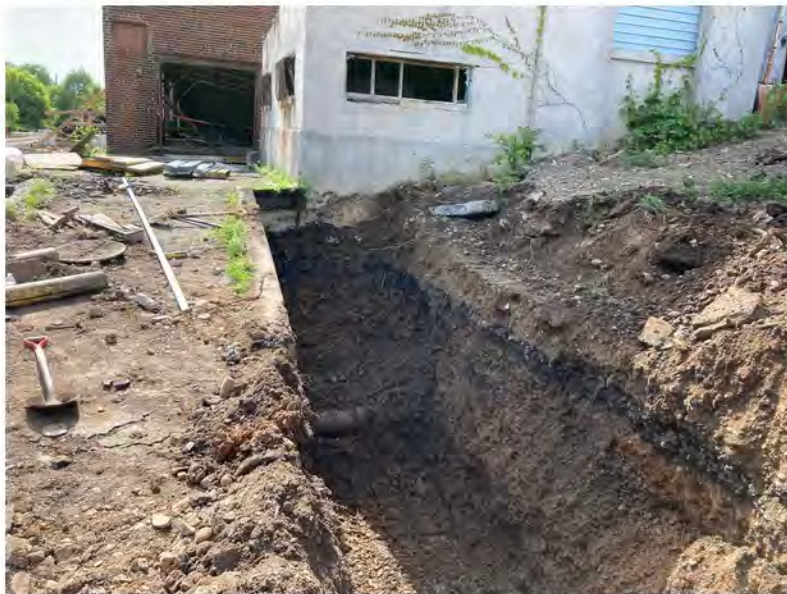
2022-06-14 09:51 42.1155778 N , 75.9527361 W Avenue C at northwestern corner of building, looking east
