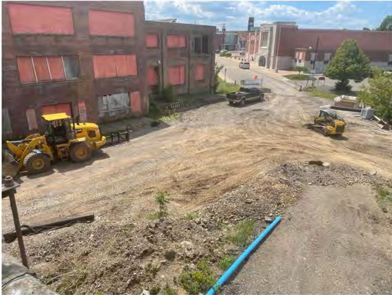
2022-06-17 14:03 42.1159083 N , 75.9529944 W Aerial view of western end of site, looking west
