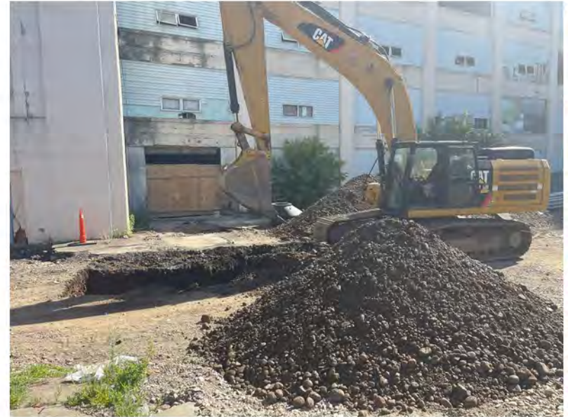
2022-06-15 09:35 42.1147639 N , 75.9525389 W Excavation on Helen Drive, near Avenue B
