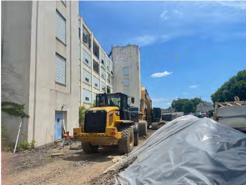
2022-06-15 12:58 42.1156889 N , 75.9531389 W Western end of site along Helen Drive, looking east
