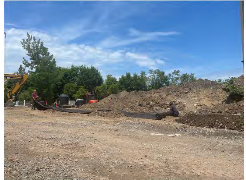
2022-06-15 13:09 42.1157583 N , 75.9529944 W Western end of site along Avenue C, looking northwest
