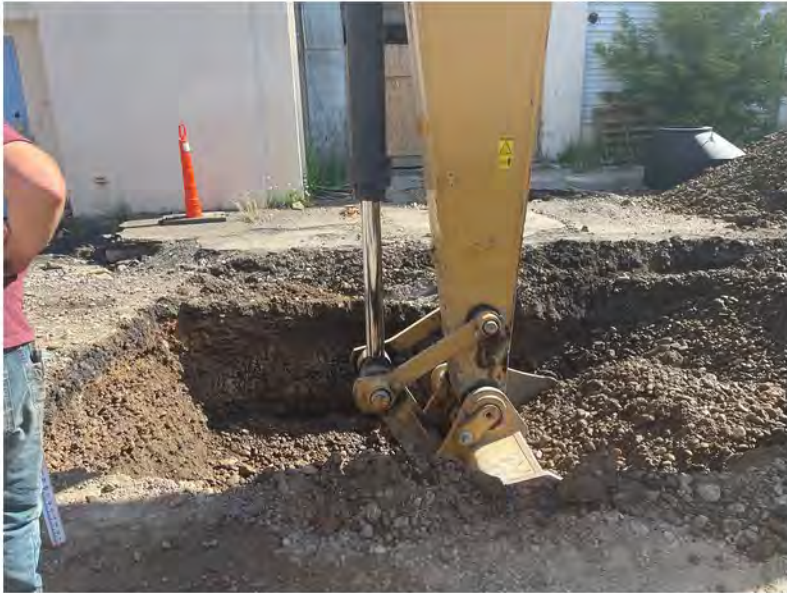
2022-06-15 09:29 42.1147028 N , 75.9529889 W Excavation on Helen Drive, near Avenue B
