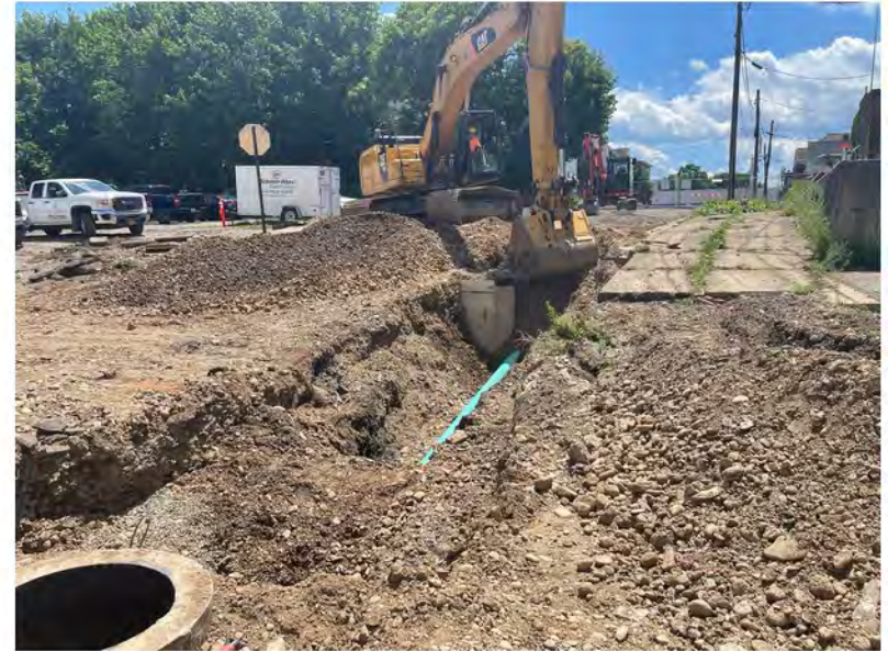
2022-06-17 13:42 42.1154778 N , 75.9525306 W Storm sewer excavation along Avenue B, looking south
