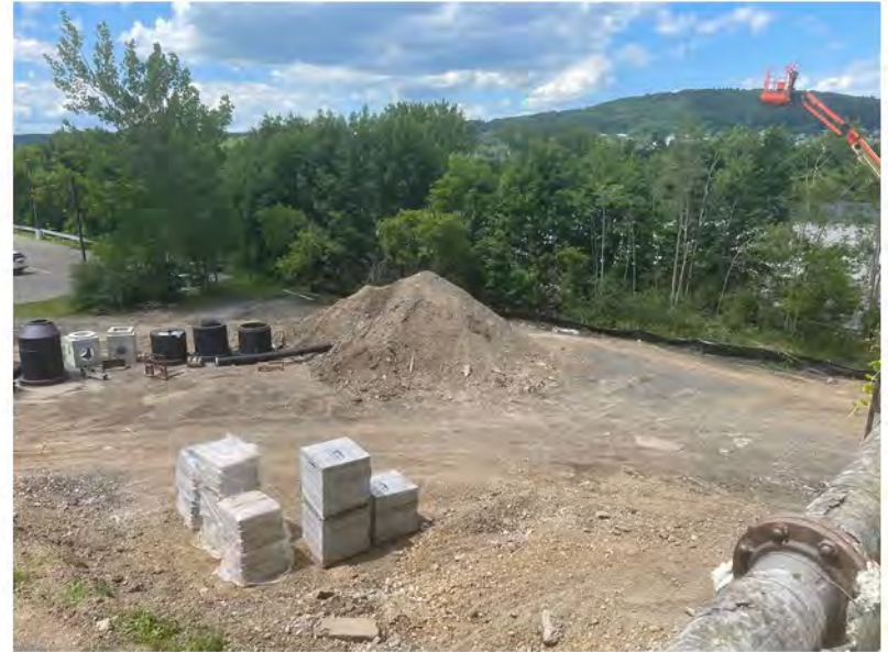
2022-06-17 14:03 42.1159083 N , 75.9530028 W Aerial view of western end of site, looking northwest
