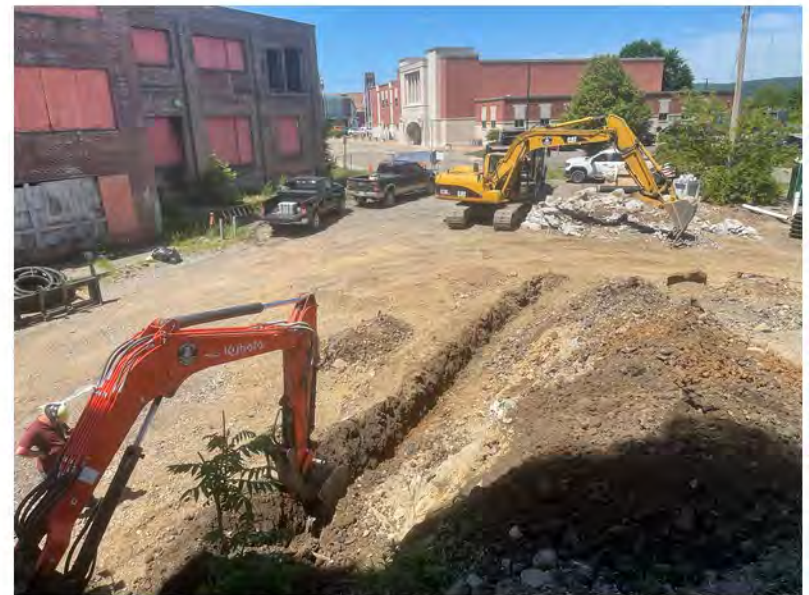
2022-06-15 11:44 42.1157222 N , 75.9539111 W Aerial view of western end of site, looking west
