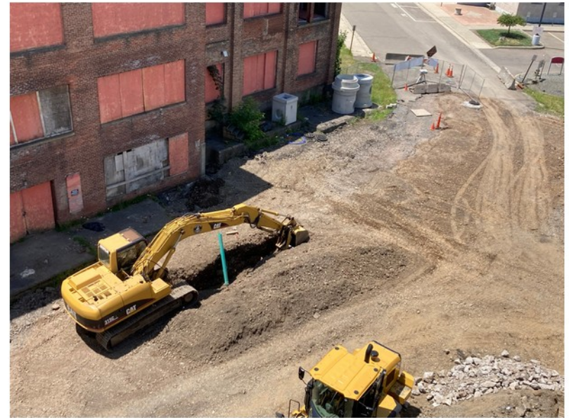
2022-06-24 13:02 42.1158750 N , 75.9530194 W Aerial view of west end of site, looking west
