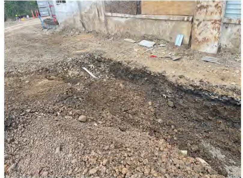
2022-06-30 13:34 42.1158861 N , 75.9530028 W Sewer line excavation on west end of site
