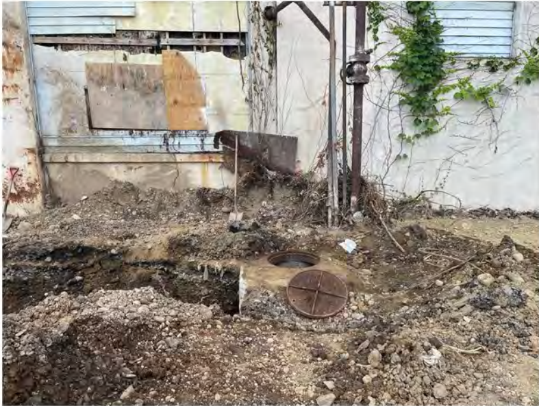
2022-07-01 09:12 42.1158250 N , 75.9530806 W Existing manhole in west end of site
