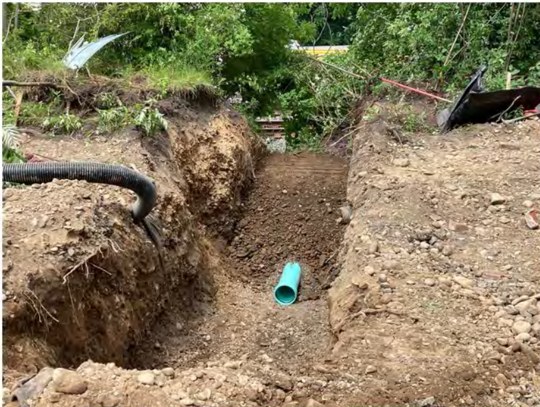
2022-06-29 14:06 42.1159833 N , 75.9529028 W Sewer line being installed
