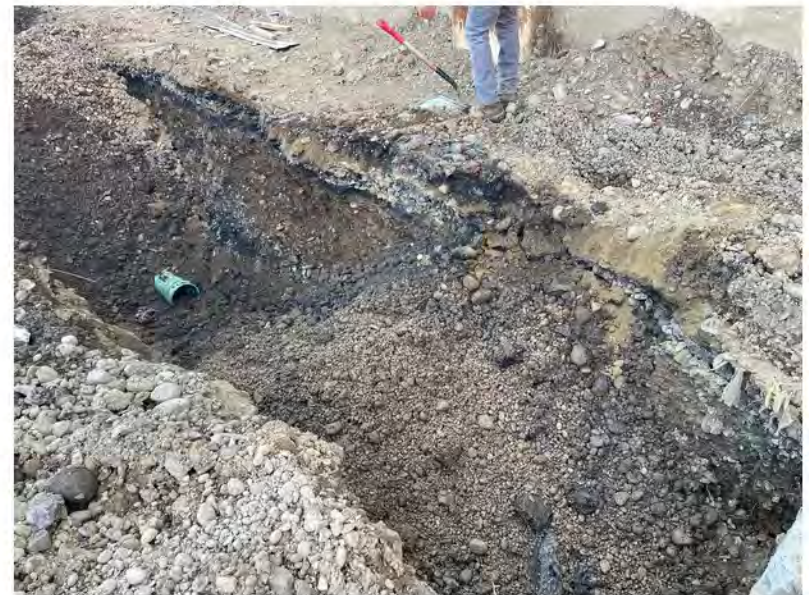
2022-07-01 08:29 42.1158750 N , 75.9530333 W Sewer line excavation on west end of site
