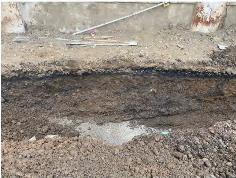
2022-06-30 13:34 42.1158833 N , 75.9530028 W Sewer line excavation on west end of site
