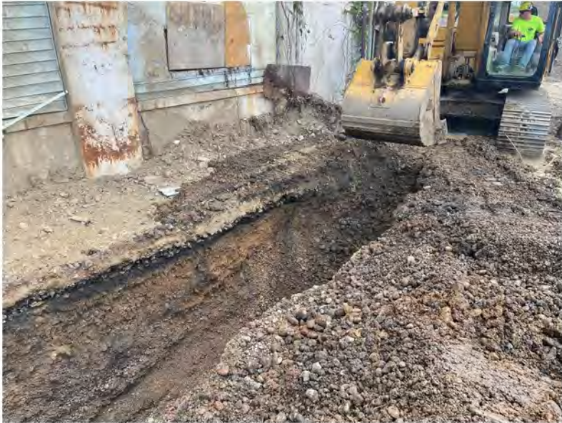
2022-06-30 13:34 42.1158778 N , 75.9530028 W Sewer line excavation on west end of site
