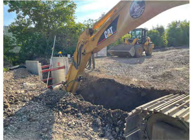
2022-06-30 07:57 42.1156694 N , 75.9539194 W Sewer line installation
