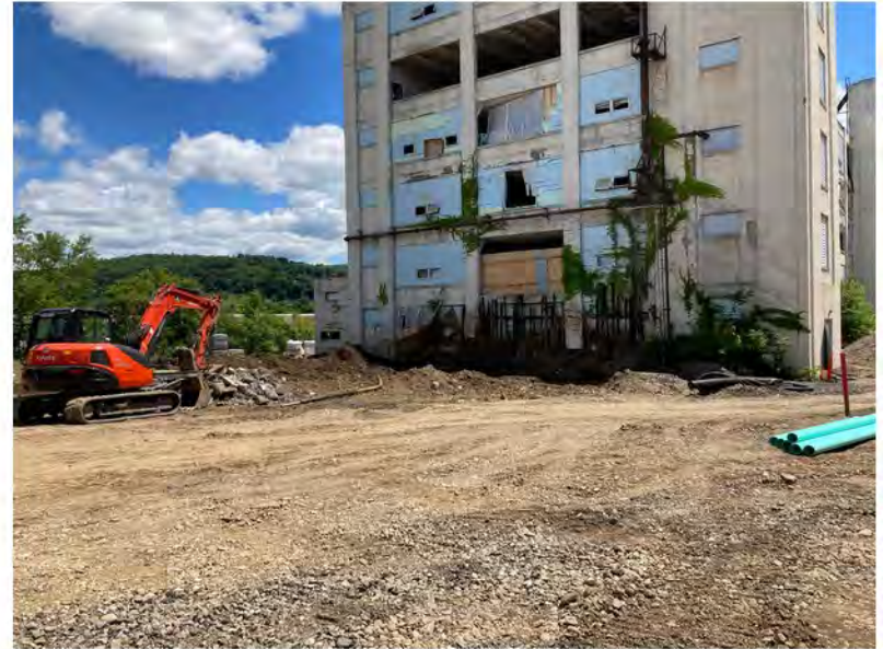
2022-06-28 12:12 42.1158167 N , 75.9533389 W Ramp at west end of building removed, looking east
