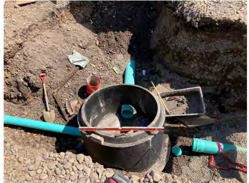
2022-07-07 10:31 42.1154583 N , 75.9533472 W Closeup of sewer work on Helen Drive
