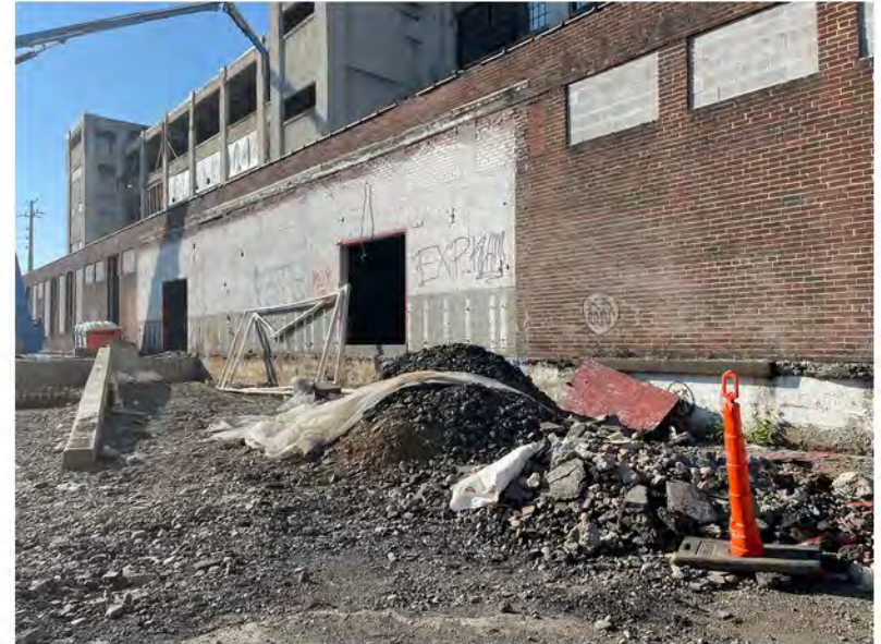
2022-07-11 08:11 42.1157694 N , 75.9512778 W Staged railroad bedding prior to load-out
