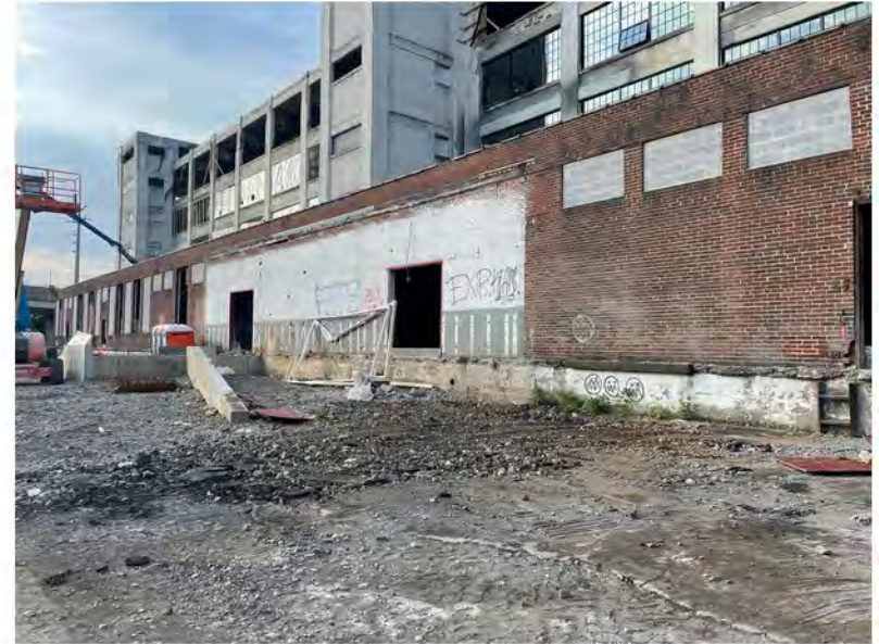
2022-07-12 07:34 42.1158056 N , 75.9512944 W Area of staged railroad bedding after load-out
