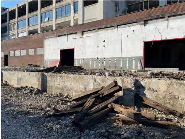
2022-07-11 08:09 42.1160250 N , 75.9523861 W Staged railroad ties prior to load-out
