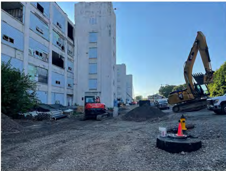
2022-07-11 07:42 42.1156778 N , 75.9529194 W Helen Drive near Avenue B, looking east
