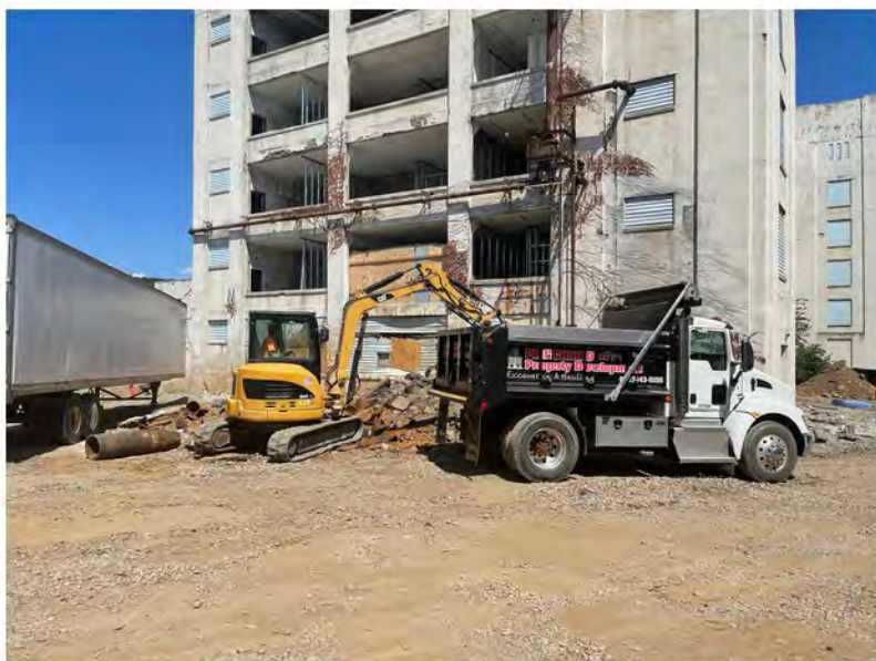
2022-07-22 15:05 42.1158111 N , 75.9532389 W Removing staged sewer pipe from west end of building
