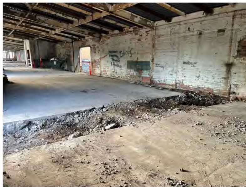
2022-07-21 08:04 42.1157500 N , 75.9513556 W Annex sewer line excavation
