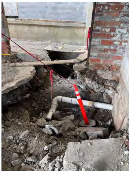
2022-07-21 07:44 42.1151722 N , 75.9513083 W Annex sewer line excavation
