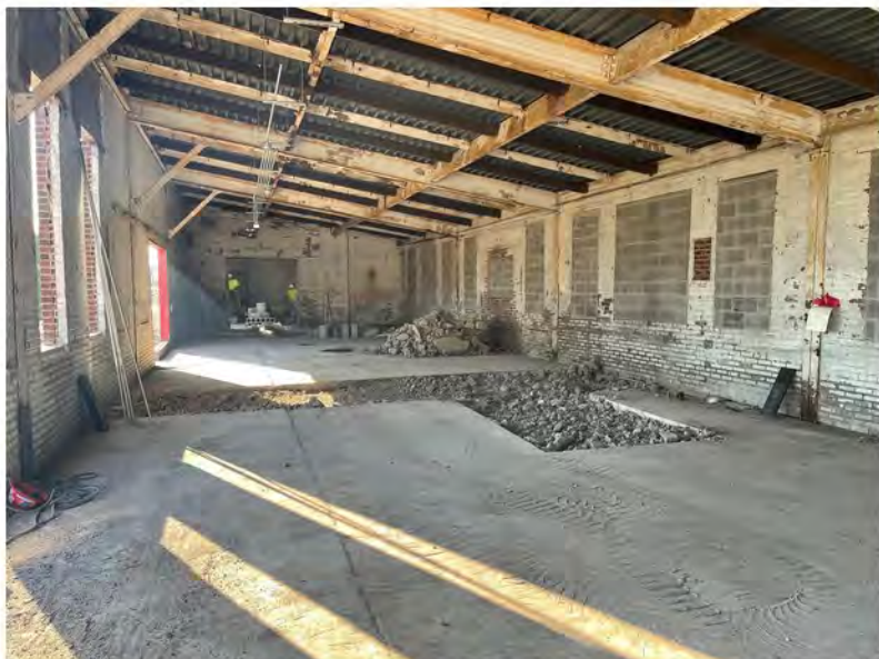
2022-07-22 07:48 42.1163889 N , 75.9530639 W Annex sewer line excavation
