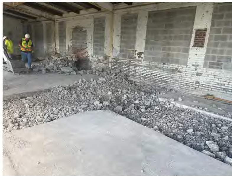
2022-07-21 13:02 42.1161417 N , 75.9525389 W Annex sewer line excavation
