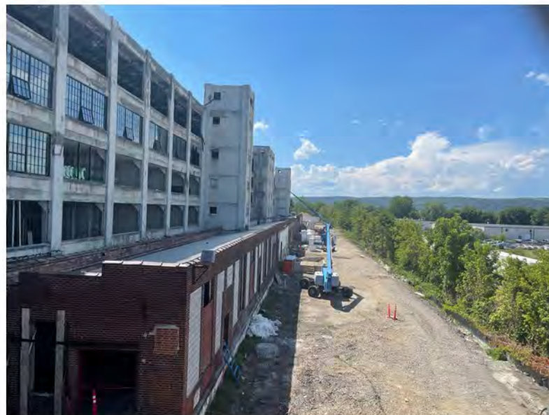
2022-07-22 15:10 42.1155056 N , 75.9504389 W Aerial view of Avenue C, looking west
