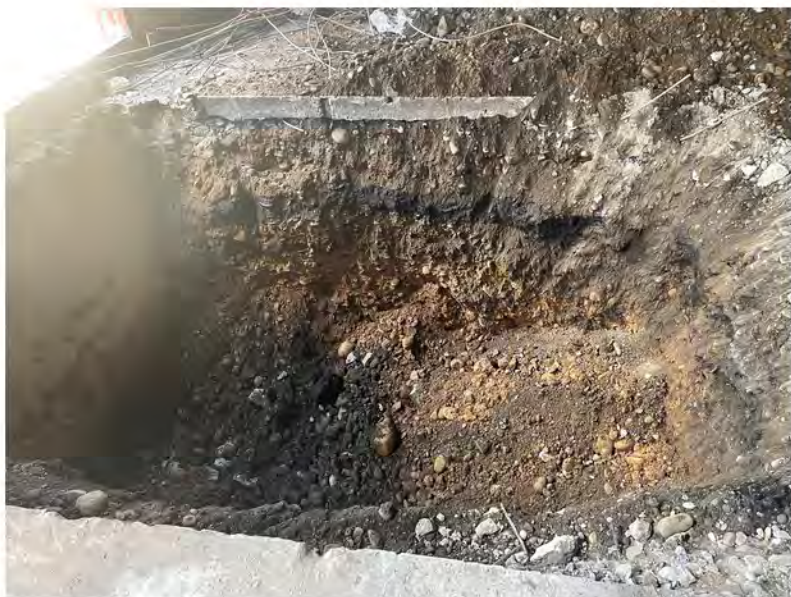
2022-07-21 13:06 42.1152944 N , 75.9504917 W Annex sewer line excavation
