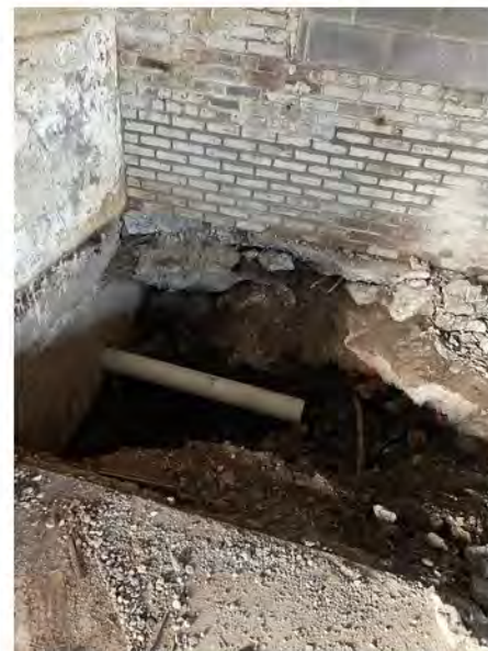
2022-07-21 08:02 42.1159750 N , 75.9523250 W Annex sewer line excavation
