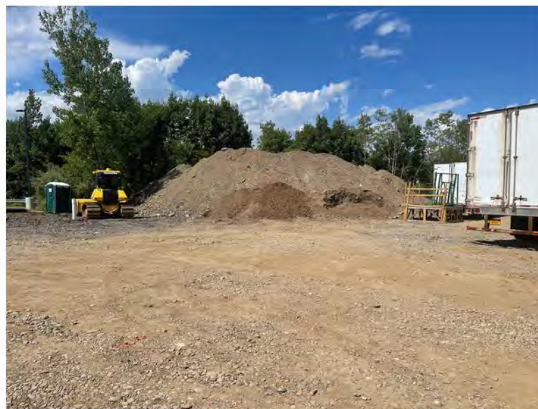
2022-07-22 15:05 42.1158056 N , 75.9532389 W West end of site, looking northwest
