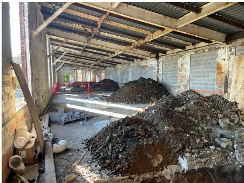
2022-07-22 07:50 42.1155972 N , 75.9509972 W Annex sewer line excavation
