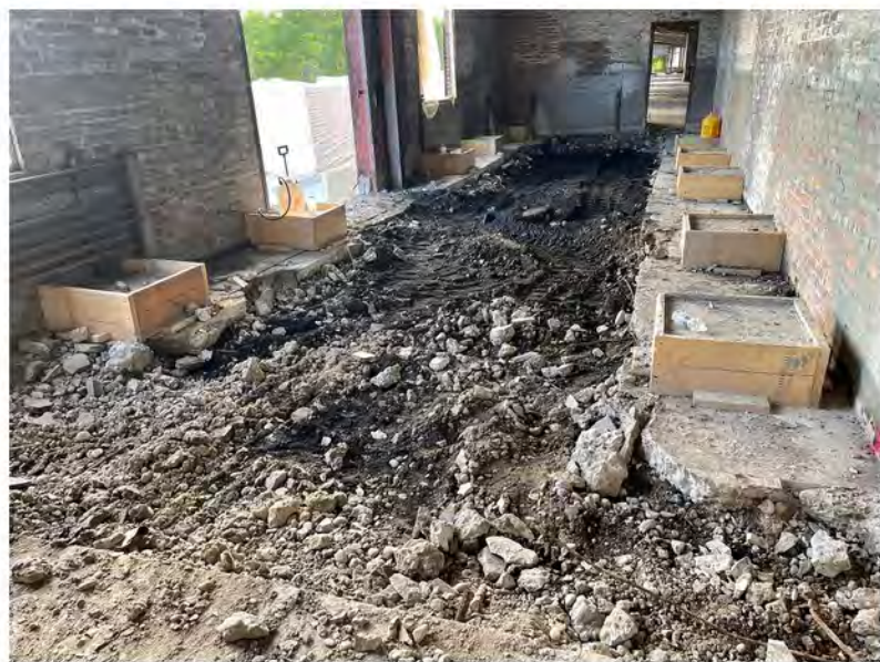
2022-07-21 08:03 42.1158722 N , 75.9517056 W Annex sewer line excavation
