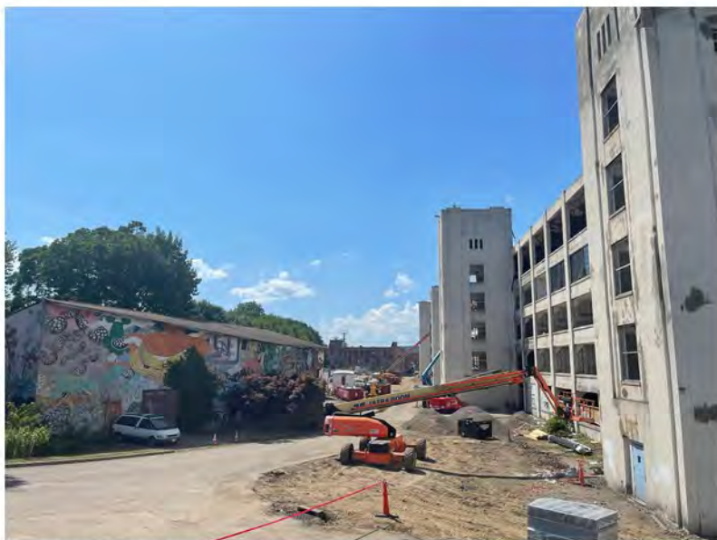
2022-07-22 15:11 42.1150694 N , 75.9503167 W Eastern end of site, looking west down Helen Drive
