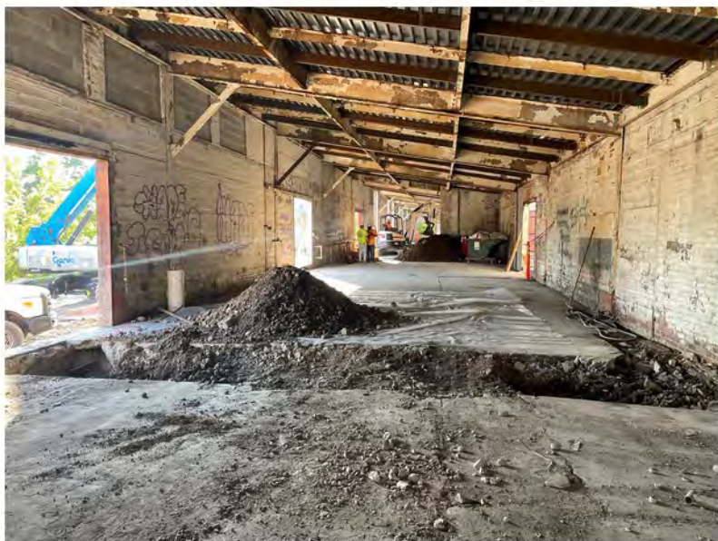
2022-07-22 07:50 42.1158056 N , 75.9514528 W Annex sewer line excavation
