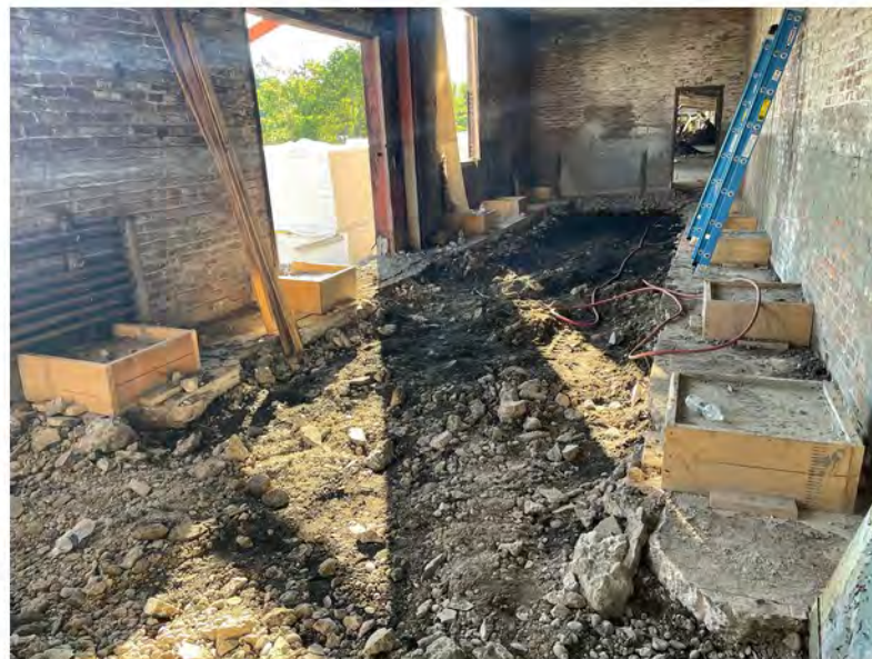
2022-07-22 07:49 42.1158611 N , 75.9517278 W Annex sewer line excavation
