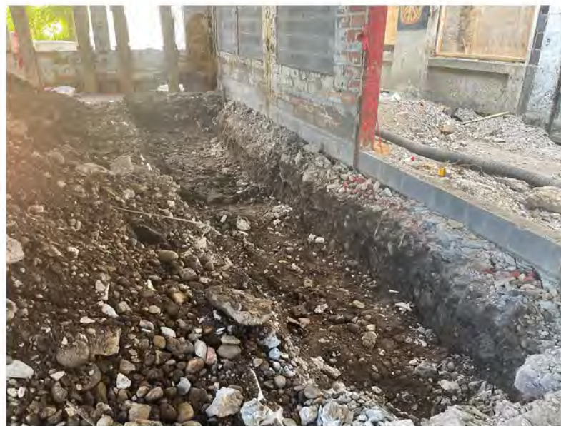
2022-07-21 13:07 42.1153333 N , 75.9508667 W Annex sewer line excavation
