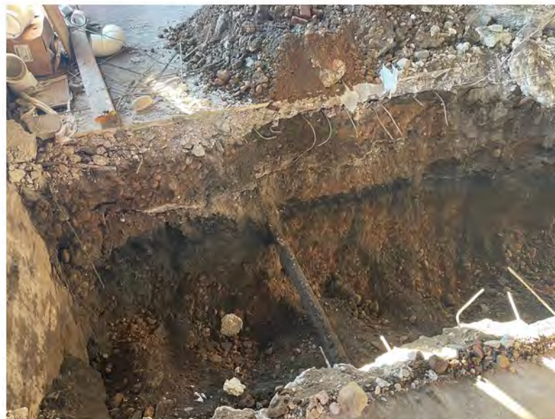
2022-07-22 07:50 42.1156056 N , 75.9510028 W Annex sewer line excavation
