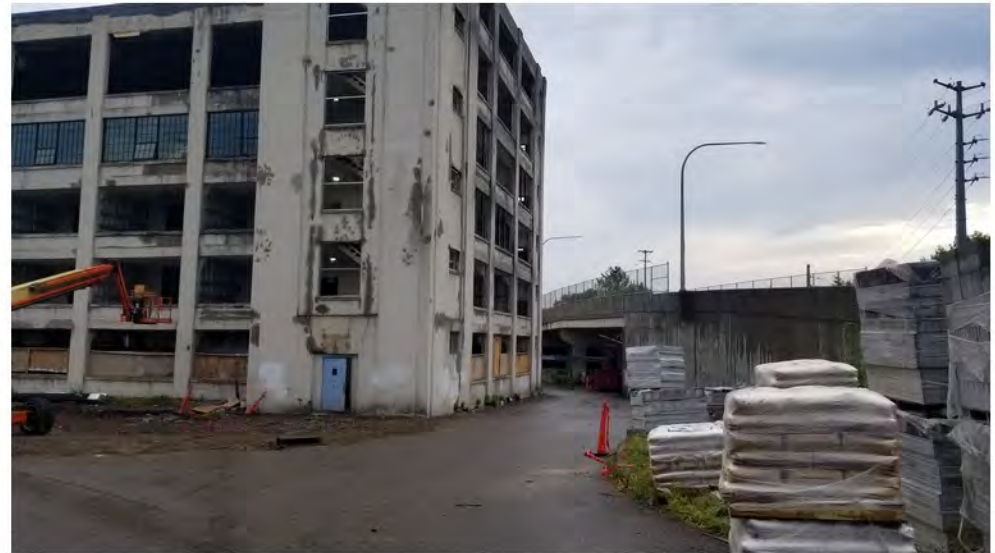
2022-07-25 07:27 42.1145246 N , 75.9504165 W Eastern portion of site, looking north
