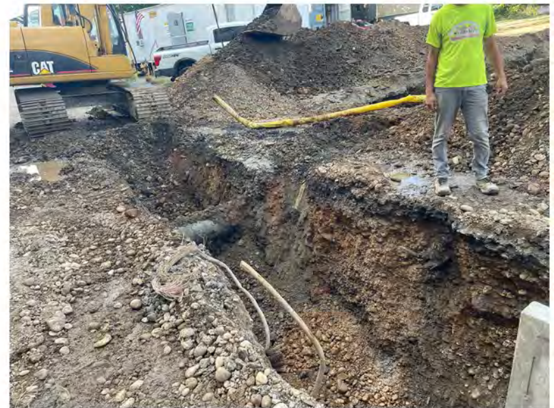
2022-07-26 07:33 42.1154250 N , 75.9517056 W Trenching along Helen Drive, looking east
