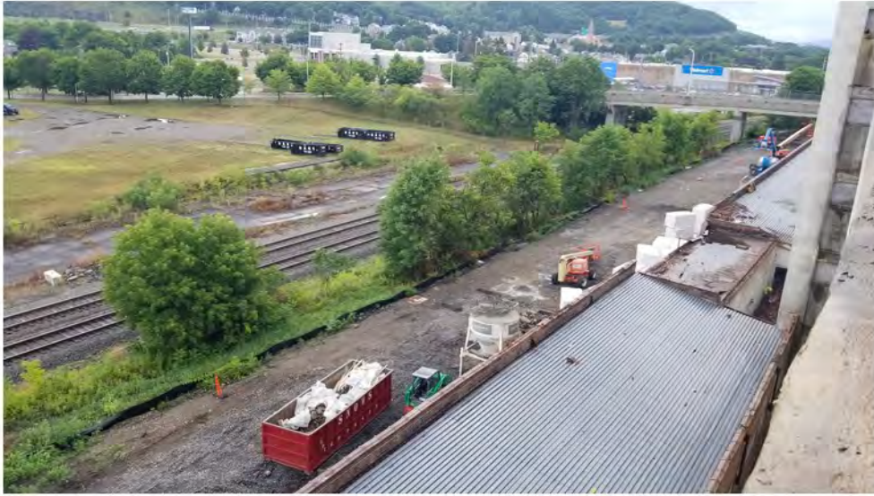
2022-07-25 08:30 42.1182078 N , 75.9504950 W Aerial view of Avenue C, looking northeast
