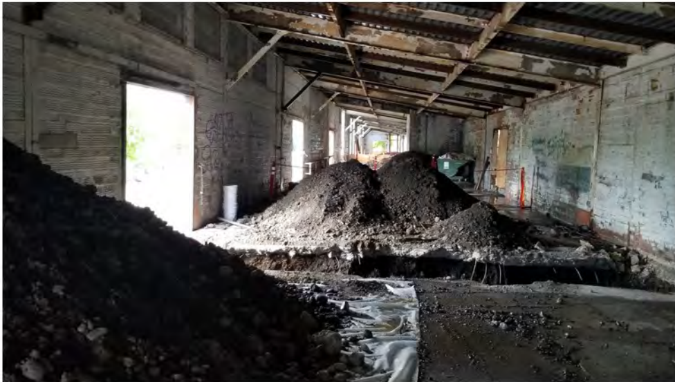
2022-07-25 08:52 42.1149005 N , 75.9512158 W Interior trenches in annex for storm sewer
