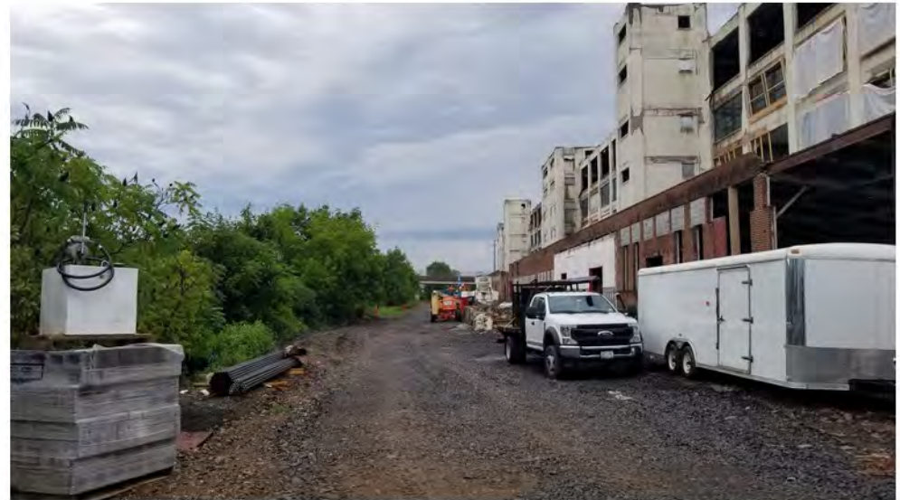
2022-07-25 07:34 42.1166382 N , 75.9527050 W Avenue C, looking east
