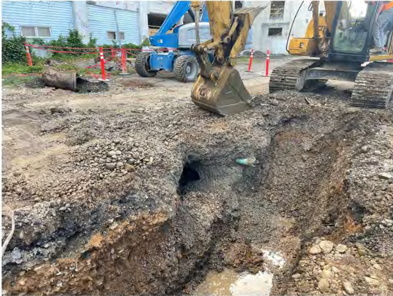
2022-07-26 07:54 42.1149444 N , 75.9518444 W Old sewer pipe removed
