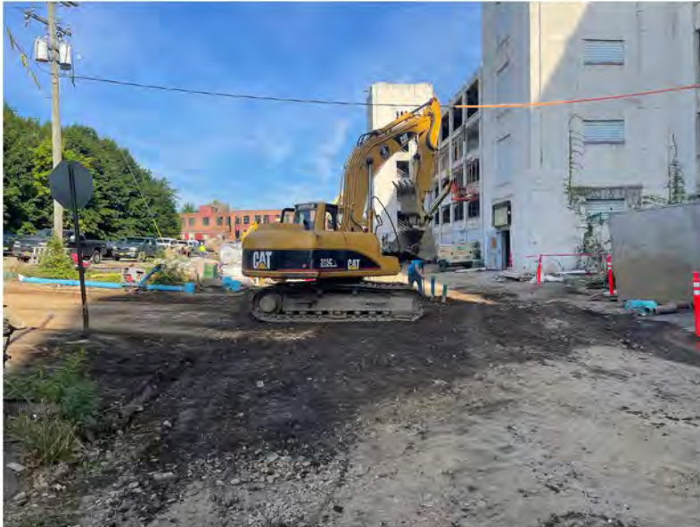
2022-07-27 08:33 42.1152333 N , 75.9514250 W Trenching along Helen Drive, looking west
