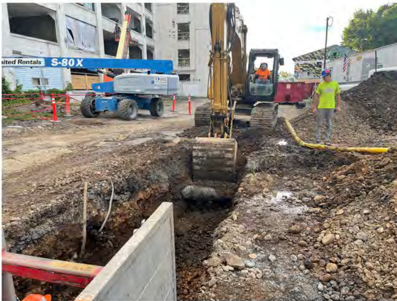
2022-07-26 07:33 42.1153833 N , 75.9517444 W Trenching along Helen Drive, looking east
