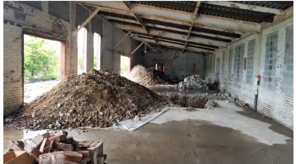
2022-07-25 08:55 42.1104310 N , 75.9588428 W Interior trenches in annex for storm sewer
