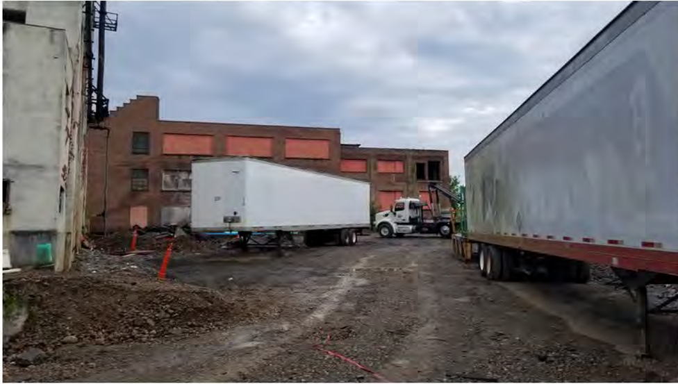
2022-07-25 07:34 42.1166382 N , 75.9527050 W Western portion of site, looking south
