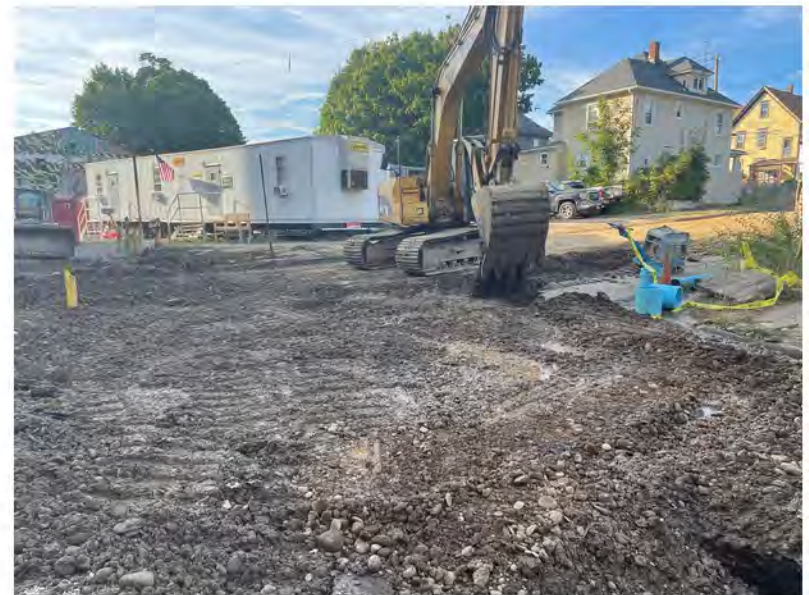
2022-07-27 08:01 42.1147944 N , 75.9518806 W Trenching along Helen Drive, looking southeast
