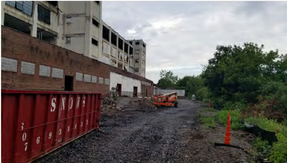
2022-07-25 07:33 42.1166382 N , 75.9527050 W Western end of Avenue C, looking west
