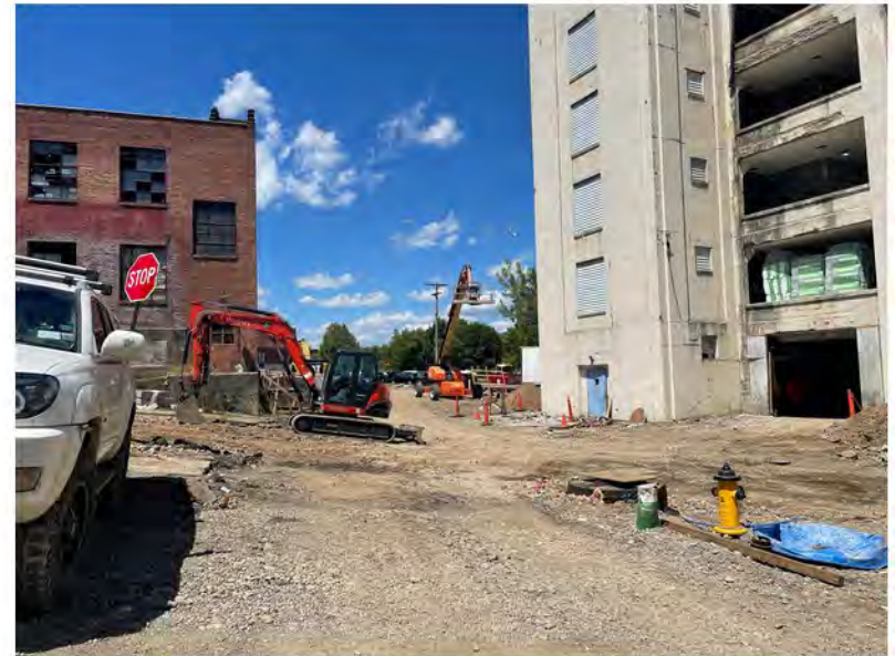
2022-07-29 12:54 42.1155361 N , 75.9527194 W Backfilling excavation on Avenue B at Helen Drive
