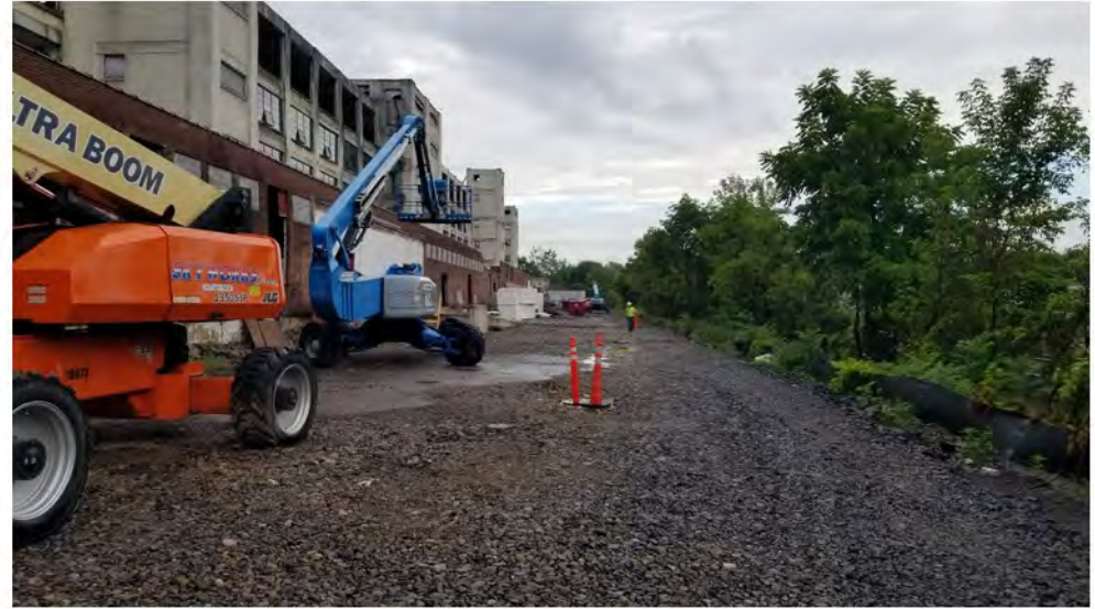
2022-07-25 07:31 42.1145150 N , 75.9507877 W Eastern end of Avenue C, looking west
