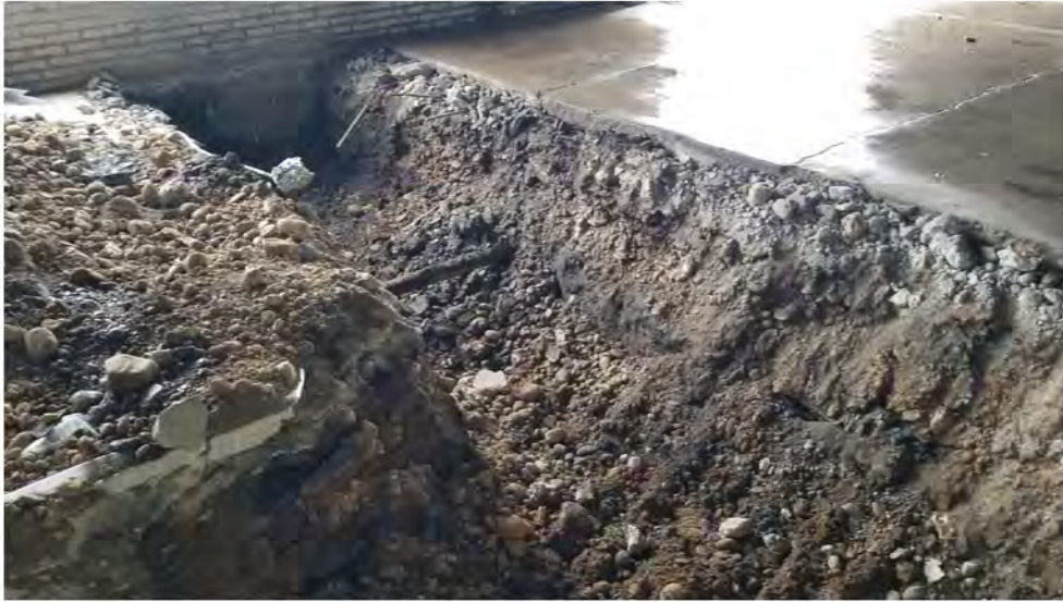
2022-07-25 08:55 42.1104310 N , 75.9588428 W Typical interior trench in annex for storm sewer
