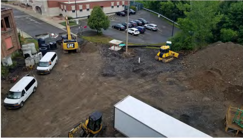
2022-07-25 08:28 42.1157613 N , 75.9543187 W Aerial view of western portion of site, looking west
