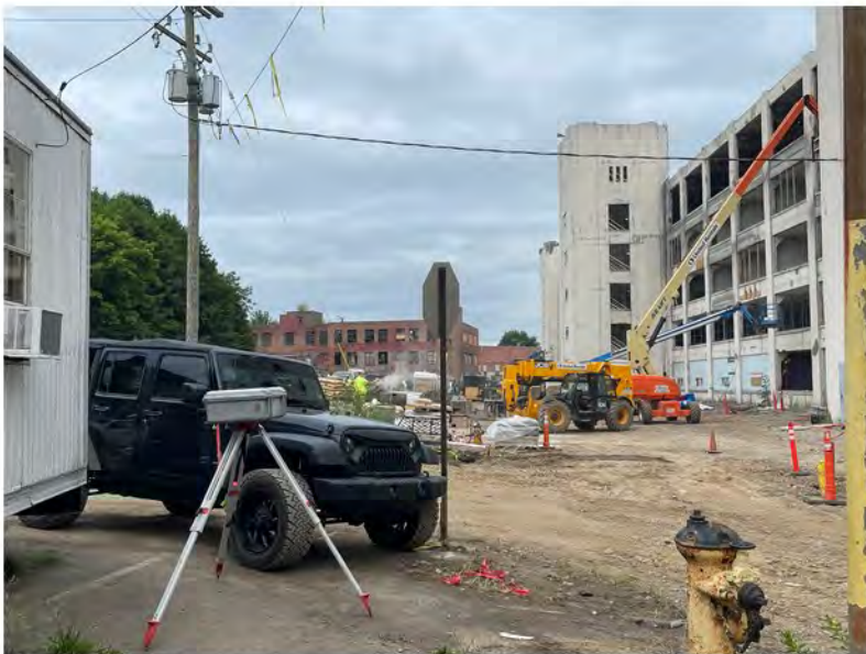
2022-08-01 07:49 42.1153556 N , 75.9514167 W Work Zone #1, Helen Drive at Avenue A, looking west
