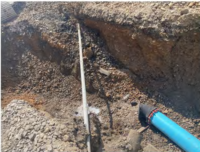
2022-08-02 11:07 42.1153806 N , 75.9515833 W Excavation along Helen Drive
