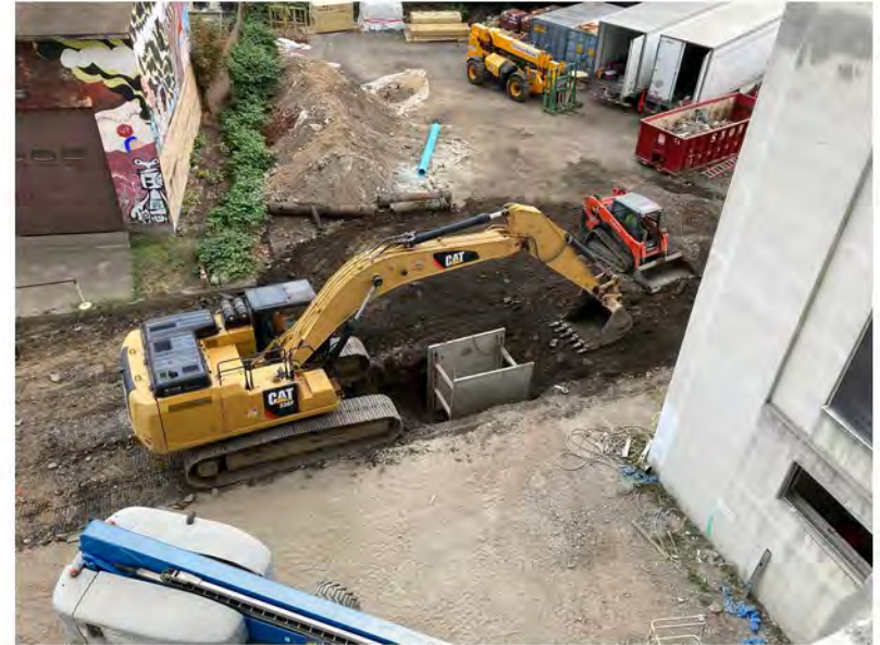
2022-08-04 13:24 42.1149139 N , 75.9508528 W Aerial view of excavations on Helen Drive, looking south
