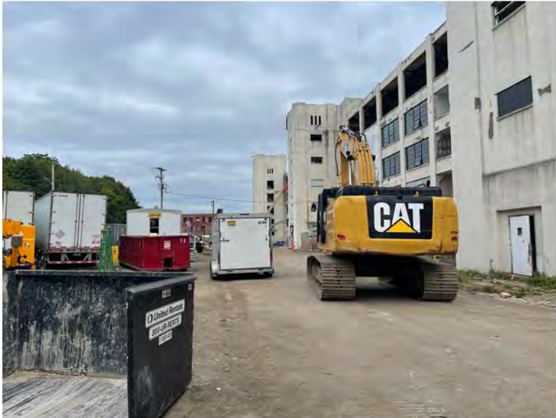
2022-08-01 07:49 42.1148722 N , 75.9514306 W Work Zone #1 (southern excavations), looking west down Helen Drive
