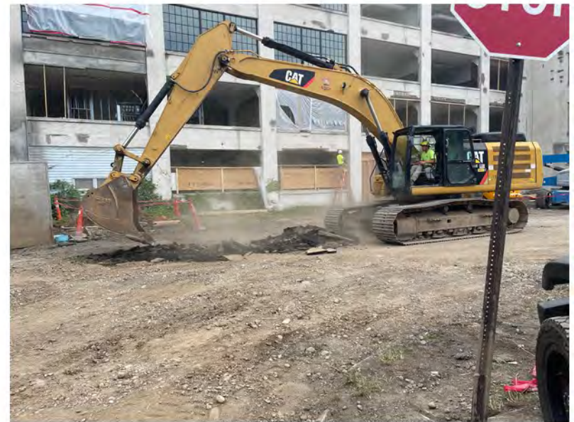
2022-08-01 07:51 42.1153306 N , 75.9515833 W Excavation on Helen Drive near Avenue A intersection
