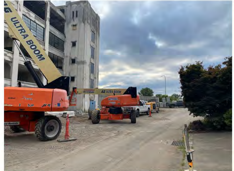
2022-08-01 07:49 42.1151889 N , 75.9509278 W Work Zone #1, looking east down Helen Drive
