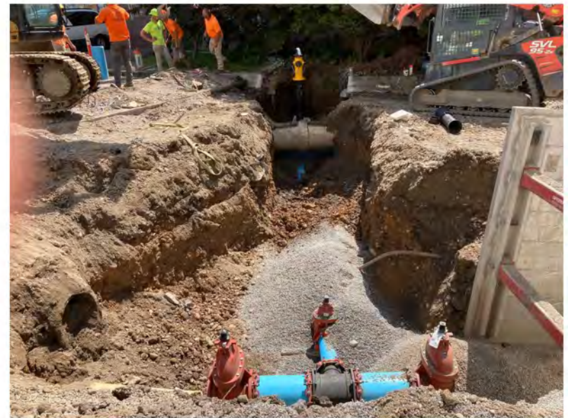
2022-08-05 14:28 42.1152611 N , 75.9507833 W Excavation on Helen Drive near eastern end of building
