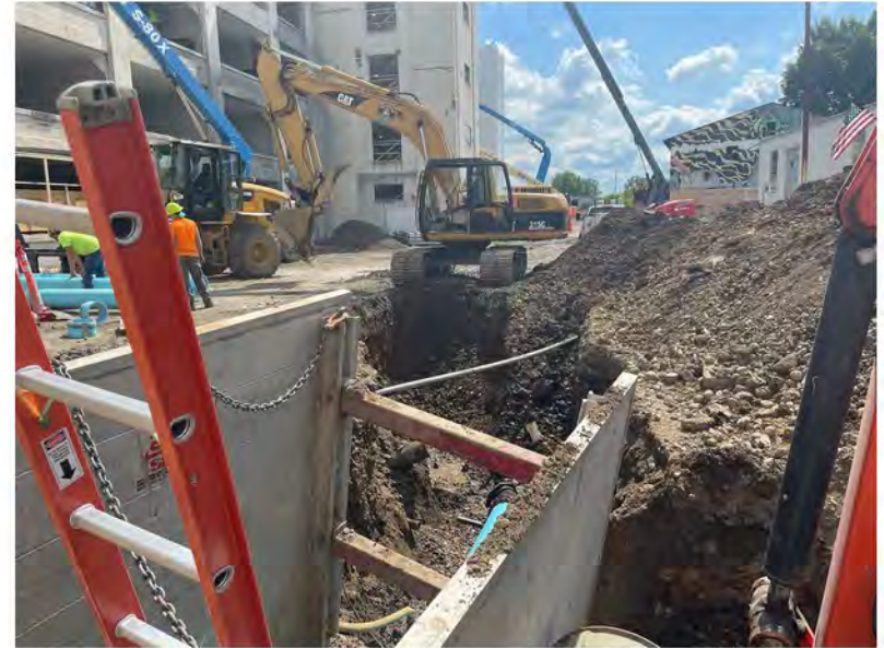
2022-08-02 11:06 42.1153444 N , 75.9516361 W Excavation along Helen Drive
