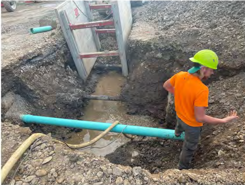
2022-08-02 07:32 42.1153750 N , 75.9516444 W Excavation along Helen Drive
