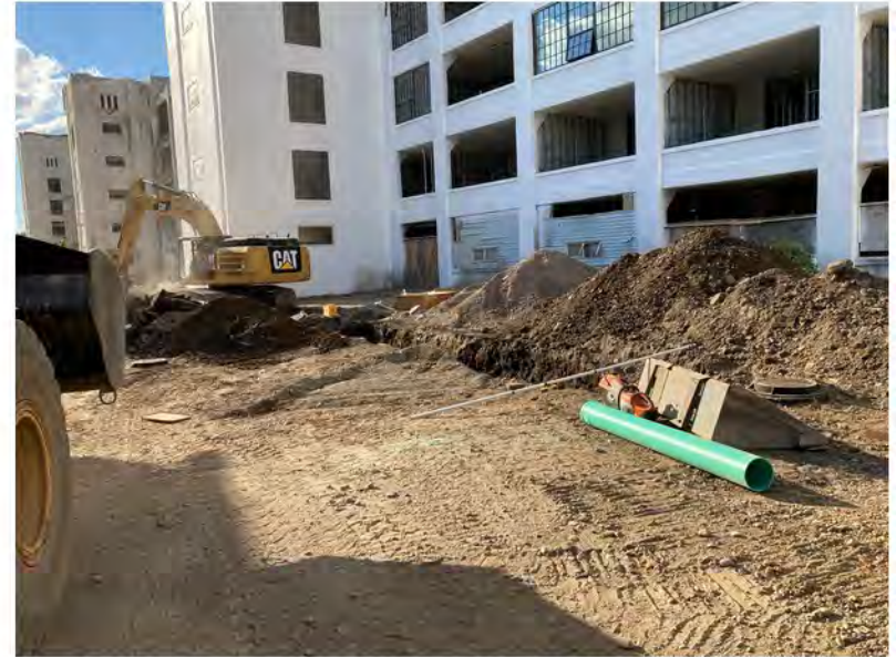
2022-08-11 18:03 42.1152694 N , 75.9506917 W Work Zone #1, Helen Drive near Avenue A, looking west
