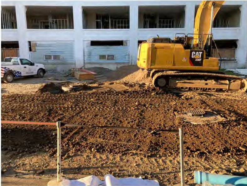
2022-08-10 19:15 42.1152694 N , 75.9509111 W Work Zone #1 (southern excavations), Helen Drive near Avenue A
