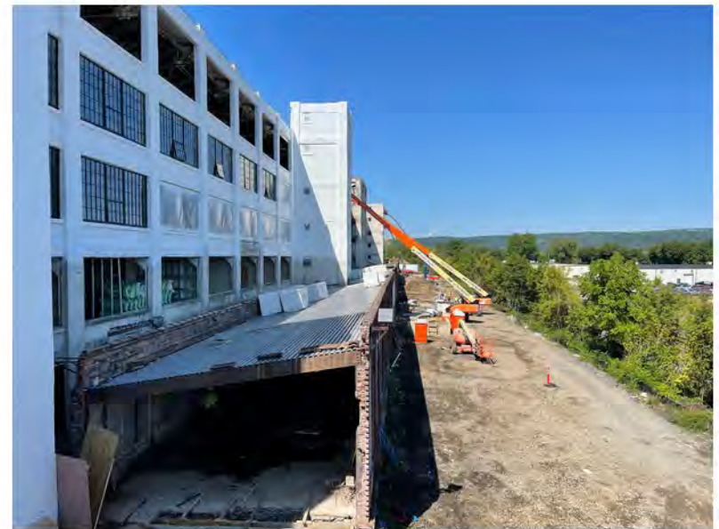
2022-08-19 11:22 42.1155194 N , 75.9502861 W Aerial view of Work Zone #2 (Avenue C)
