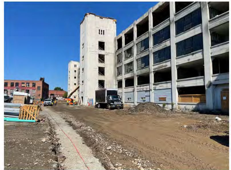
2022-08-19 10:53 42.1154361 N , 75.9518583 W Grading/leveling activities along Helen Drive, looking west
