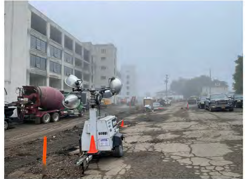
2022-08-19 07:45 42.1155389 N , 75.9525972 W Work Zone #1, grading/leveling activities along Helen Drive, looking east
