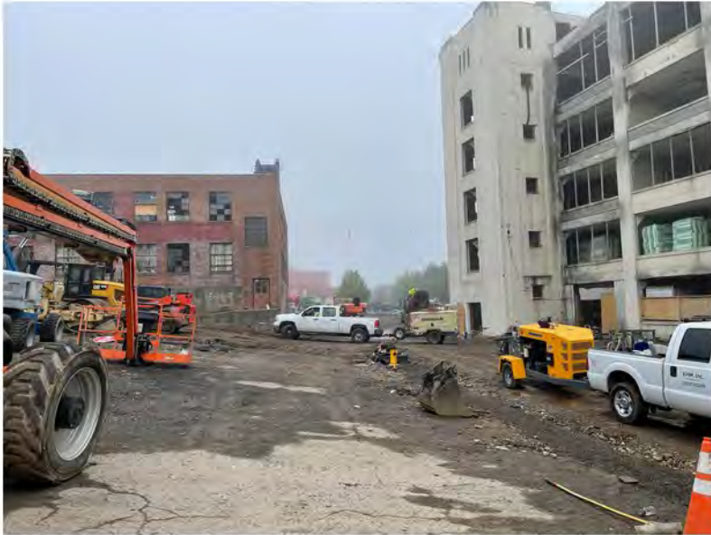
2022-08-19 07:45 42.1155194 N , 75.9525833 W Work Zone #1, grading/leveling activities along Helen Drive, looking west
