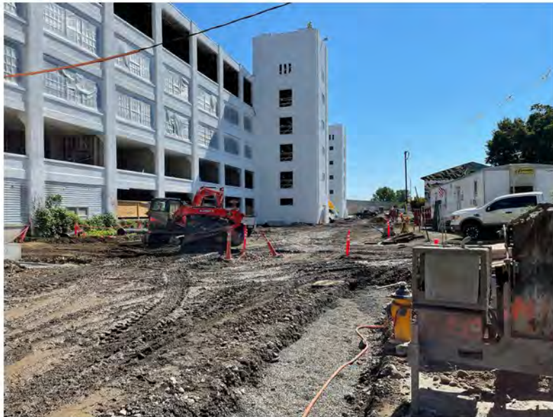
2022-08-19 10:53 42.1157639 N , 75.9516528 W Grading/leveling activities along Helen Drive, looking east
