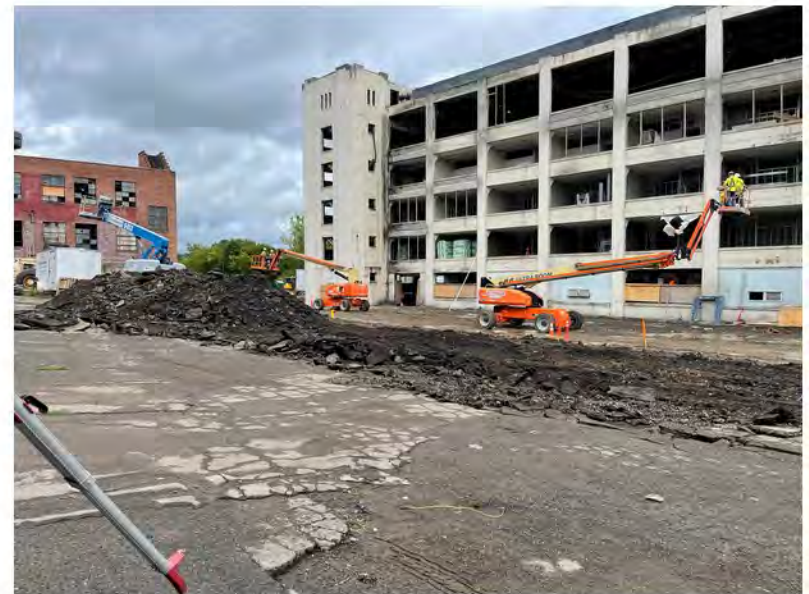
2022-08-22 10:50 42.1153861 N , 75.9525306 W Removal of asphalt and curb work in southwestern parking lot (along Helen Drive)
