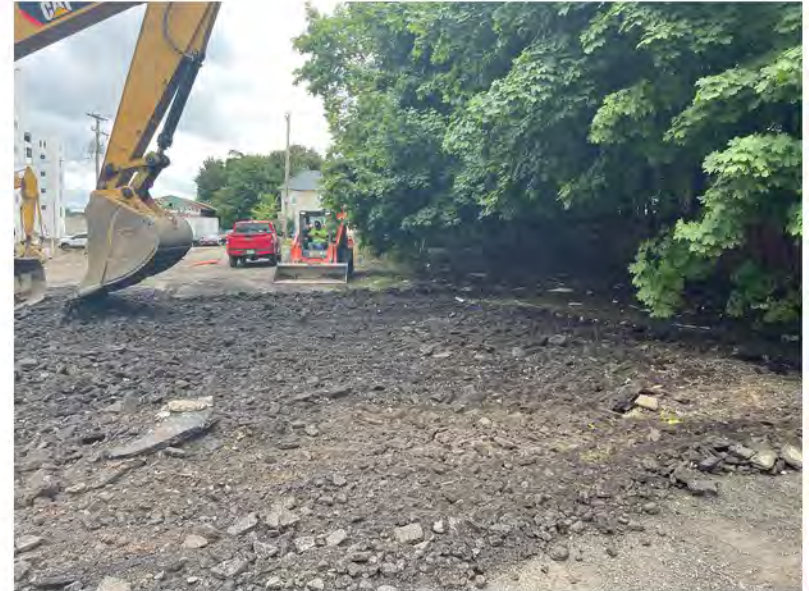
2022-08-22 11:20 42.1153528 N , 75.9524167 W Removal of asphalt in southwestern parking lot (south-central portion)
