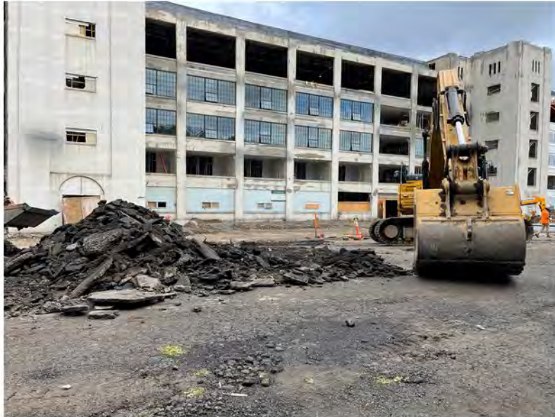
2022-08-22 10:50 42.1153944 N , 75.9525306 W Removal of asphalt in southwestern parking lot (north-central portion)
