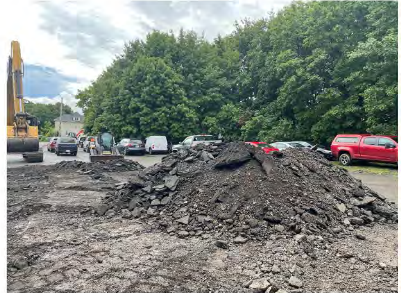
2022-08-22 09:15 42.1157111 N , 75.9527667 W Removal of asphalt in southwestern parking lot (southwestern portion)
