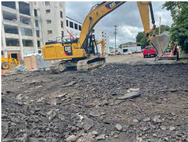
2022-08-22 11:20 42.1153667 N , 75.9524528 W Removal of asphalt in southwestern parking lot (central portion)
