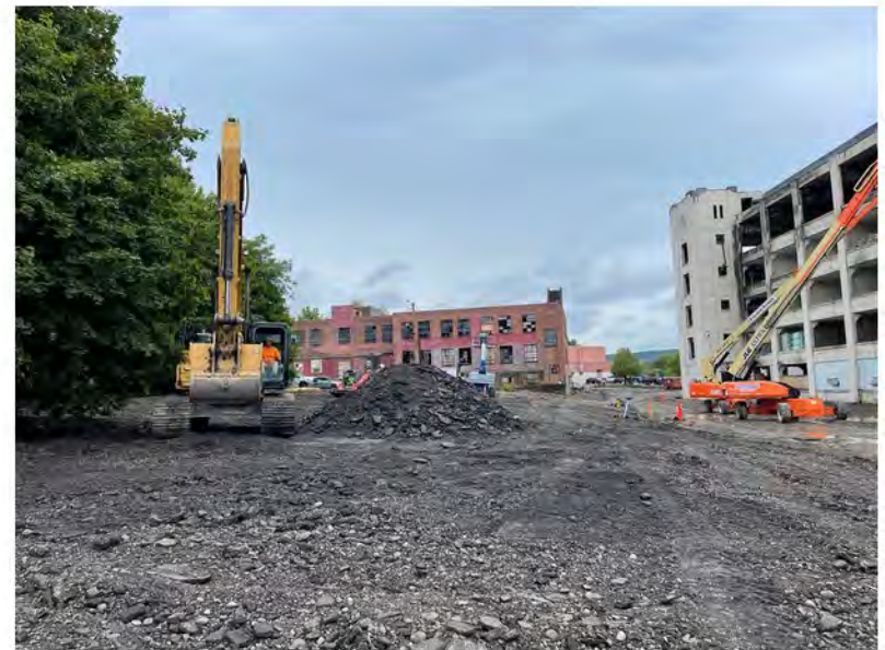
2022-08-22 13:39 42.1153611 N , 75.9520722 W Removal of asphalt in southwestern parking lot (central portion)
