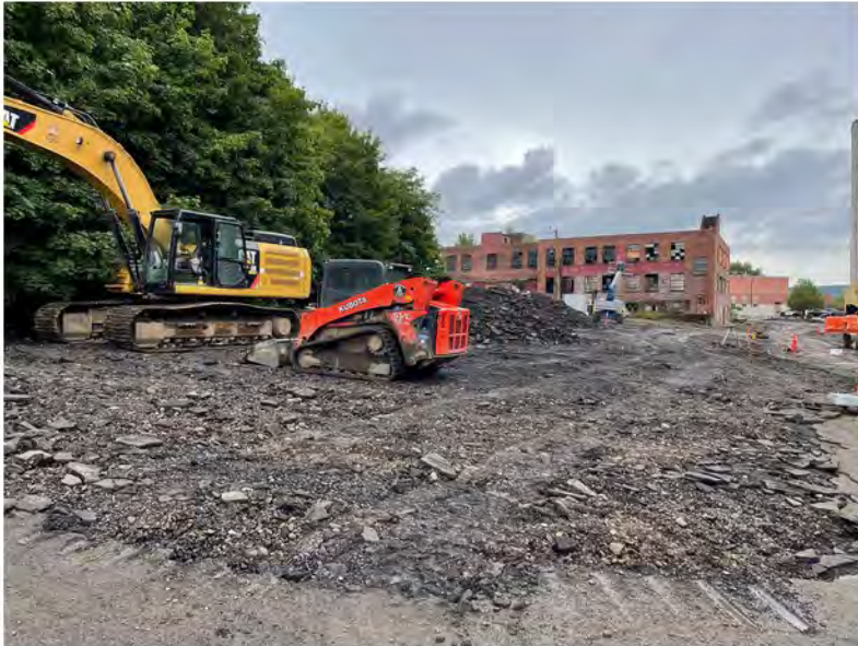
2022-08-22 13:53 42.1154333 N , 75.9520722 W Removal of asphalt in southwestern parking lot (eastern portion)
