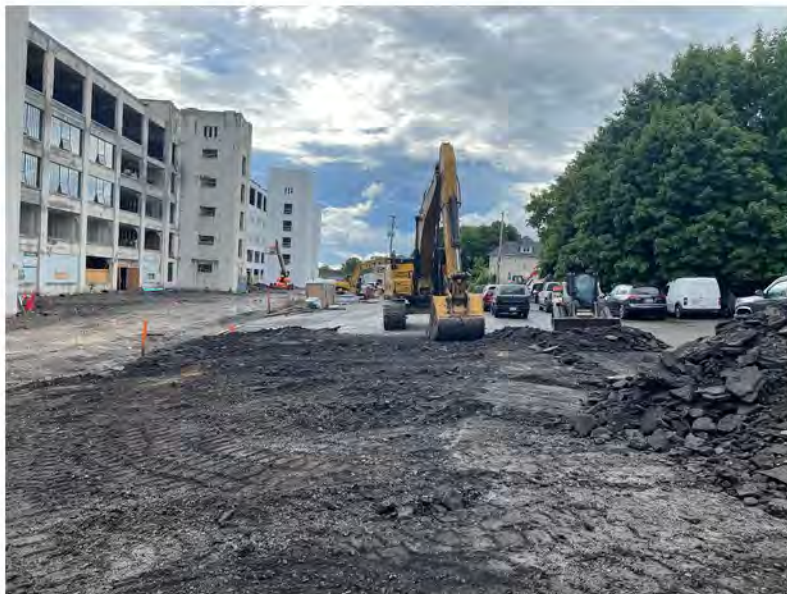
2022-08-22 09:15 42.1156917 N , 75.9527583 W Removal of asphalt in southwestern parking lot (north-central portion)
