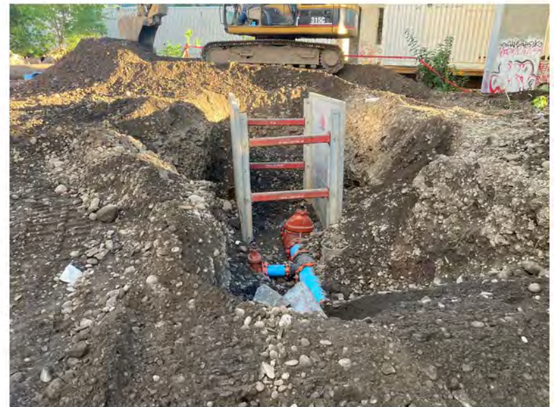
2022-09-02 07:23 42.1155556 N , 75.9504917 W Installation of water line at east end of site
