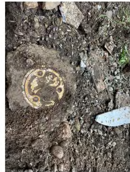
2022-09-08 11:51 42.1147472 N , 75.9515222 W Monitoring well near water line excavation by eastern end of building. Curb box temporarily removed but well riser was not disturbed.
