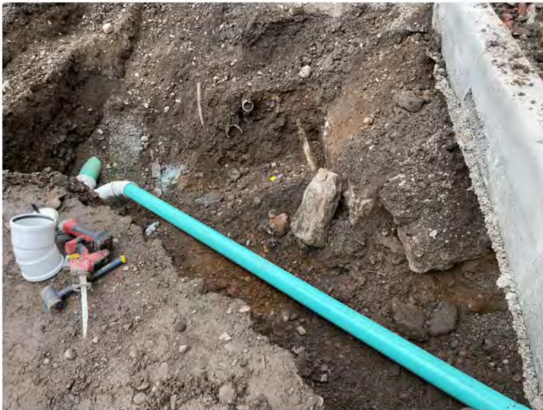
2022-09-08 11:52 42.1152722 N , 75.9507139 W Installation of water line near eastern end of building
