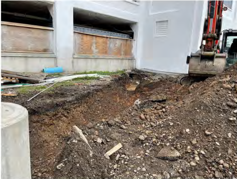
2022-09-08 11:52 42.1152444 N , 75.9507222 W Water line excavation by eastern end of building.
