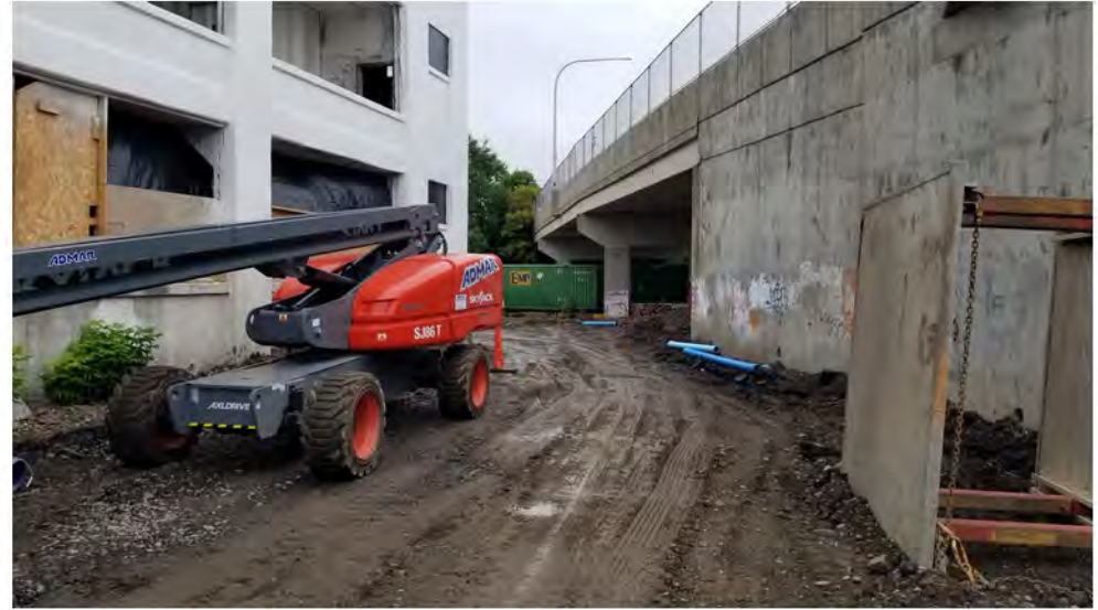
2022-09-13 09:29 42.1151808 N , 75.9503672 W Eastern portion of Avenue C, looking north.
