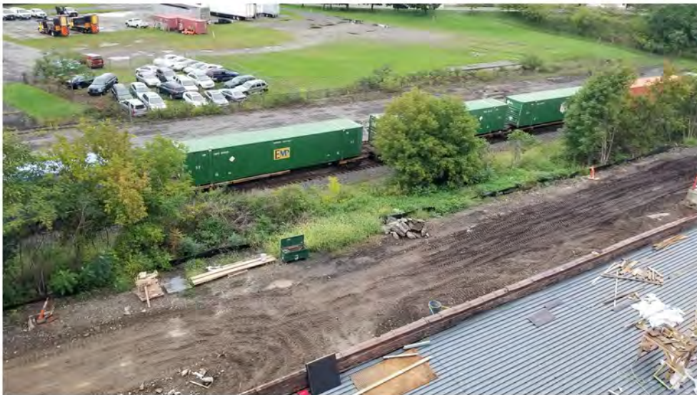
2022-09-13 09:42 42.1155774 N , 75.9525682 W Aerial view of west-central portion of Avenue C, looking northeast.
