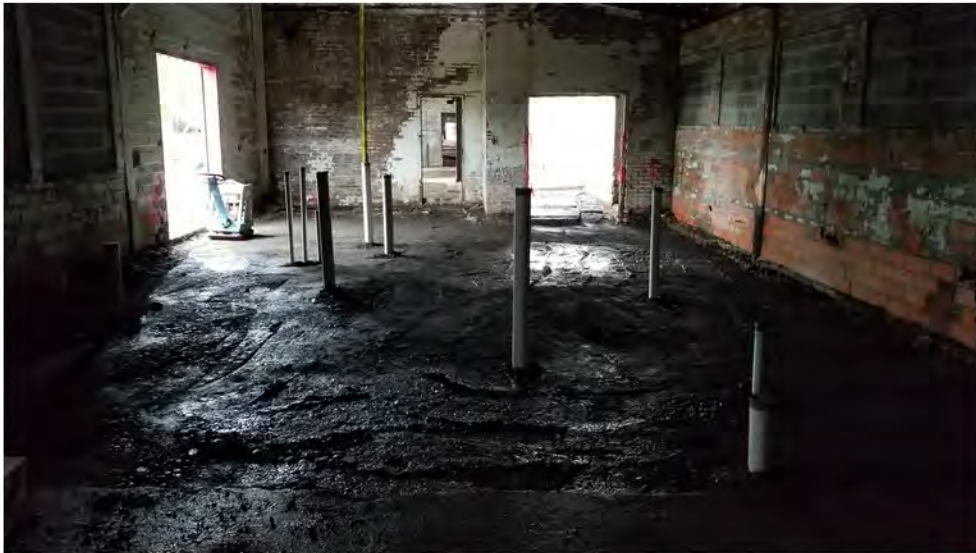
2022-09-13 09:35 42.1162279 N , 75.9494084 W Interior of annex after placement of plumbing.
