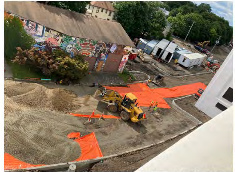
2022-09-14 13:15 42.1152528 N , 75.9509417 W Aerial view of placement of demarcation barrier along eastern portion of Helen Drive.
