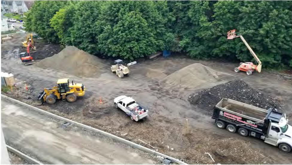
2022-09-13 09:41 42.1152857 N , 75.9524684 W Aerial view of southwestern parking lot, looking southeast.
