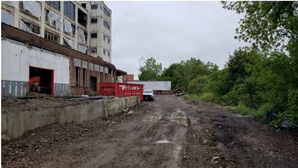
2022-09-13 09:32 42.1160307 N , 75.9540288 W West-central portion of Avenue C, looking west.
