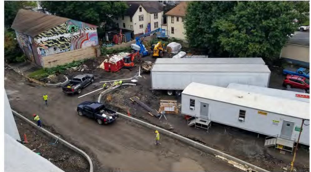
2022-09-13 09:44 42.1149301 N , 75.9517343 W Aerial view of southeastern parking lot, looking southeast.
