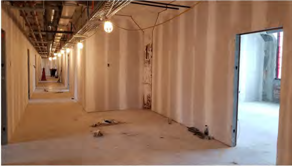
2022-09-13 09:47 42.1046889 N , 75.9370701 W Typical status of interior renovations (for info only).
