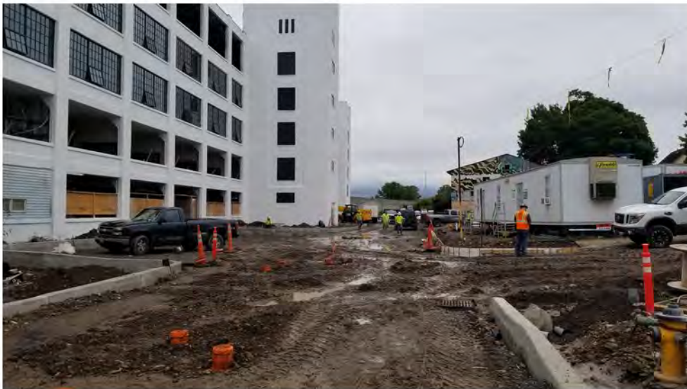
2022-09-13 09:25 42.1154510 N , 75.9521885 W Helen Drive near intersection with Avenue A, looking east.
