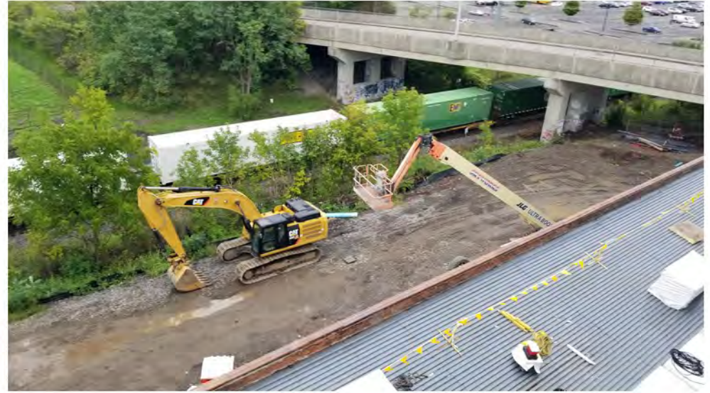
2022-09-13 09:45 42.1148847 N , 75.9516073 W Aerial view of northeastern portion of site, looking northeast.
