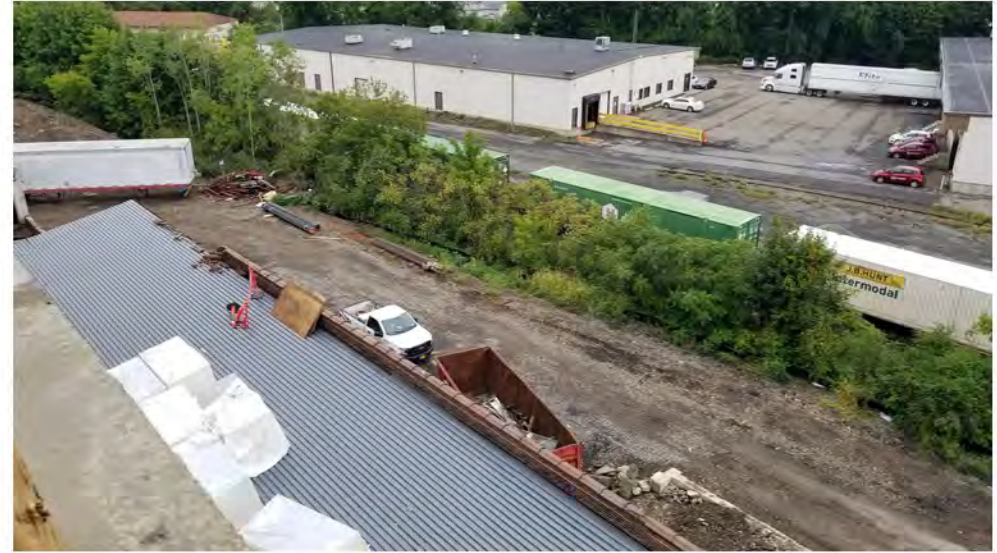
2022-09-13 09:42 42.1155774 N , 75.9525682 W Aerial view of western portion of Avenue C, looking northwest.
