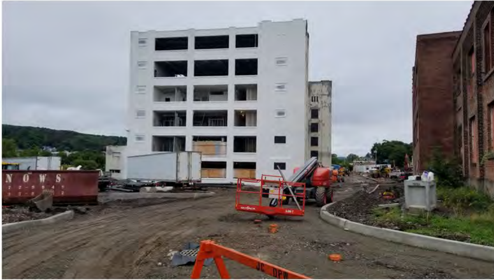
2022-09-13 09:15 42.1158331 N , 75.9540661 W West end of site, looking east.
