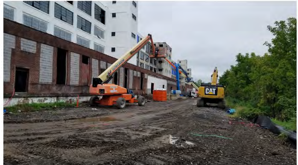
2022-09-13 09:30 42.1160472 N , 75.9479569 W Eastern end of Avenue C, looking west.
