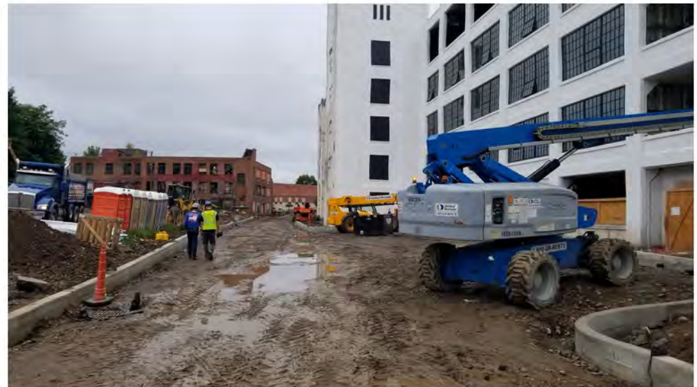
2022-09-13 09:25 42.1153123 N , 75.9516094 W Helen Drive near intersection with Avenue A, looking west.
