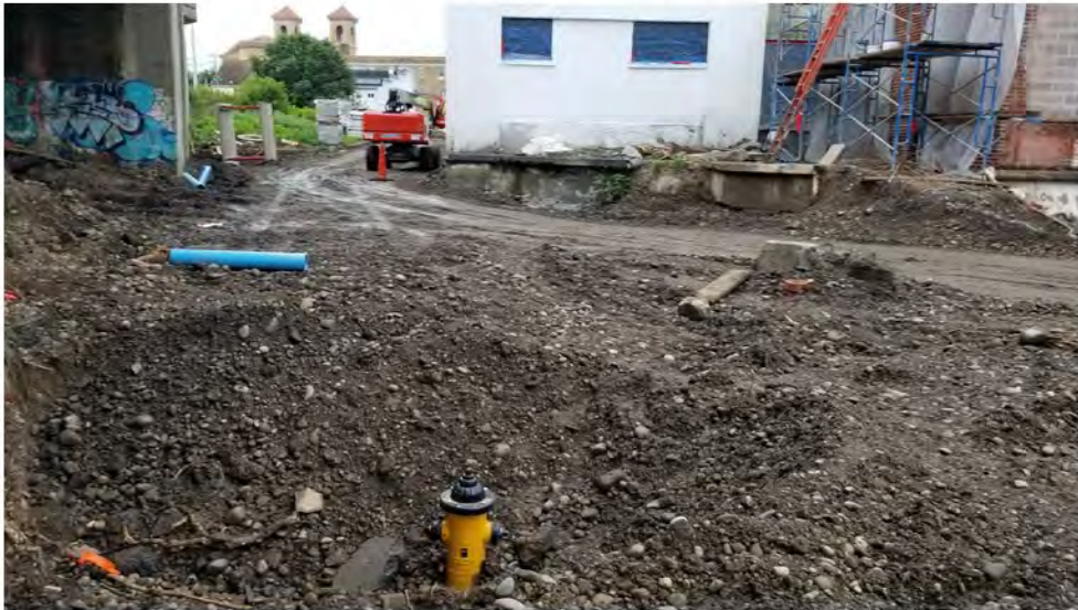
2022-09-13 09:29 42.1160472 N , 75.9479569 W Northeastern corner of site, looking east.
