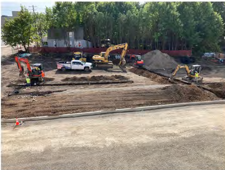
2022-09-21 14:24 42.1154639 N , 75.9519722 W Excavation associated with installation of electrical conduit and drainage lines in eastern portion of southwestern parking lot, looking south
