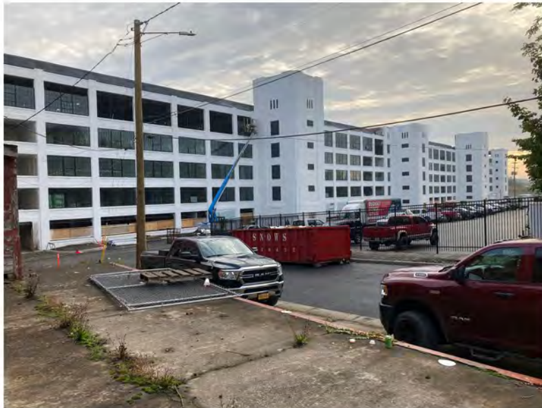
2022-10-07 08:19 42.1153972 N , 75.9531333 W Status of site work, Avenue B looking northeast
