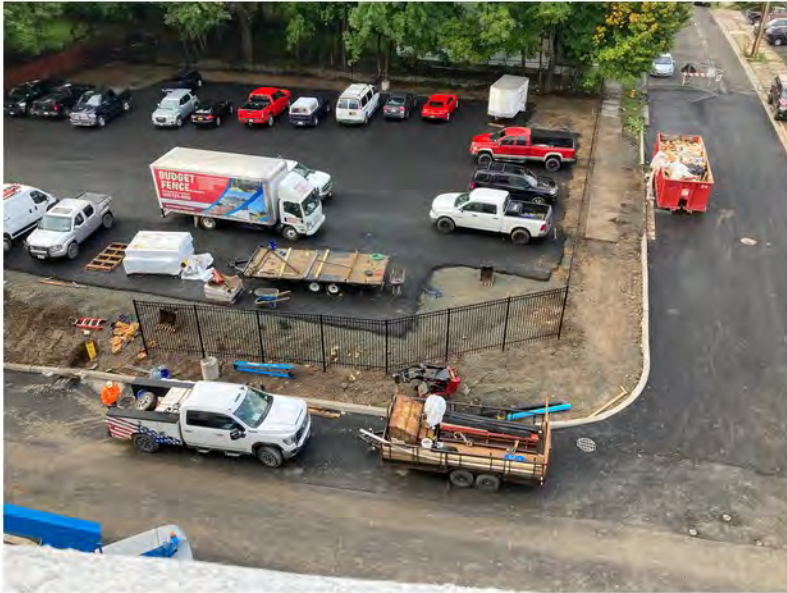
2022-10-07 08:44 42.1156583 N , 75.9528111 W Aerial view of western portion of southwestern parking lot and Avenue B, looking south
