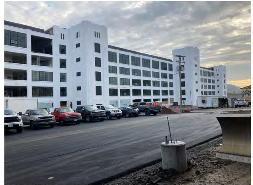
2022-10-07 08:21 42.1156722 N , 75.9520639 W Status of site work, southwestern parking lot looking northeast
