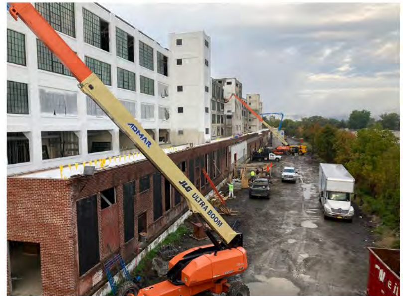
2022-10-07 08:25 42.1155889 N , 75.9503250 W Status of site work, Avenue C looking west
