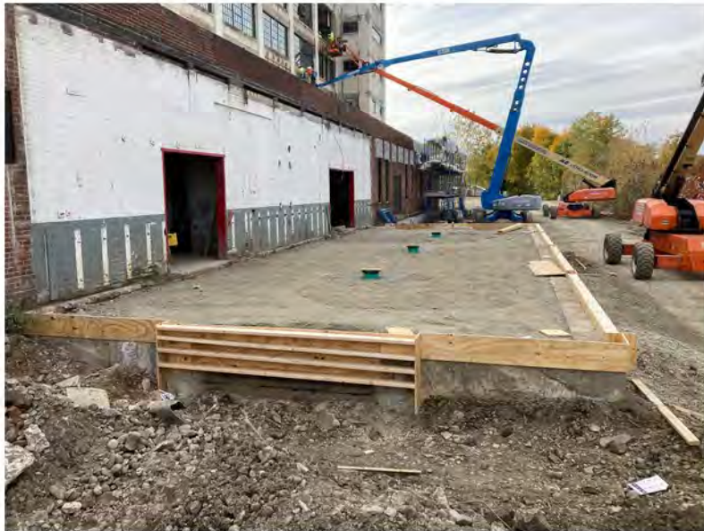
2022-10-20 15:25 42.1157194 N , 75.9520556 W Installation of loading dock off Annex Building, looking west.
