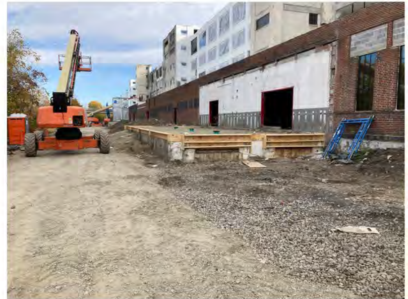
2022-10-20 15:26 42.1160722 N , 75.9525528 W Status of site work along Avenue C, looking east.
