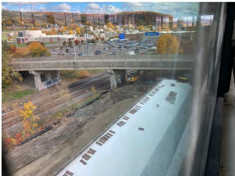
2022-10-25 13:09 42.1154333 N , 75.9509278 W Aerial view of eastern portion of Avenue C, looking northeast
