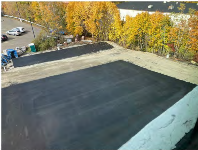
2022-10-25 13:00 42.1157722 N , 75.9528667 W Aerial view of western end of site, looking northwest
