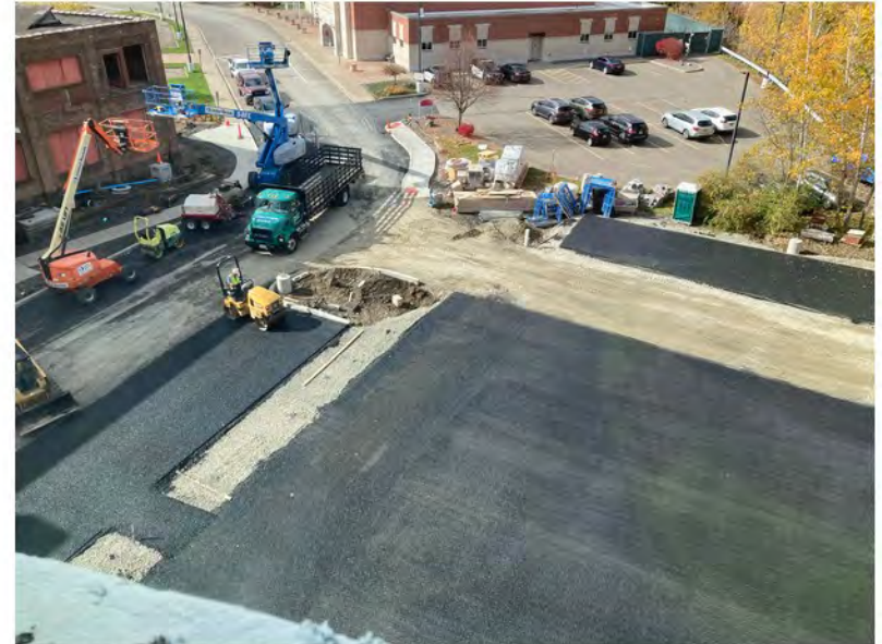
2022-10-25 13:00 42.1157694 N , 75.9531333 W Aerial view of western end of site, looking west
