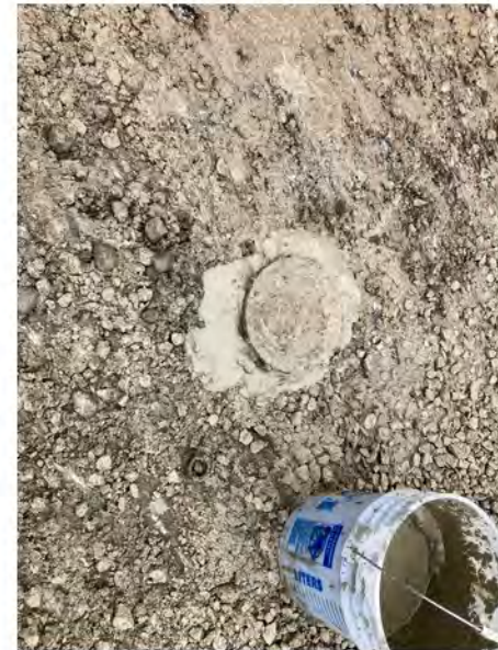
2022-10-24 10:47 42.1160472 N , 75.9527972 W Typical decommissioning of well
