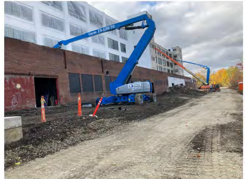
2022-10-25 13:30 42.1158917 N , 75.9516056 W Avenue C and Annex Building, looking west
