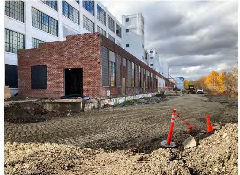
2022-10-25 13:28 42.1156000 N , 75.9503556 W Avenue C and Annex Building, looking west
