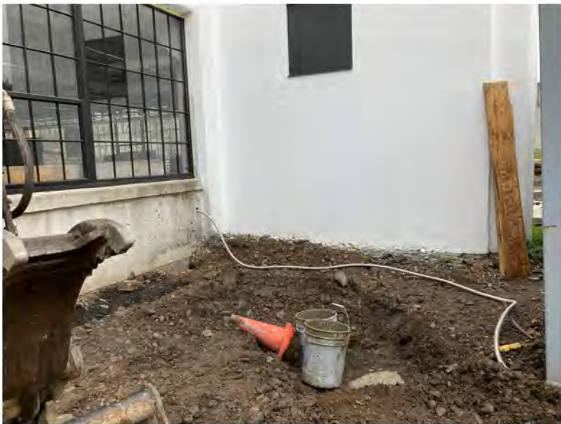
2022-10-24 11:50 42.1151806 N , 75.9507306 W Typical decommissioning of well
