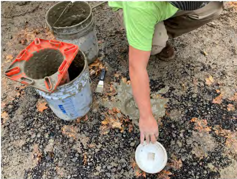
2022-10-24 10:14 42.1152389 N , 75.9520028 W Typical decommissioning of well
