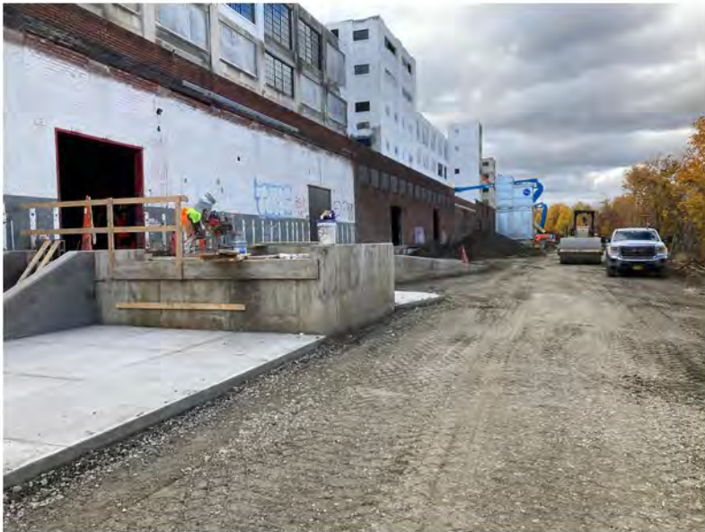
2022-10-25 13:29 42.1156889 N , 75.9508889 W Avenue C, looking west
