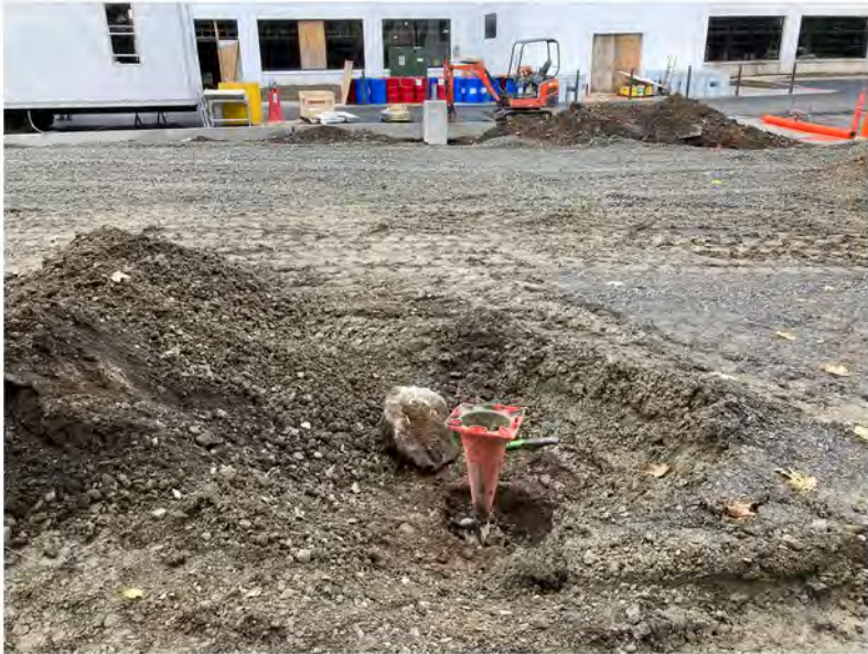
2022-10-24 11:03 42.1151083 N , 75.9513944 W Typical decommissioning of well
