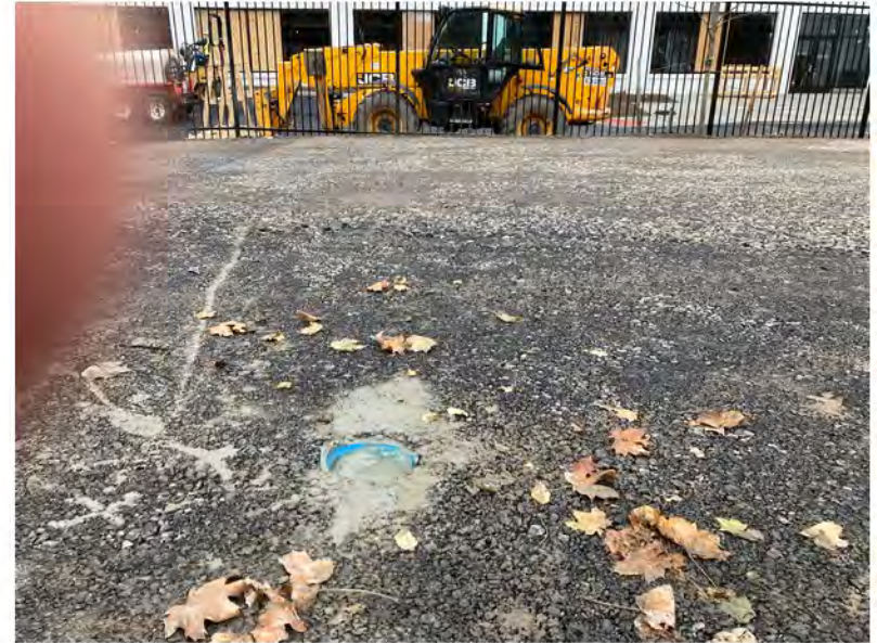
2022-10-24 11:11 42.1155611 N , 75.9527278 W Typical decommissioning of well
