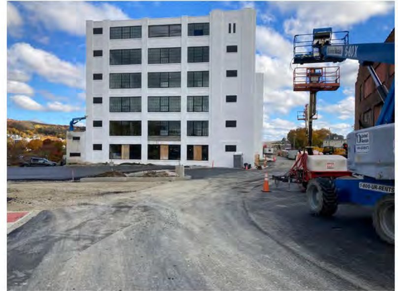
2022-10-25 13:34 42.1159083 N , 75.9534917 W Western end of Main Building, looking east
