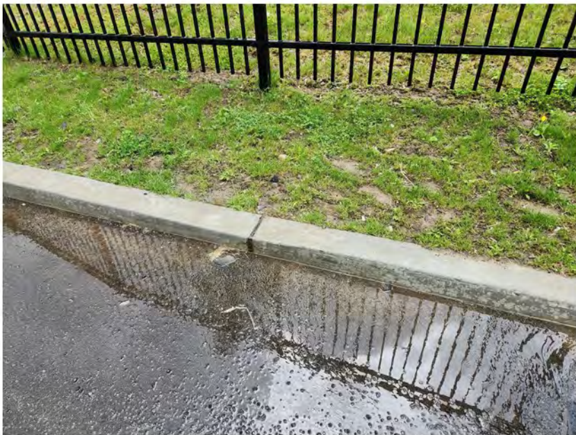
Area of thin lawn area on steep grade, immediately after a downpour. No erosion observed.
