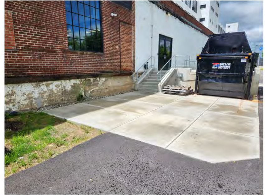
Loading dock area
