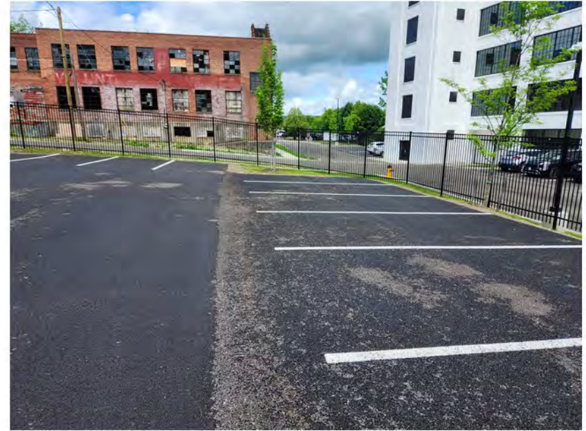
Western end of southwestern parking lot
