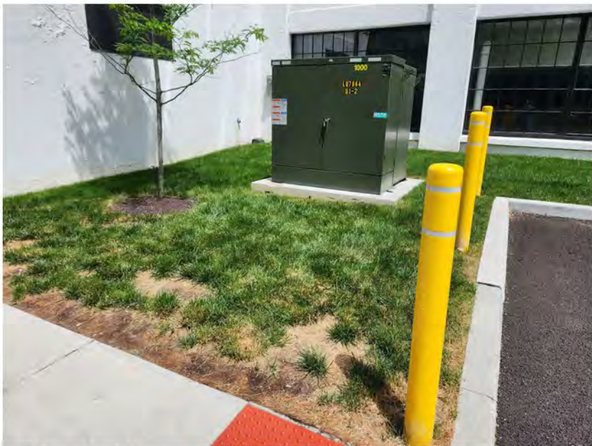
Closeup of lawn area adjacent to parking lot along Helen Drive
