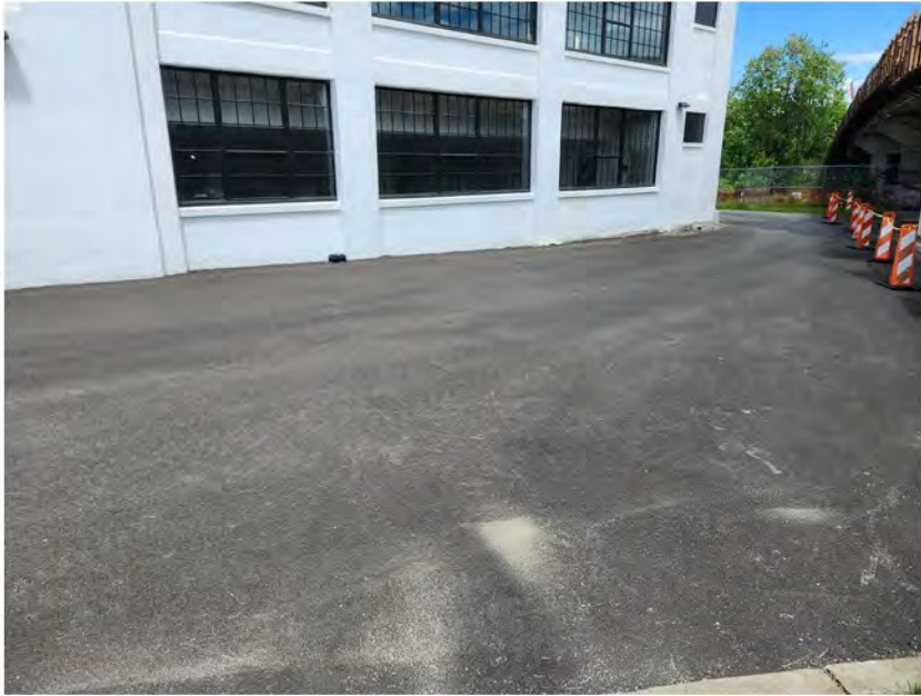
Eastern driveway, looking north
