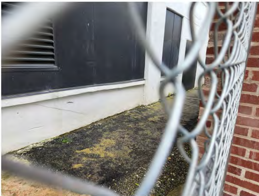
"Courtyard" between main building and annex
