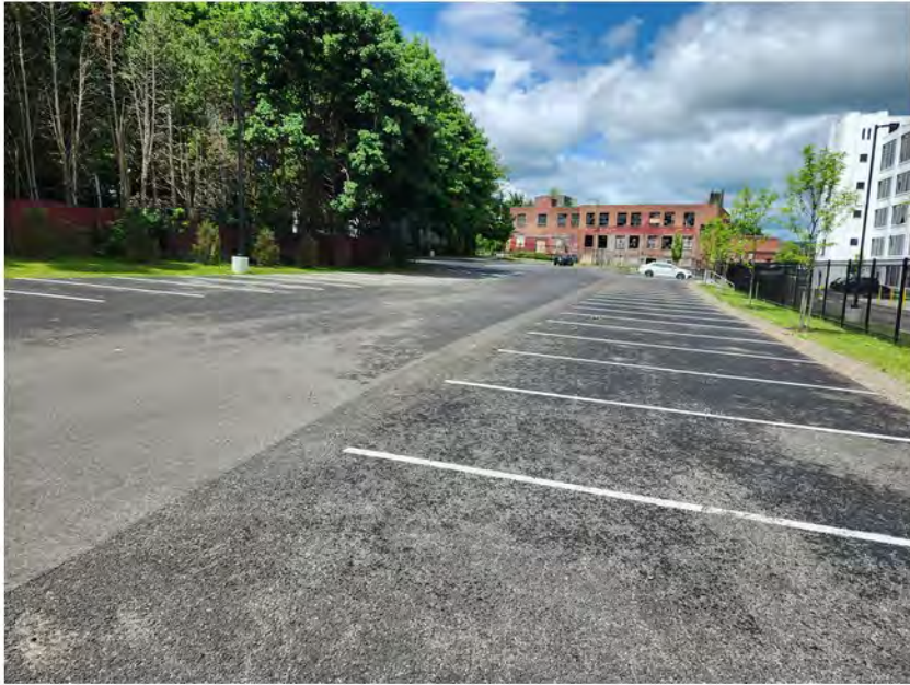
Central and eastern section of southwestern parking lot, looking west
