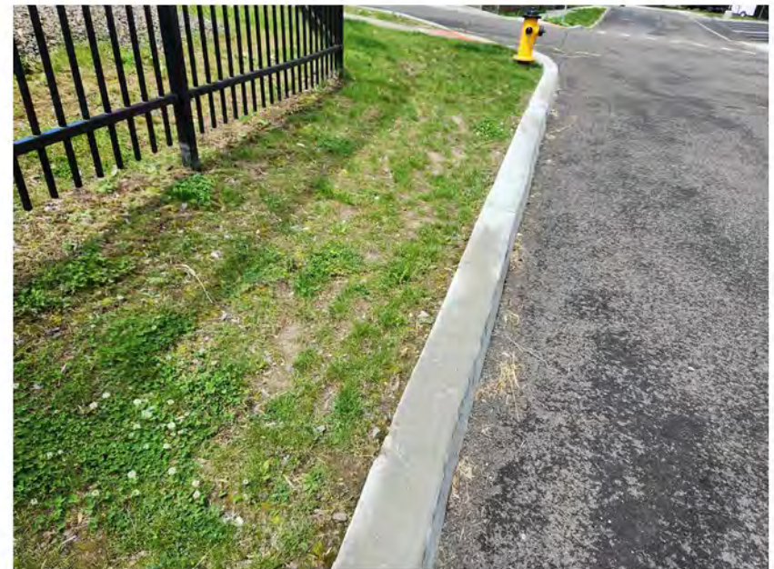
Closeup of lawn at intersection of Helen Drive and Avenue B
