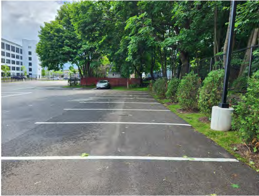
Southern portion of southwestern parking lot, looking east
