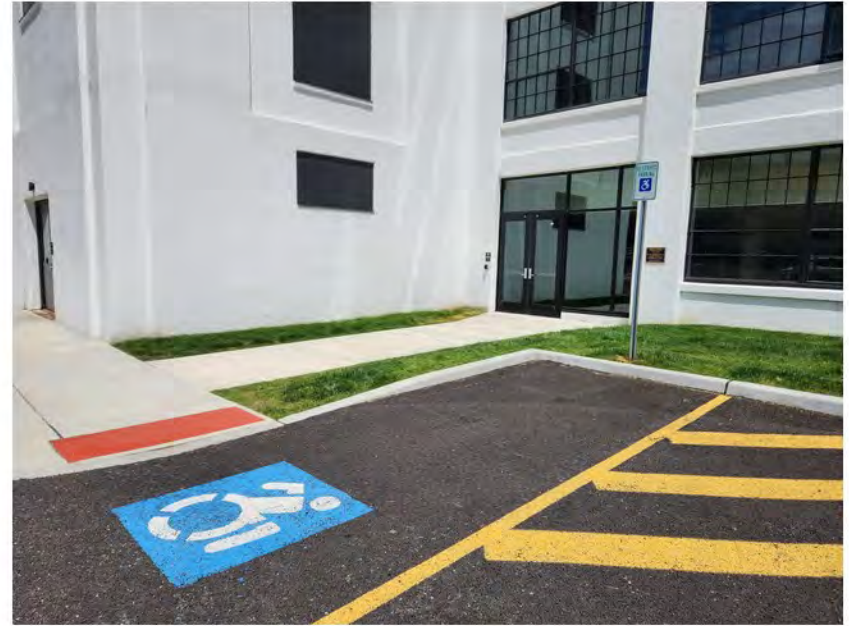
Stairwell entrance along Helen Drive
