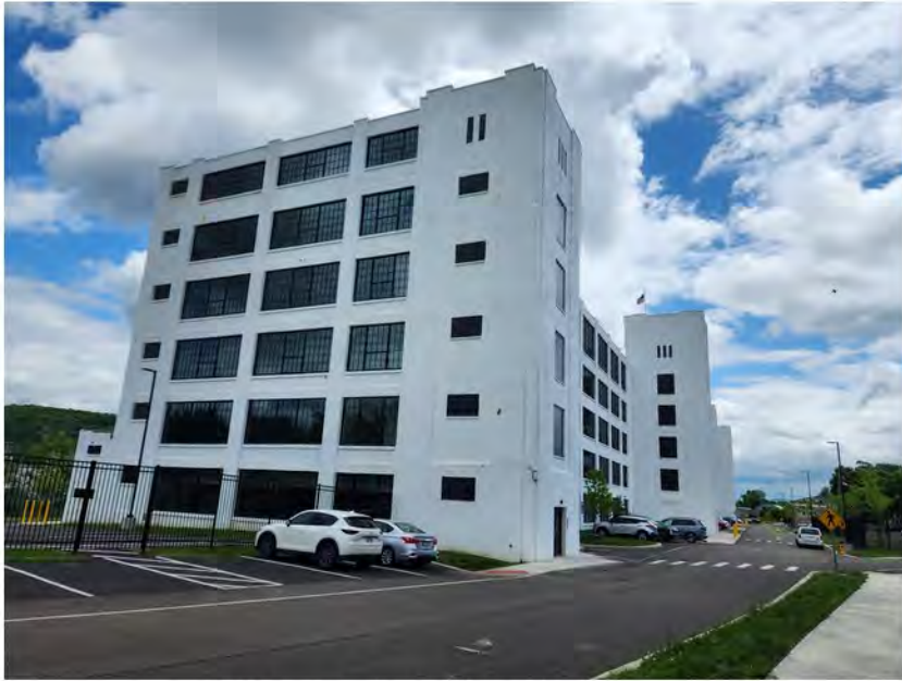
Western end of building, looking east
