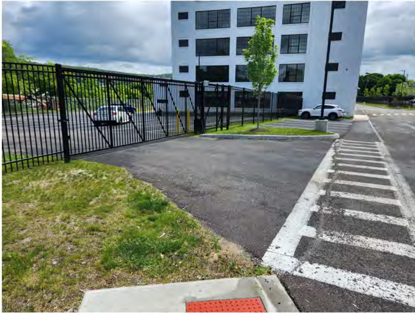
Western end of site, looking east
