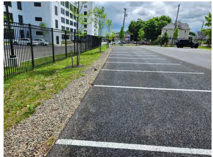
Northern section of southwestern parking lot, looking east
