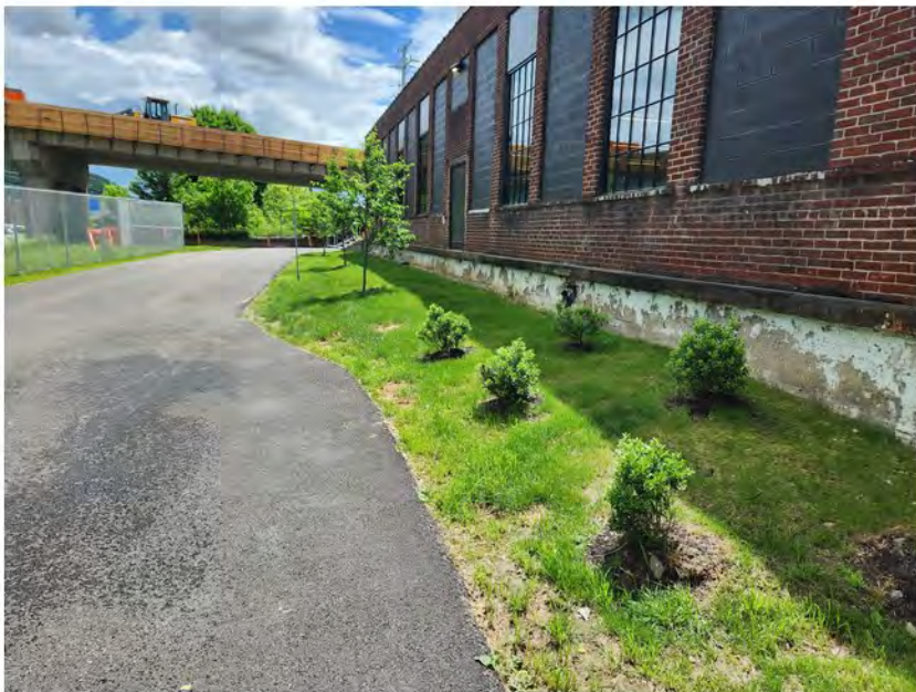
Eastern lawn area along Avenue C, looking east
