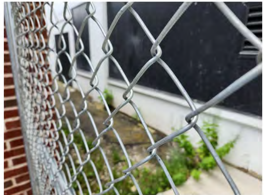
"Courtyard" between main building and annex
