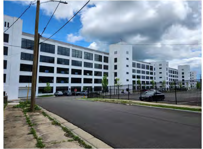
Southern facade of building, looking northeast
