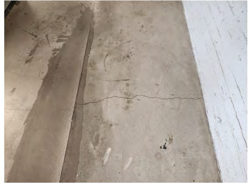
Minor crack in slab
