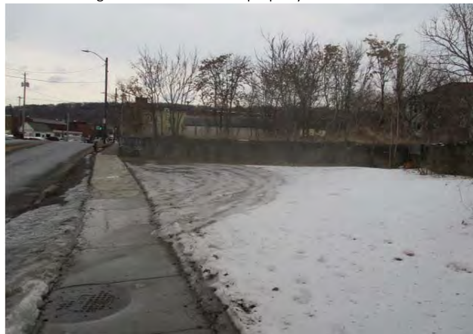
Former loading dock west side of the property
