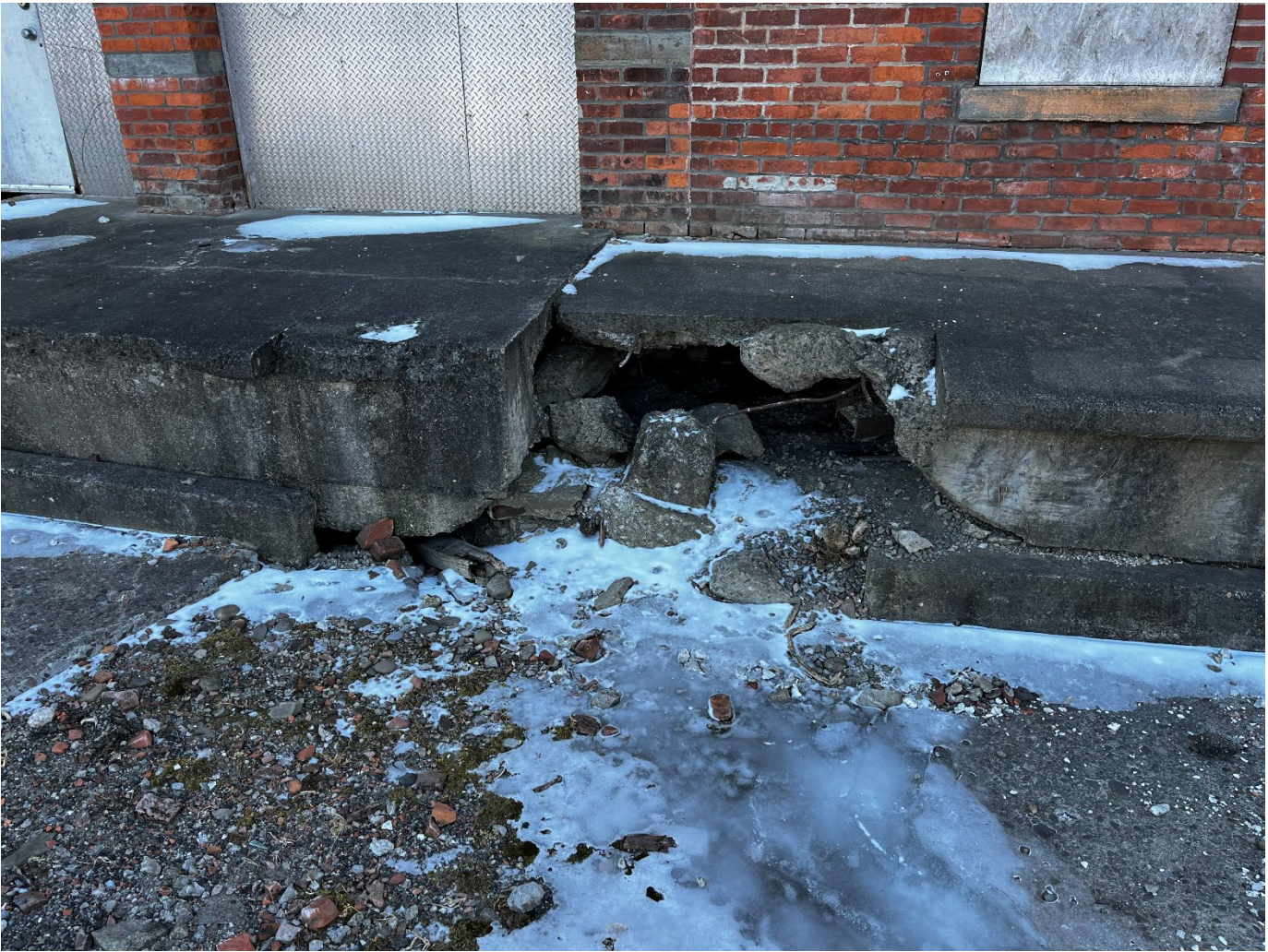
Photo 5 – Broken concrete area
