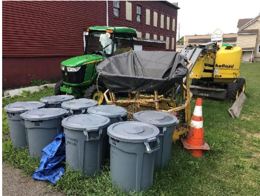
View of the mulch drums, compact tractor, and man lift located at the northeast extent of the Subject Property.
