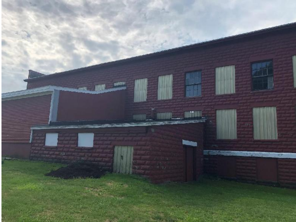
View of the north side of the building facing southeast.
