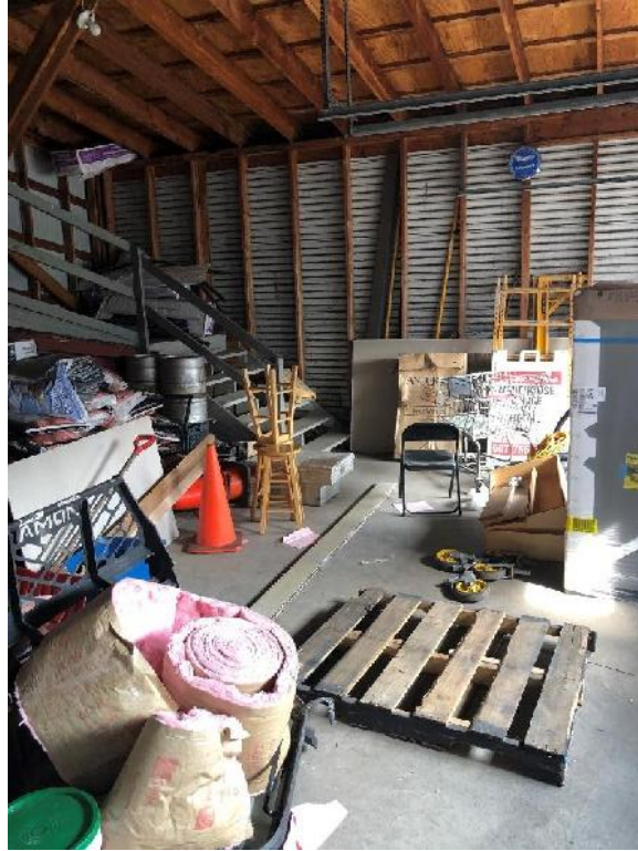
View of the northwest loading dock facing north.
