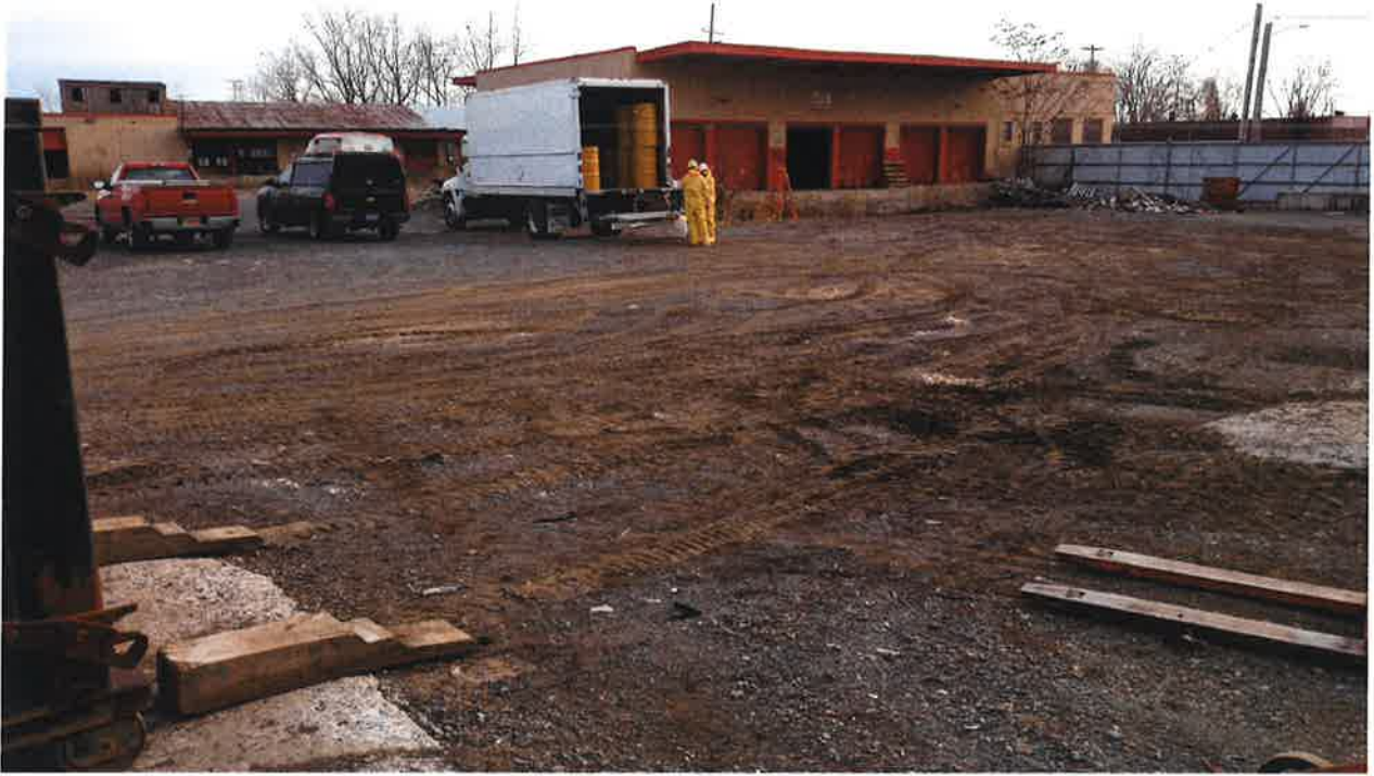
Photo 7 – Building 5 (foreground) & Building 4 (background) – facing North
