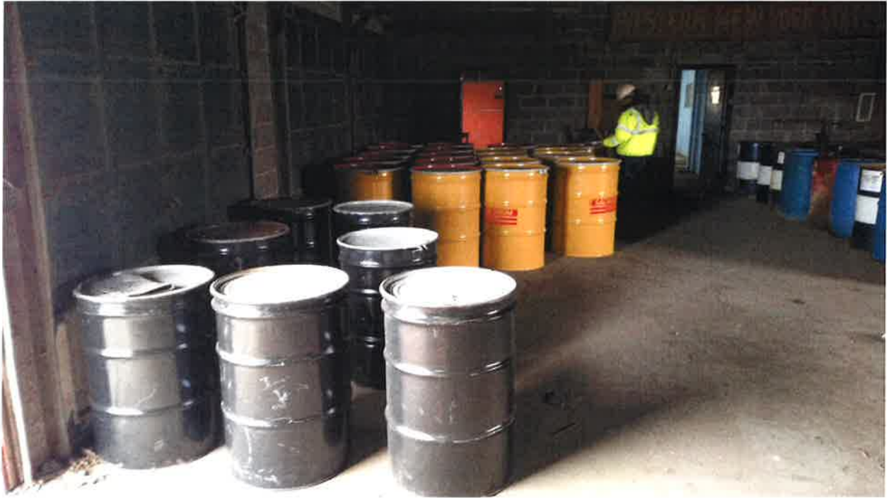
Photo 9 – Building 5 – Nineteen over packed 85 gallon drums (background) and seven 55 gallon water drums (foreground) condensed and housed within building 5
