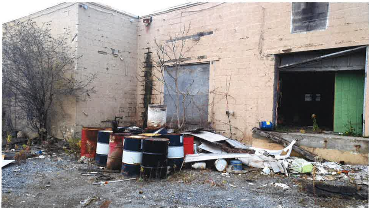
Photo 2 – Yard area near building 6 – Numerous abandoned 55 gallon drums and various debris
