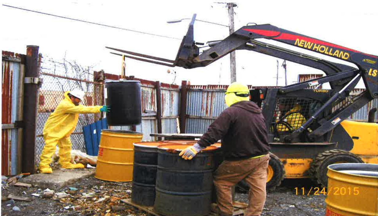
Photo 8 – Yard near building 1 – Over-packing of 55 gallon drum into 85 gallon drum
