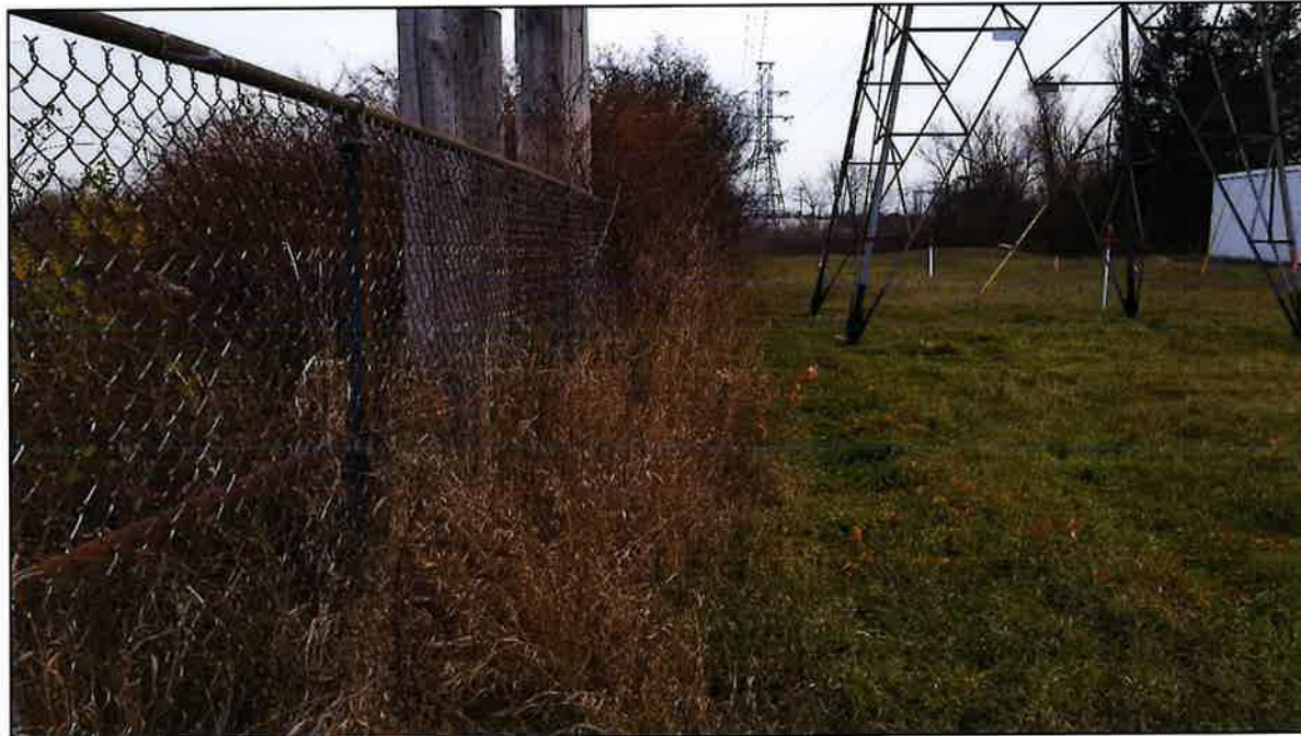
Photo: 52. Facing E at flag “WL A 196” towards PEM in Wetland Complex A (on left) and uplands and electric substation (on right) (photo taken 11/15/2017).
