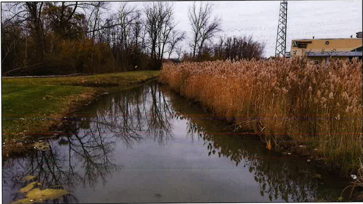
Photo: 9. Facing N at culvert, flag "GPS BENCH 1" towards swale and PEM in Wetland Complex A (on right) (photo taken 11/14/2017).
