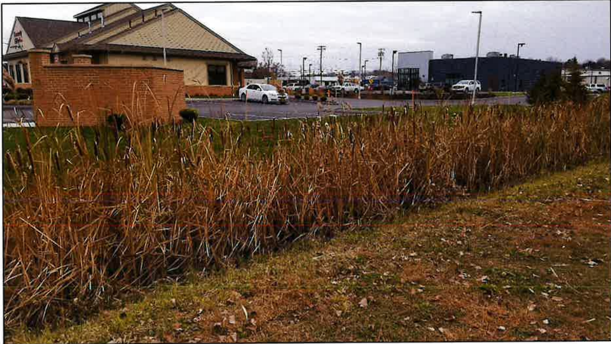
Photo: 3. Facing S at SP-01 towards swale (photo taken 11/14/2017).
