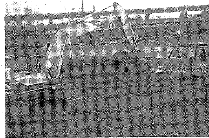
Photograph 12: The gasoline, fuel oil, and waste oil UST cavities were filled with bank run gravel upon completion of remedial excavation activities.
