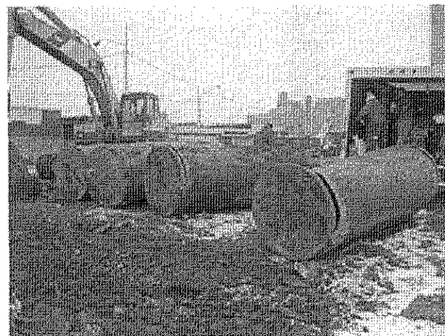
Photograph #2: From left to right, condition of gasoline USTs 1-4 upon removal; (fair/good) Looking northeast.
