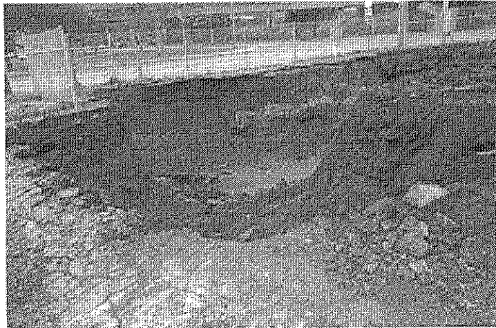
Photograph 9: Extent of remedial excavation at the southern side of the south excavation pit of the gasoline UST field; Looking west-northwest.
