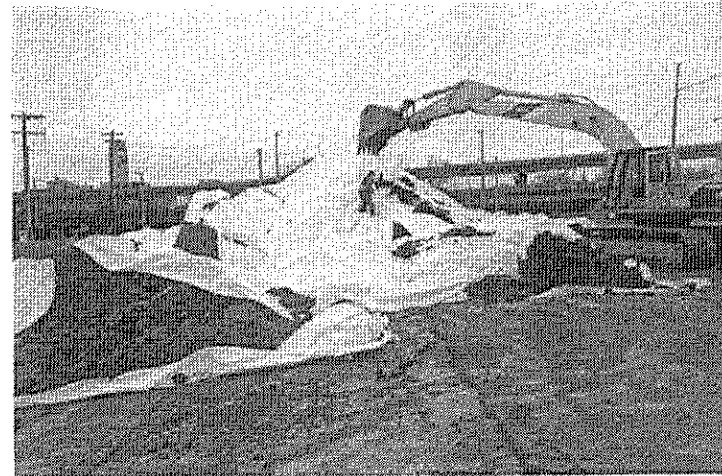
Photograph 10: Petroleum-impacted soil stockpile placed on and covered with polyethylene sheeting.
