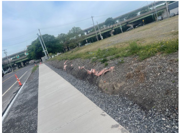
Image of the engineered cap disturbance during sidewalk installation activities.
